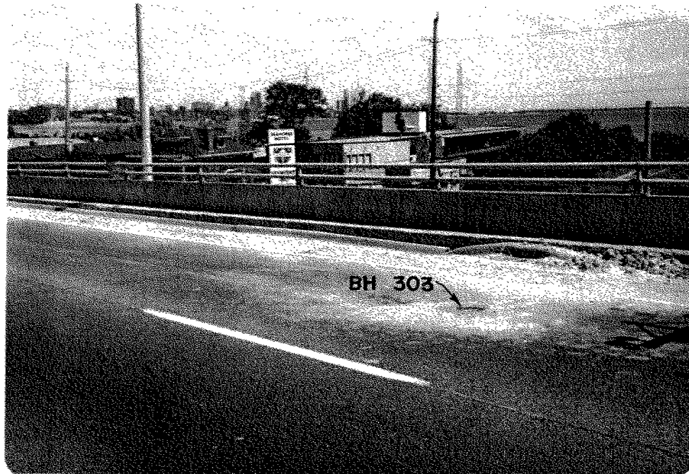
SETTLEMENT OF PAVEMENT SURFACE AND DIFFERENTIAL MOVEMENT WITH RESPECT TO CATCH BASIN.
