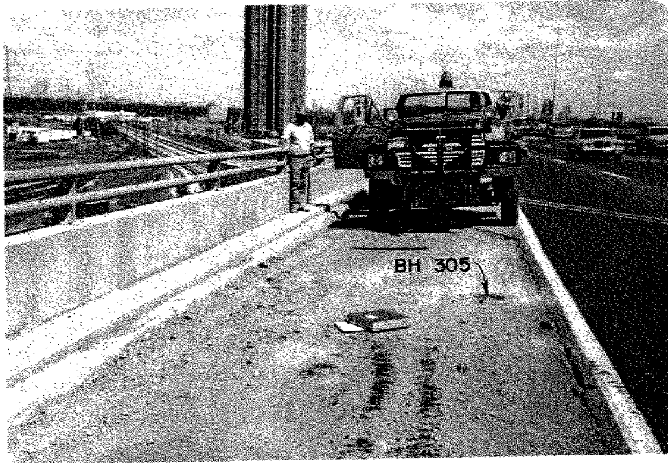
SETTLEMENT OF EMBANKMENT SHOULDER - NOTE SETTLEMENT OF CURB RELATIVE TO PAVEMENT.
