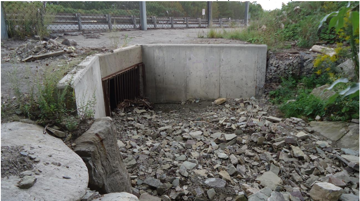
Photograph 4: Looking northeast at the inlet structure and debris accumulation area (September 14, 2016).
