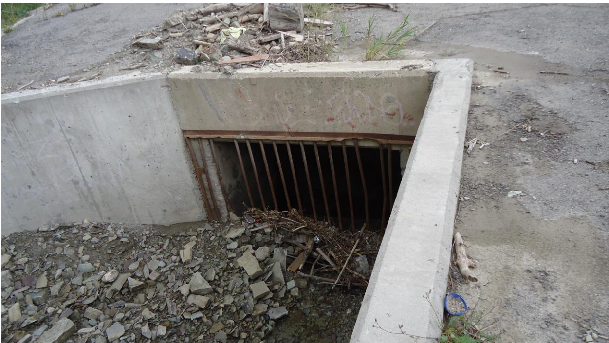
Photograph 6: Looking at the inlet structure and debris accumulated at the rack base (September 14, 2016).
