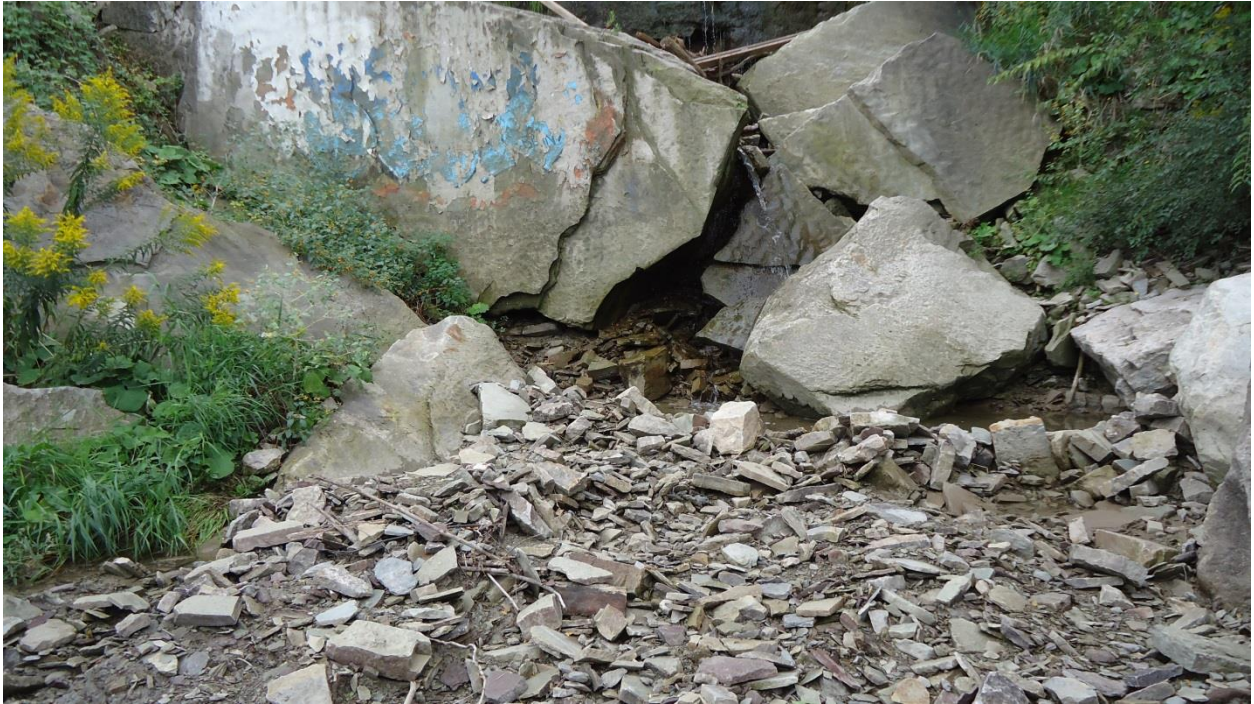
Photograph 3: Looking south at the outfall chamber of Lower Princess Falls; huge boulders, cobbles and debris have accumulated as a result of erosion (September 14, 2016).
