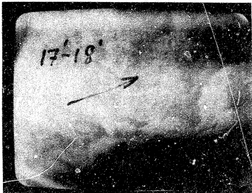
Photograph #13 Caisson 5, El. 234 feet Radial view of void at top of tremied concrete
