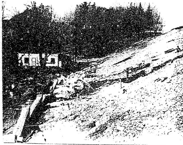
View to north, showing piezometer and slope indicator pipes, as well as wet areas on side slope
