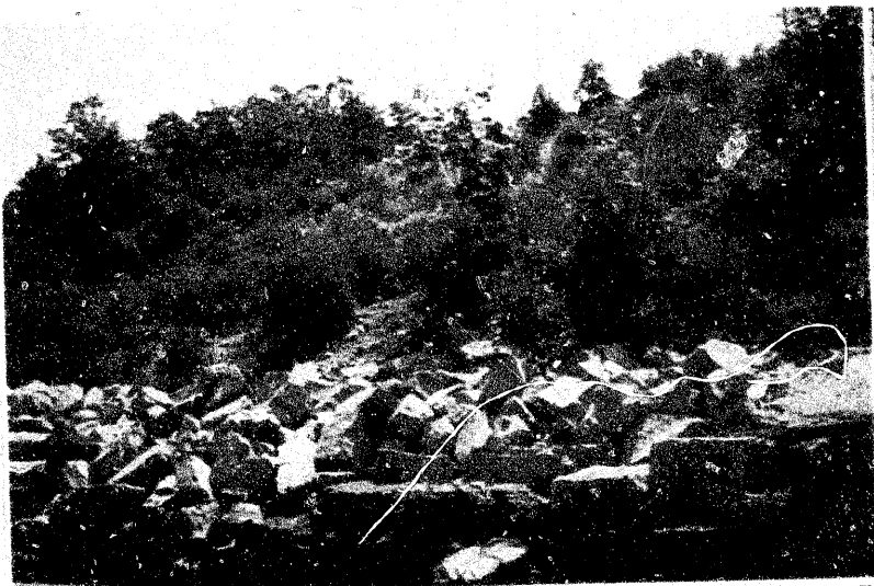
12: S. Wilson's Drive Near Ferguson, outside of J. L. Hamilton Attempt at Arresting Creeping Crawling by Lining Top With Large Rock.
