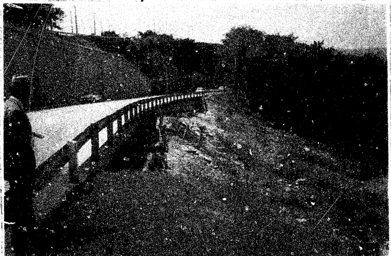
FIG. 24: Flock Road - New Depression Road, Hamilton. Step 1: Failure Prior to Completion of Crest - Shows how Provision of Curbed Curb and Shoulder.
