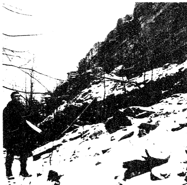
Fig. 8 - Taken in abandoned railway cut showing Clinton Formation at bottom of cut. Note how breakdown and erosion of Rochester Formation has undermined overlying rock causing rock slumps in centre and rock falls at bottom of picture.
