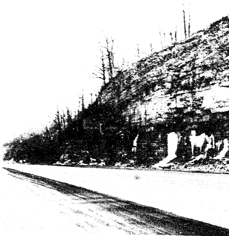
Fig. 24 - Taken in No. 2 highway cut near Ancaster showing how break down of shale by ground water percolation tends to undermine overlying formations.
