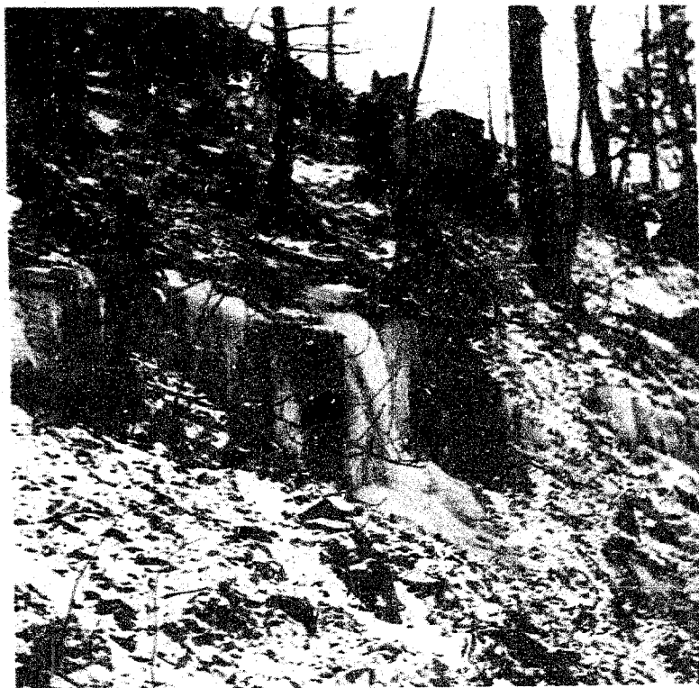
Fig. 23 - Taken at chng. 243+00 - 200' L. looking west showing ground water flowing over Clinton Formation.
