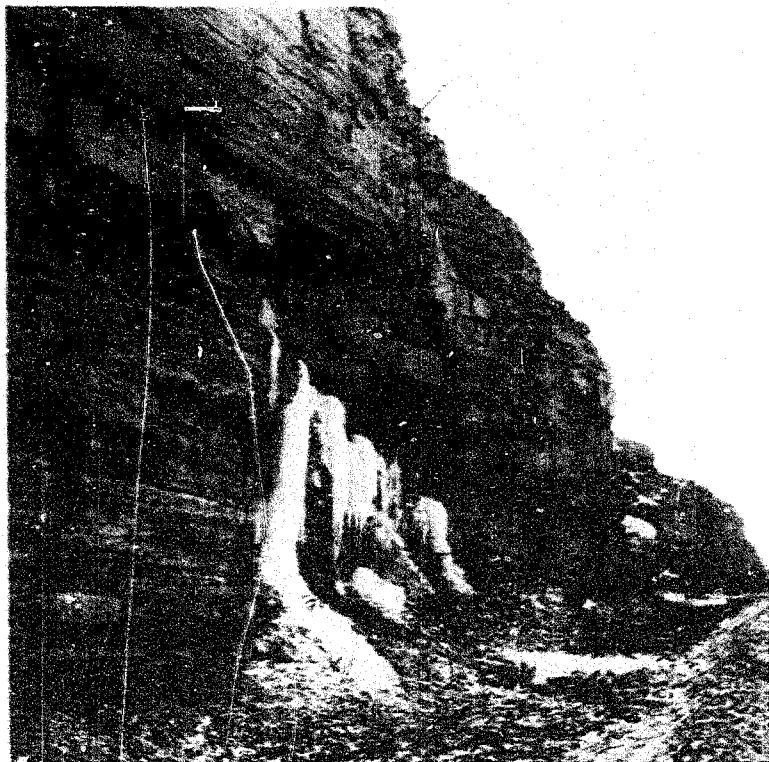
Fig. 25 - Close-up view of fig. 24 showing weak vertical planes in limestone overlying eroded shale. Wedge and splinter shaped particles will soon fall here.
