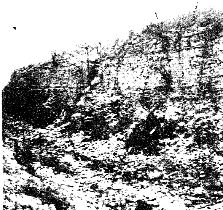
Fig. 6 - Taken in abandoned railway cut showing "Undivided" Lockport and Gasport member. Note tendency of "Undivided" member to break down and form rubble at toe of cut.
