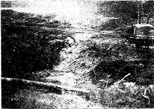
Excavation of organic material for South Service Road.
