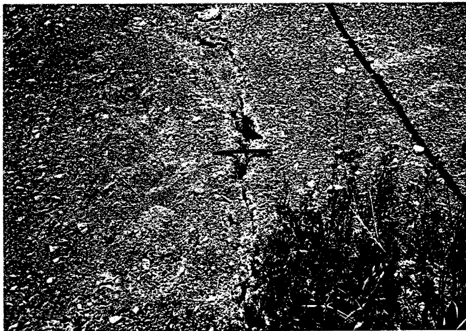
PHOTO #5. CLOSEUP OF LONGITUDINAL CRACKS ON NORTH APPROACH
