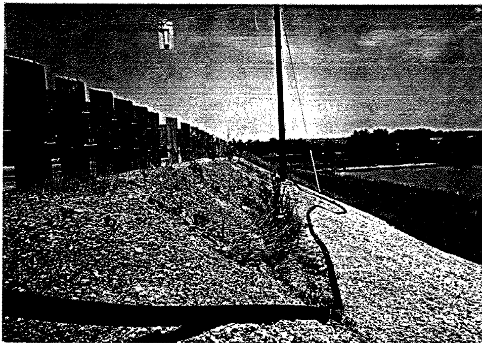
PHOTO #7. SURFICIAL SLOUGHING AT NORTH APPROACH FILL (EAST SIDE, LOOKING NORTH)
