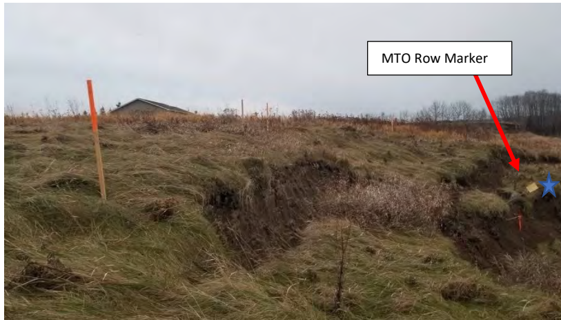
Figure 8: Top of Slope Failure on Friday 13th of Nov 2020 - No Changes from Wednesday 11th of Nov 2020
