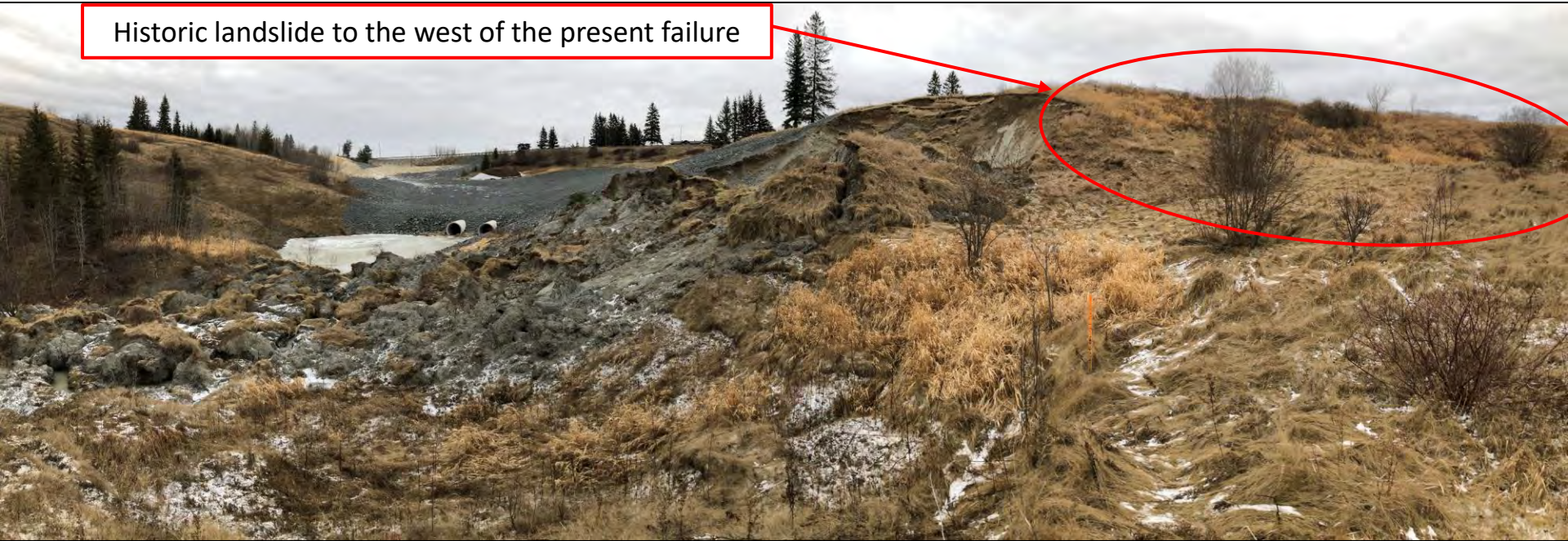
Photo 8: Panoramic view of the landslide, looking northeast to southeast. Bowl-like topography to the west is likely a remnant of a historic landslide.
