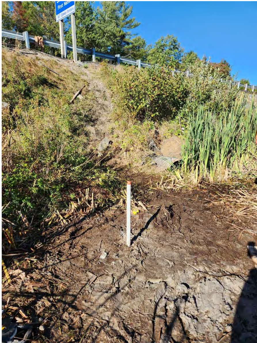
Photograph 6: Borehole 23-10 After Completion
