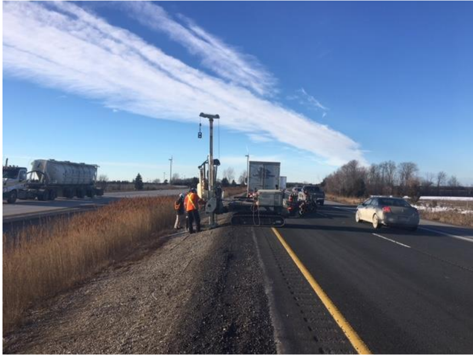
Photo 1. Drilling BH17-20 at Hwy 401, facing west
