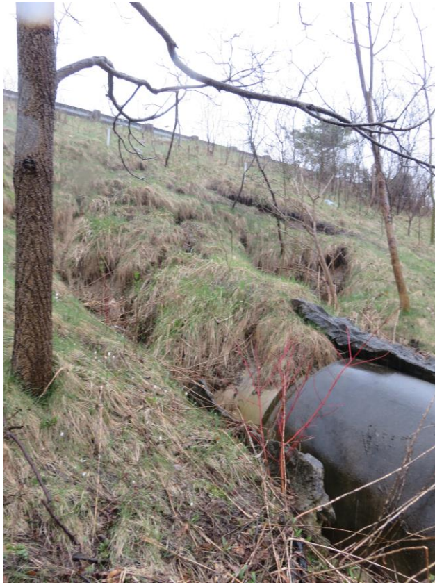
Photo 11: Slope failure above the existing culvert looking west-north from the outlet
