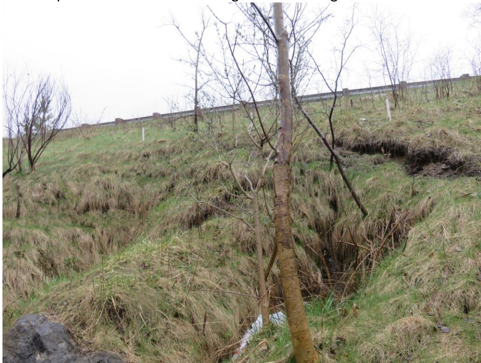
Photo 12: Slope failure above the existing culvert looking west from the outlet
