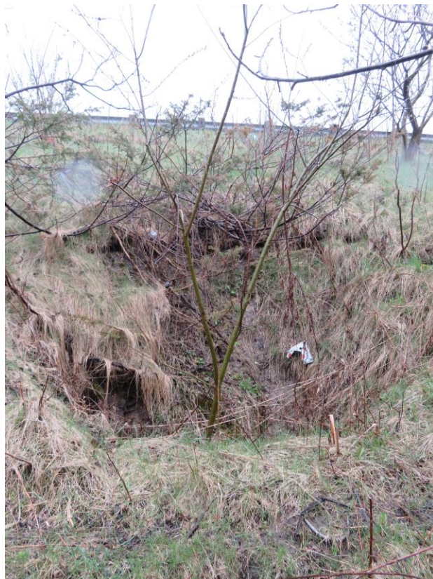
Photo 14: Slope failure above the storm water pipe looking west from the outlet
