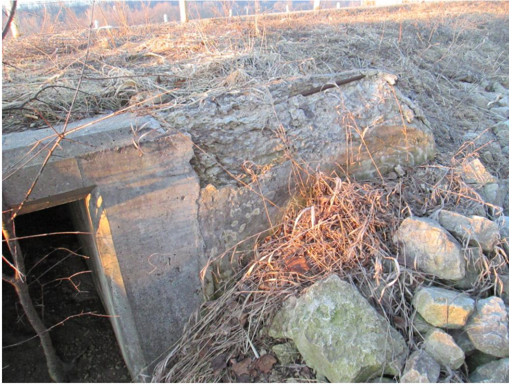
Photo 7: Deterioration of wingwall on outlet side
