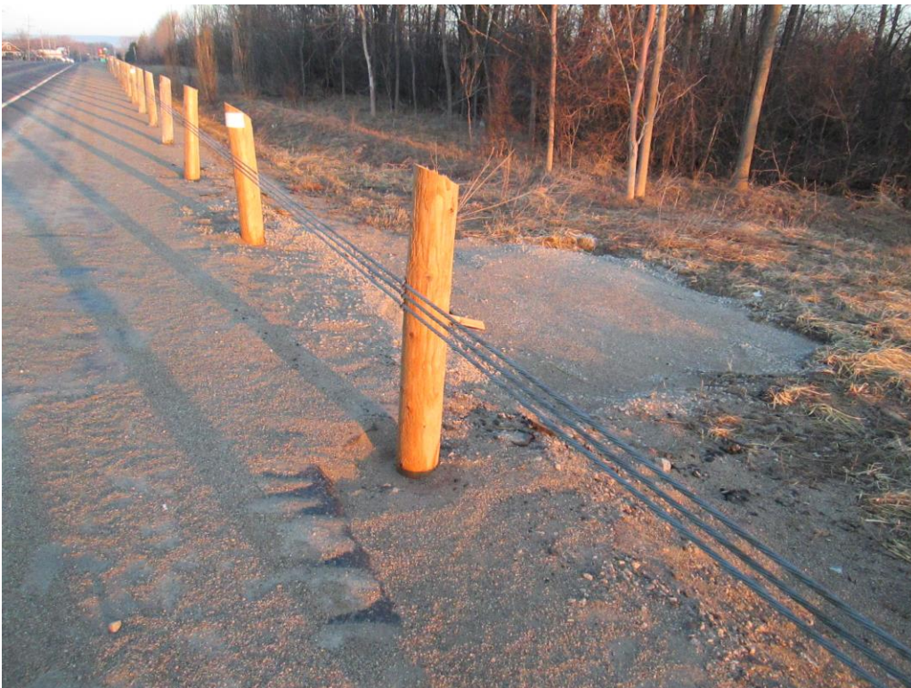
Photo 8: Recent cut and backfill mark on outlet side of the culvert
