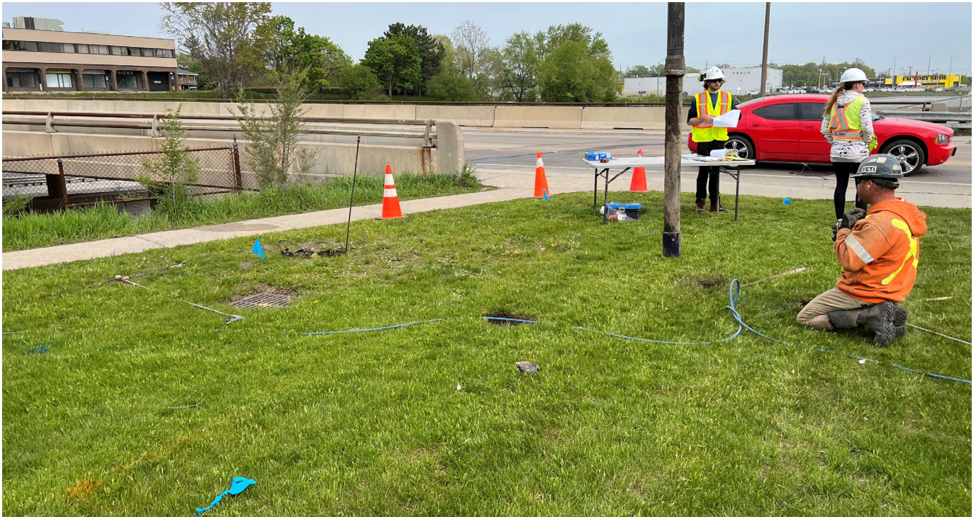
Photograph #6 – Hydroexcavation at Borehole FS23-06, facing north. (May 2023)
