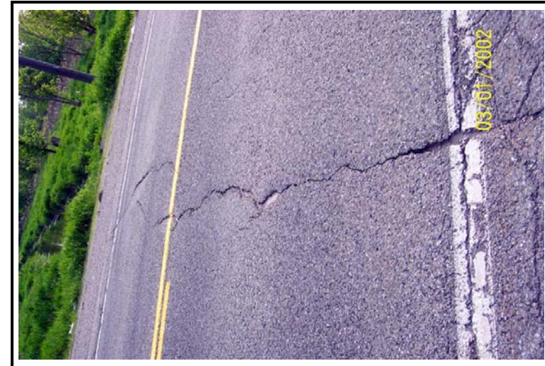
Photo 3 Asphalt Deterioration Along Roadway
