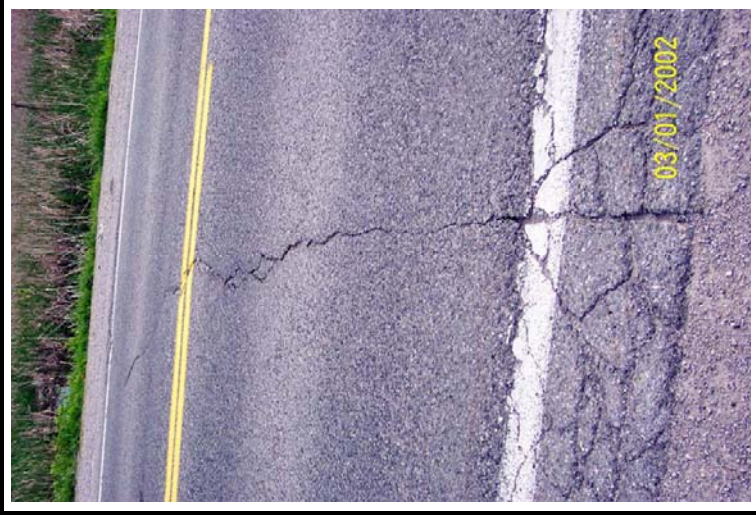
Photo 3 Asphalt Deterioration Along Roadway
