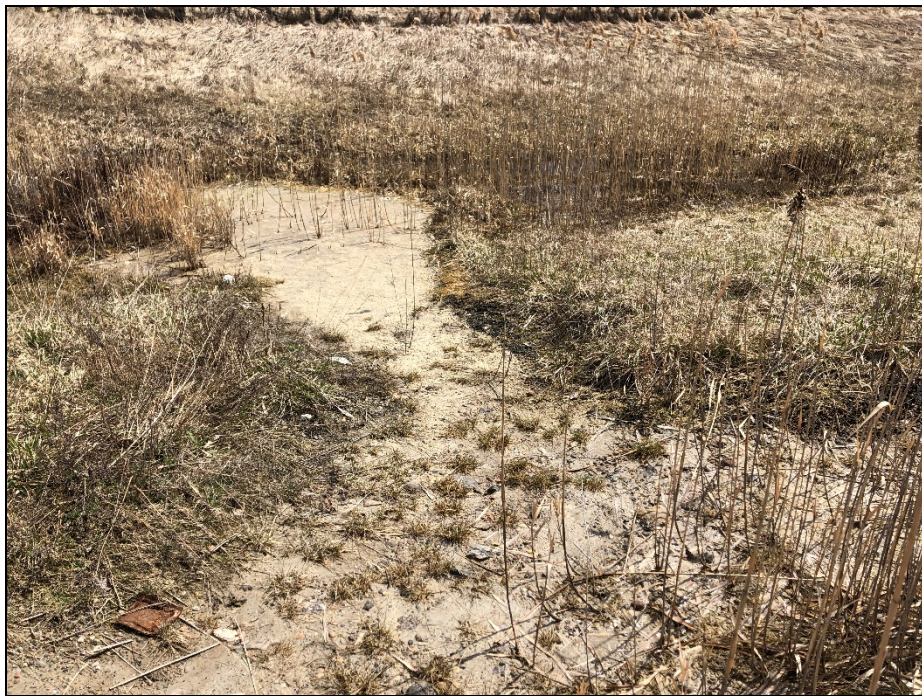
Photos 4 and 5- Existing slope at the S-E/W Ramp, looking towards the slope from top and mid-slope. Localized wet area at the toe of the slope.
