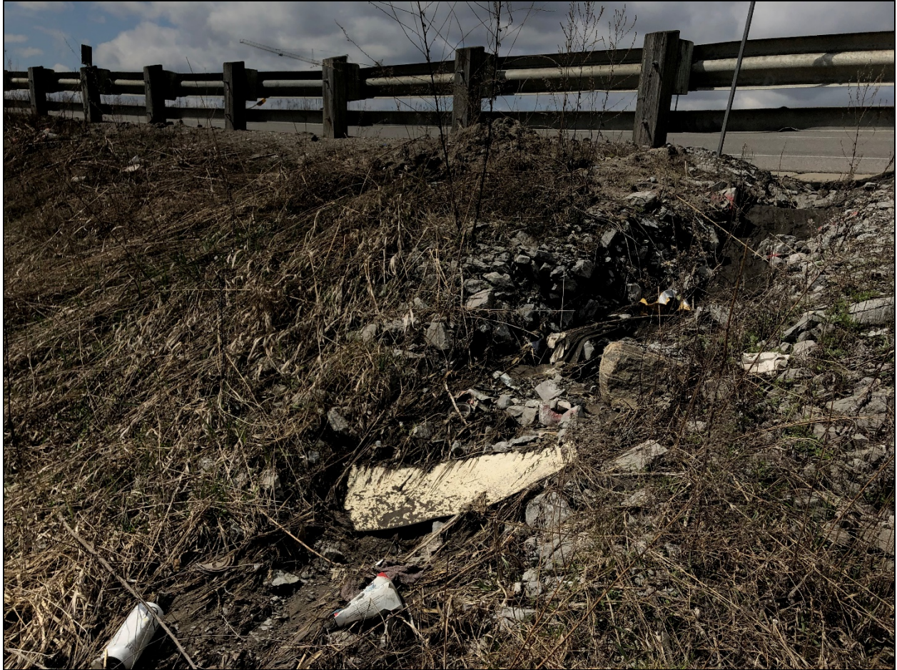
Photo 1- East side of the S-E/W Ramp Modified swale at the of the curb. Fill observed at the top of the slope.
