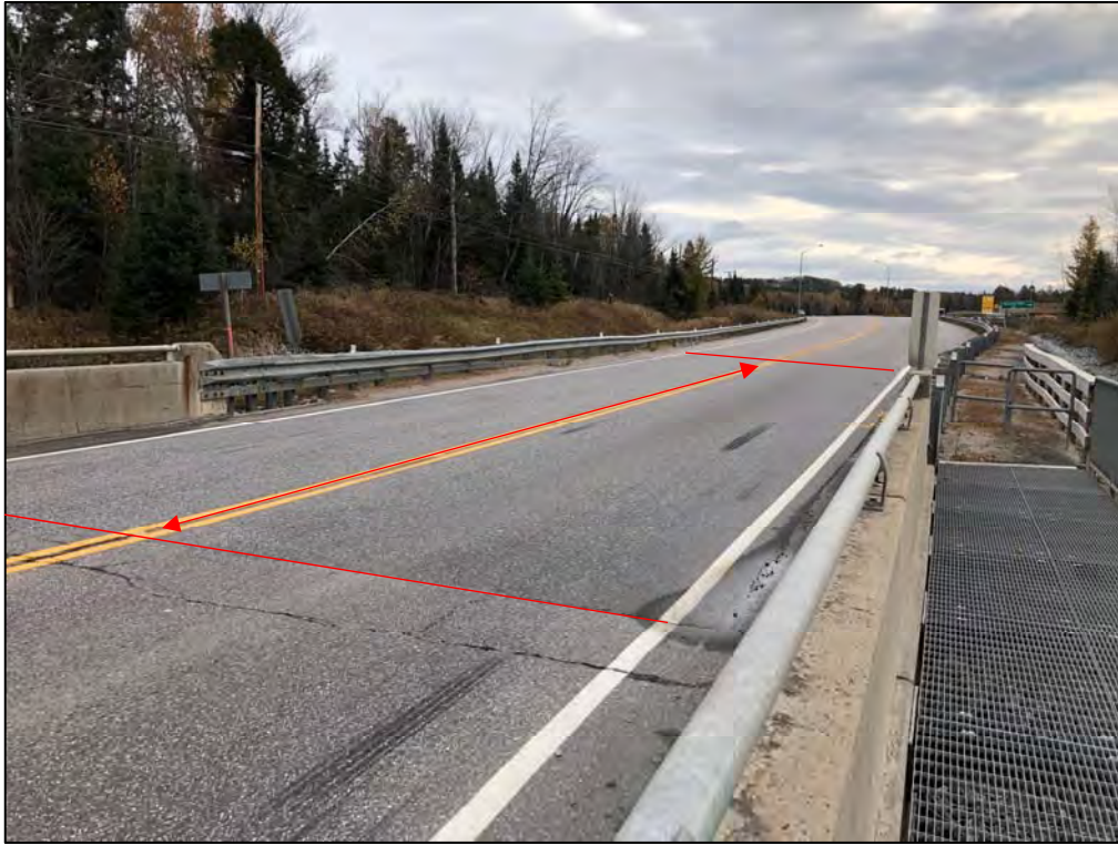
Photo 9: Newer asphalt padding on east approach [October 26, 2018]
