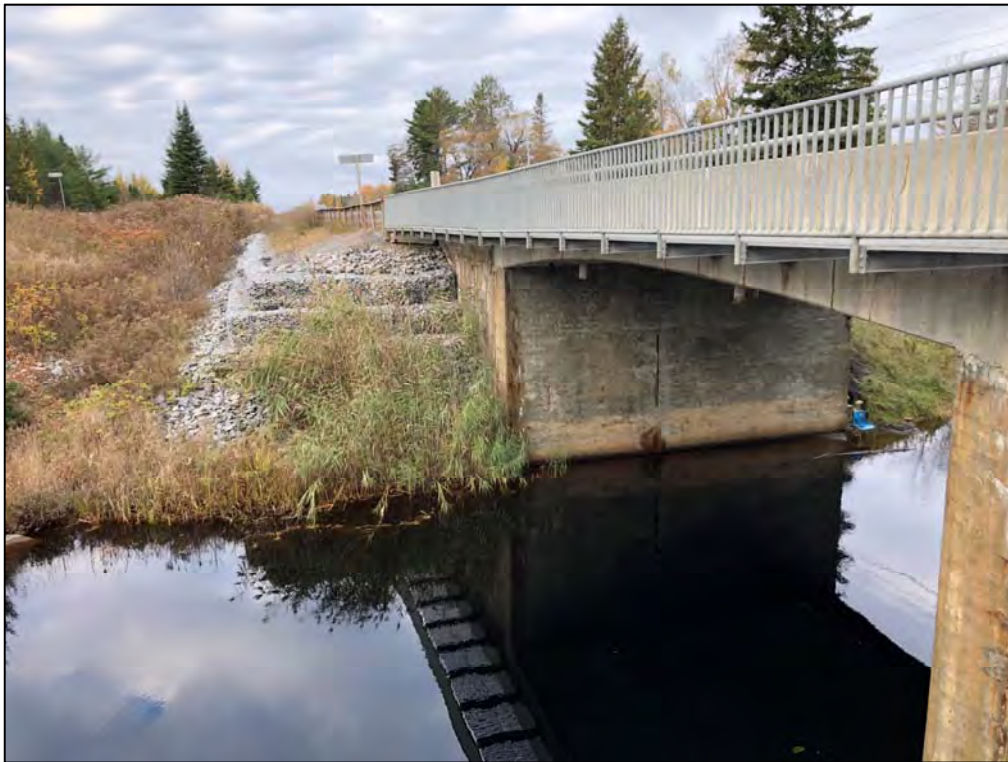
Photo 3: View of southwest gabion wall and west abutment [October 26, 2018]
