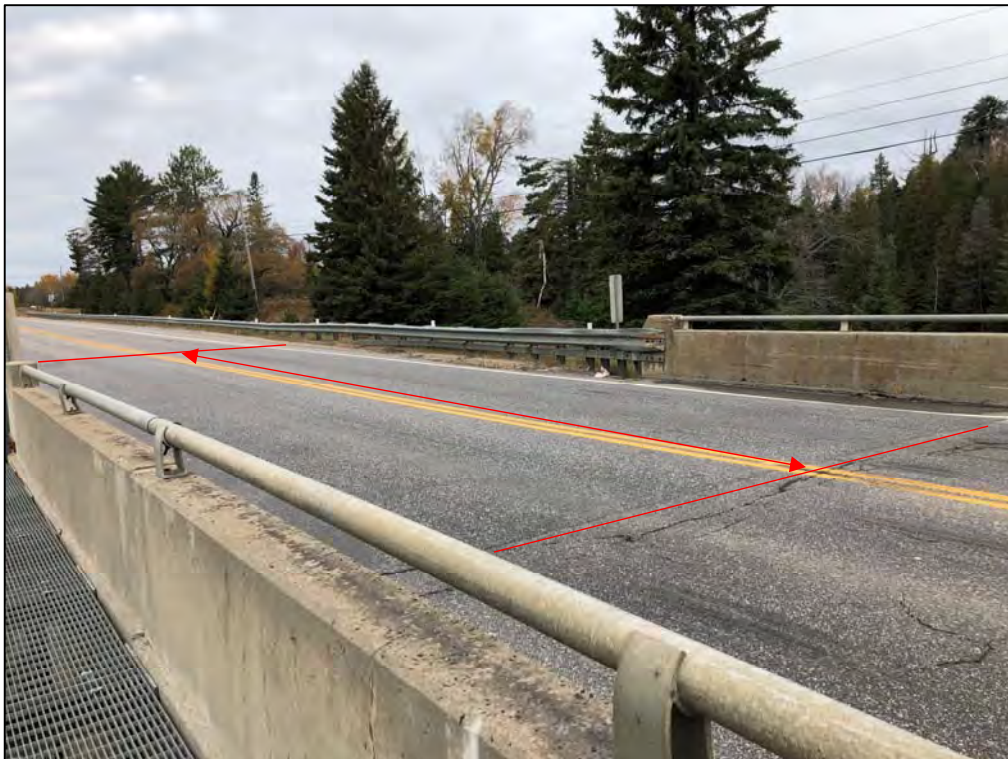
Photo 10: Newer asphalt padding on west approach [October 26, 2018]
