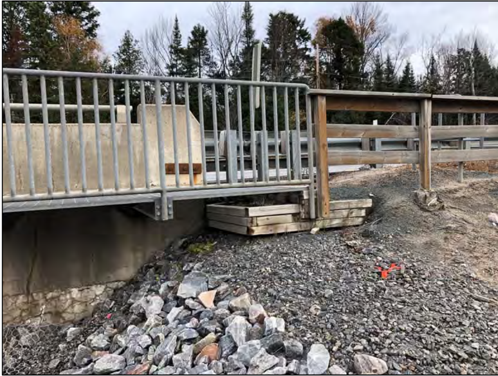
Photo 5: Erosion undermining sidewalk crib footing [October 26, 2018]
