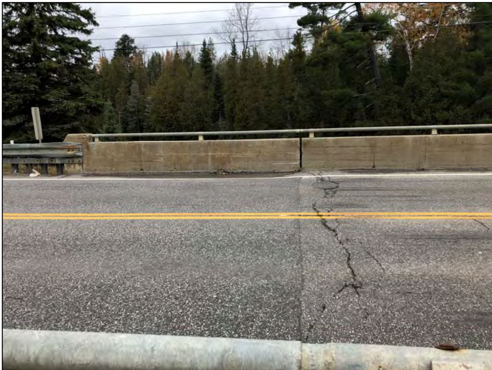
Photo 8: Tension crack above west abutment, note ponding on approach [October 26, 2018]
