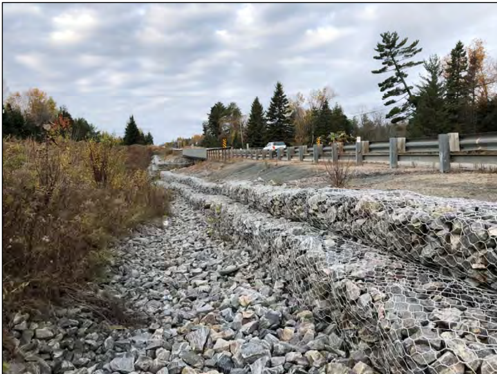
Photo 6: Southeast gabion retaining wall [October 26, 2018]
