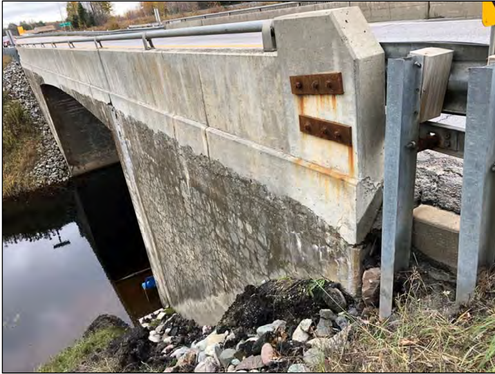
Photo 11: Erosion along northwest wing wall [October 26, 2018]
