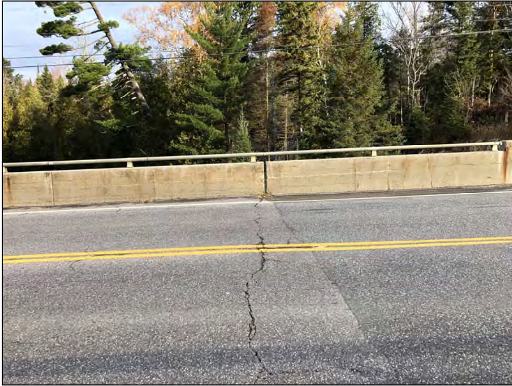
Photo 7: Tension crack above east abutment, note ponding on approach [October 26, 2018]
