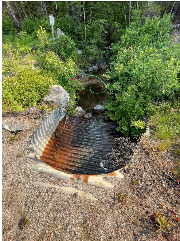
Photograph 2: Highway 17 – Clay River Culvert – Embankment West Slope at Inlet, Looking East
