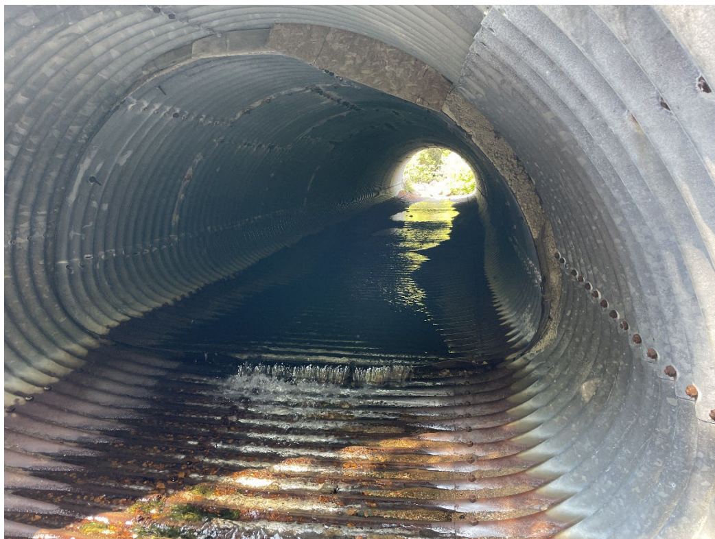
Photograph 4: Highway 17 – Clay River Culvert – Outlet
