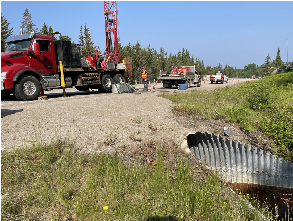
Photograph 3: Highway 17 – Clay River Culvert – Embankment East Slope at Inlet, Looking North
