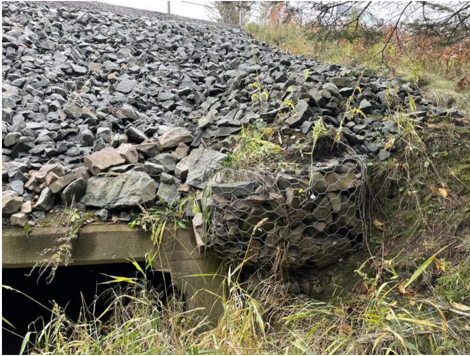
Photograph 11: Damaged Gabion Basket Wall at Outlet
