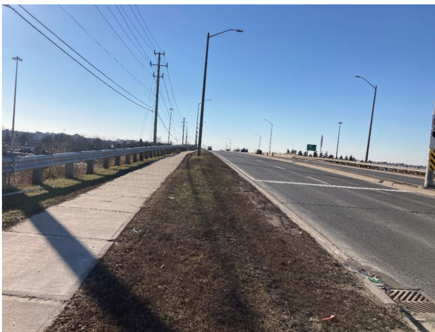
Photograph 2: Looking west at sidewalk along the crest of the southeast embankment; note the section of leaning guardrail in the background
