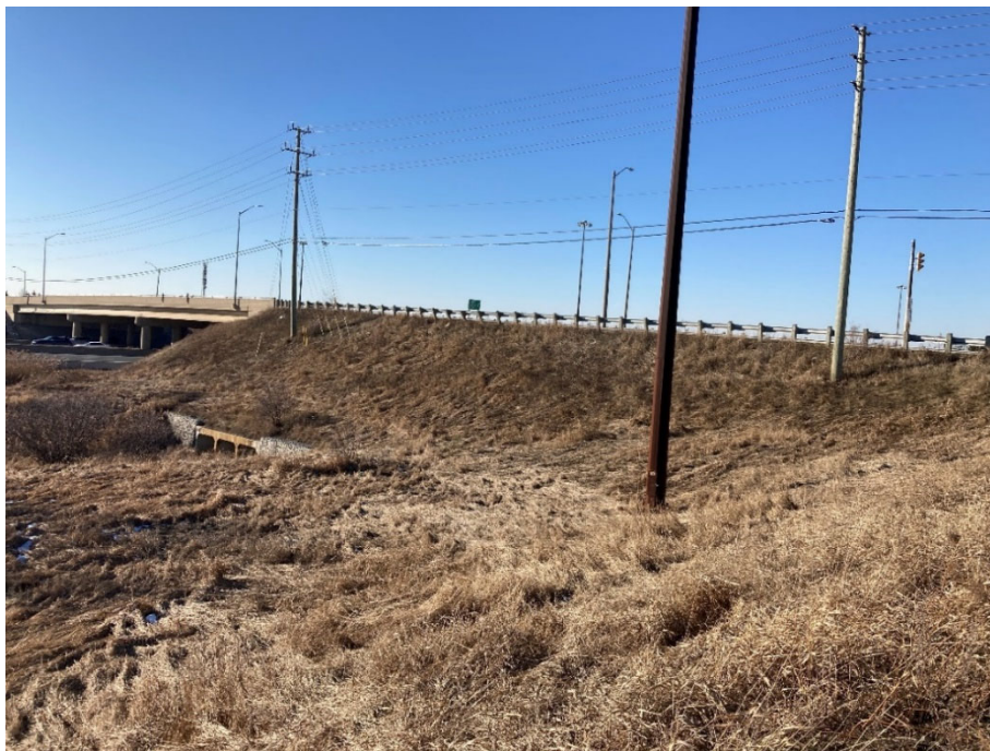
Photograph 1: Looking northwest at existing southeast embankment side slope; note the section of leaning guardrail in the background
