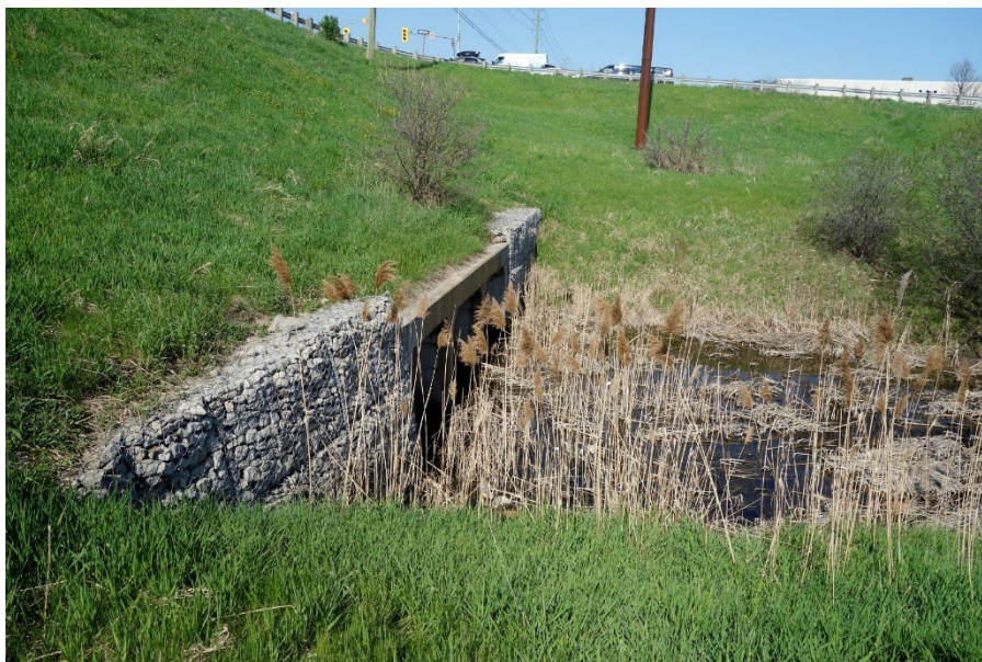
Photograph 3: Looking east towards gabion walls at Black Creek Triple Cell Culvert outlet (photograph taken at the toe of the southeast embankment)
