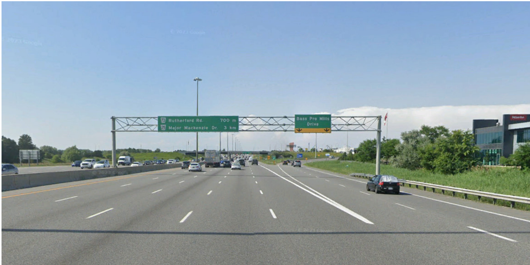
Photograph 9: Looking northbound at existing sign structure OHS-9 Existing tri-chord sign, left (median-mounted) and right (ground-mounted) footings Station 14+985
