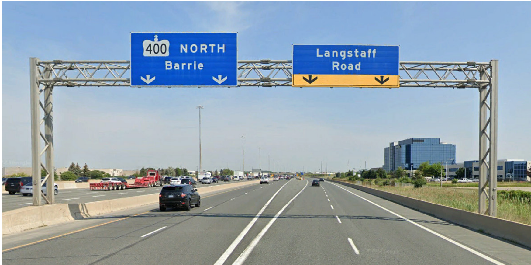
Photograph 3: Looking northbound at existing sign structure OHS-3 Existing tri-chord sign, left (median-mounted) and right (ground-mounted) footings Station 13+240
