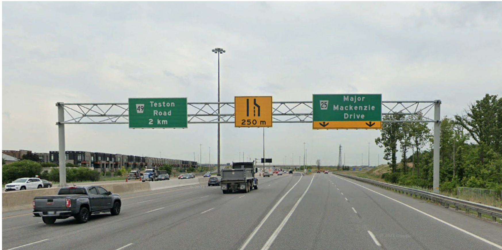
Photograph 19: Looking northbound at existing sign structure OHS-19 Existing tri-chord sign, left (median-mounted) and right (ground-mounted) footings Station 17+835
