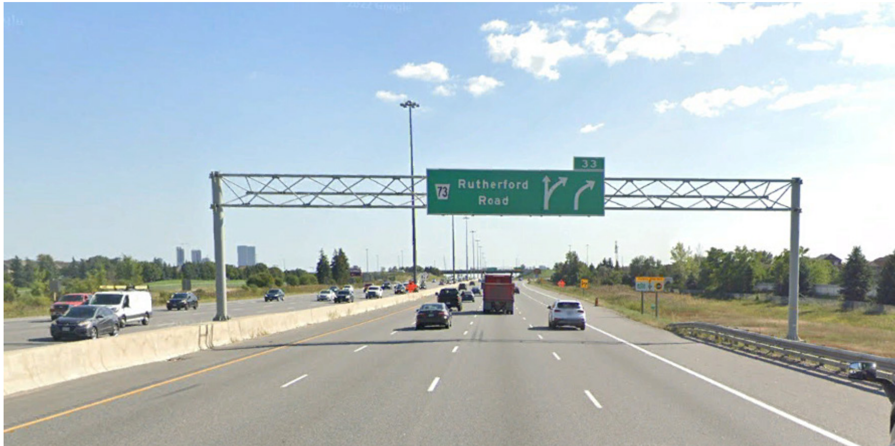
Photograph 17: Looking southbound at existing sign structure OHS-17 Existing tri-chord sign, left (median-mounted) and right (ground-mounted) footings Station 17+165
