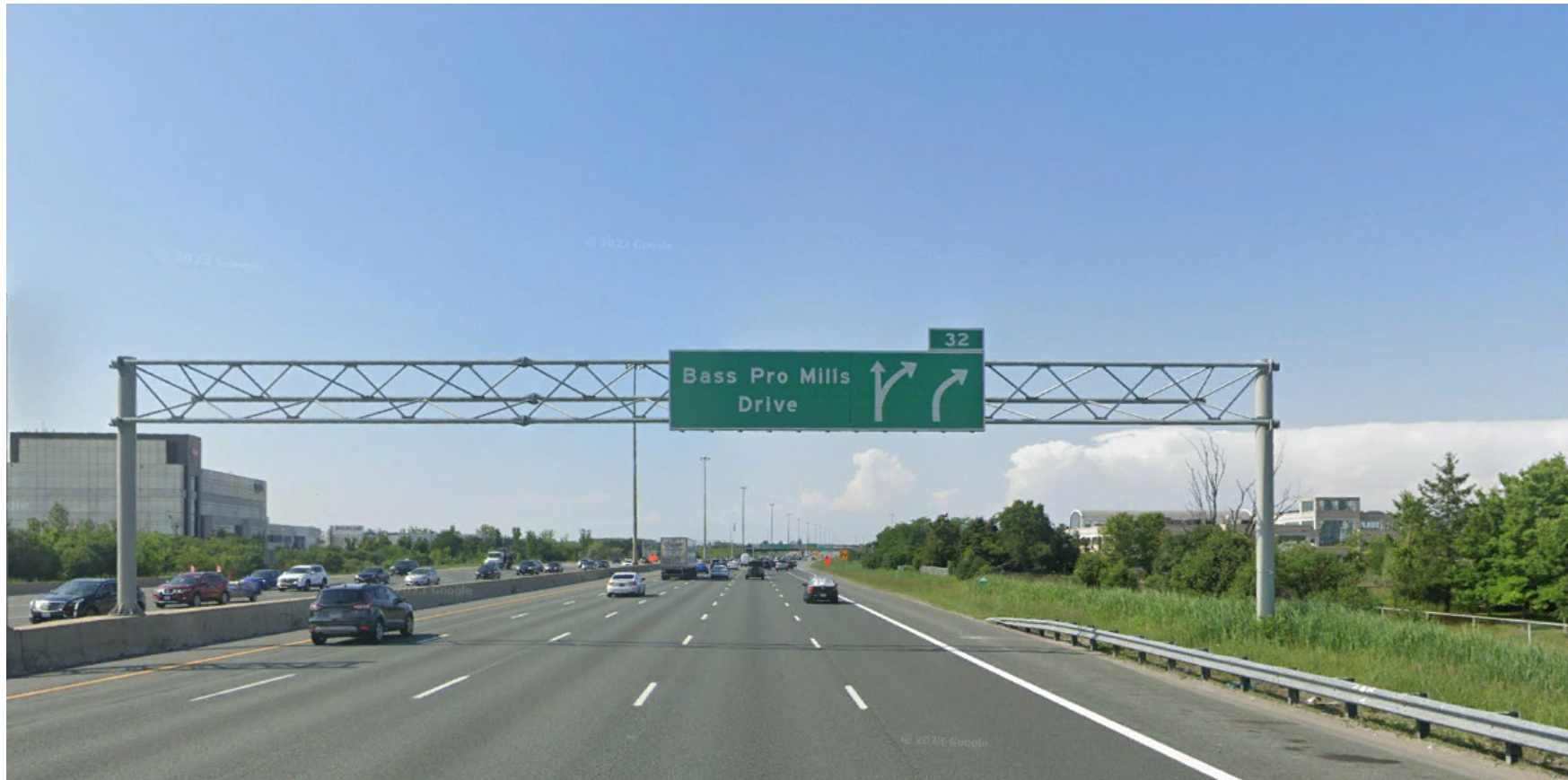
Photograph 7: Looking northbound at existing sign structure OHS-7 Existing tri-chord sign, left (median-mounted) and right (ground-mounted) footings Station 14+523
