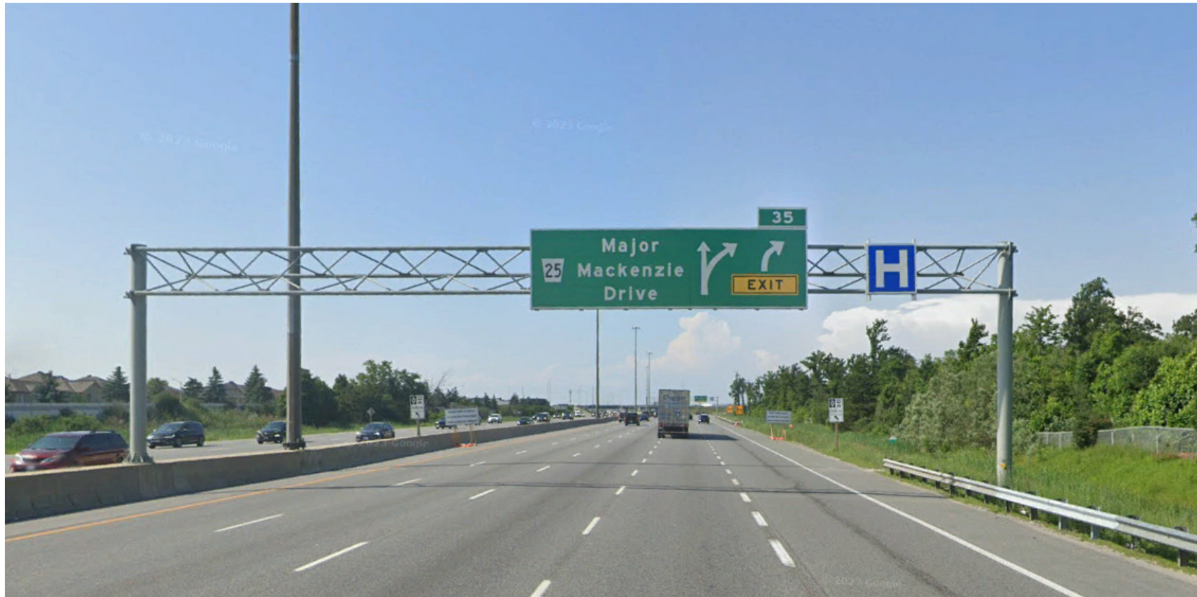
Photograph 18: Looking northbound at existing sign structure OHS-18 Existing tri-chord sign, left (median-mounted) and right (ground-mounted) footings Station 17+374
