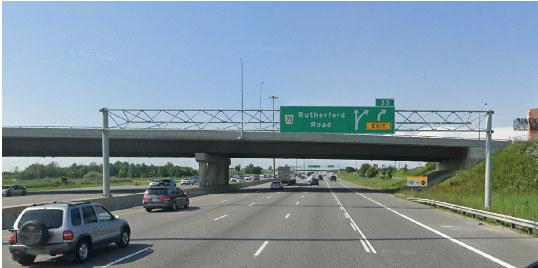
Photograph 11: Looking northbound at existing sign structure OHS-11 Existing tri-chord sign, left (median-mounted) and right (ground-mounted) footings Station 15+256
