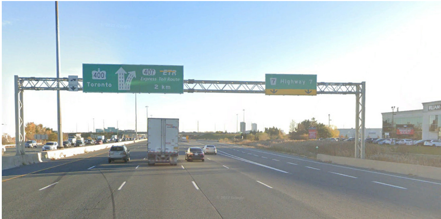
Photograph 8: Looking southbound at existing sign structure OHS-8 Existing tri-chord sign, left (median-mounted) and right (ground-mounted) footings Station 14+526
