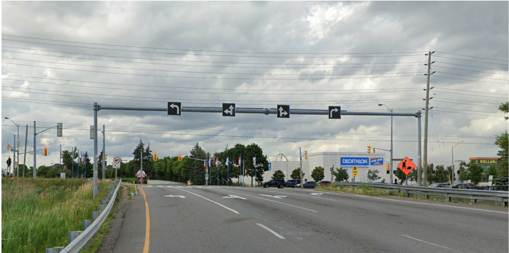
Photograph 13: Looking north at existing sign structure OHS-13 Existing monotube sign, left (ground-mounted) and right (ground-mounted) footings Rutherford S-E/W Ramp Station 10+381
