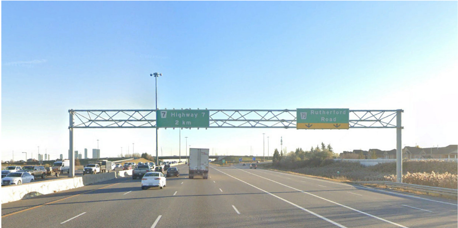
Photograph 16: Looking southbound at existing sign structure OHS-16 Existing tri-chord sign, left (median-mounted) and right (ground-mounted) footings Station 16+704
