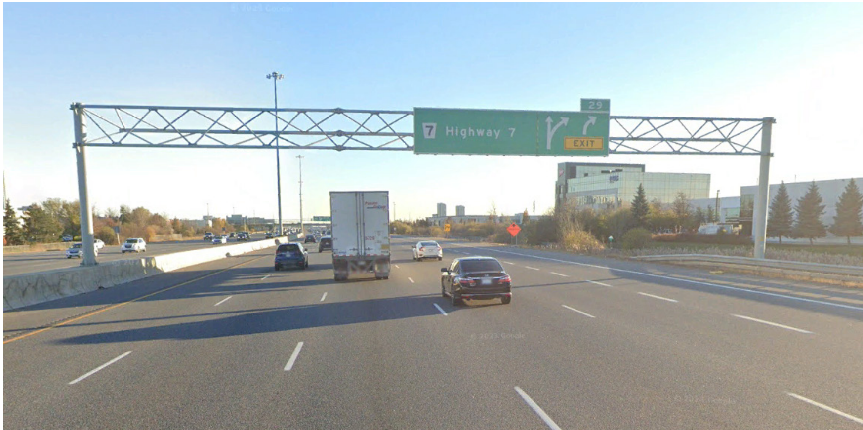
Photograph 10: Looking southbound at existing sign structure OHS-10 Existing tri-chord sign, left (median-mounted) and right (ground-mounted) footings Station 14+988
