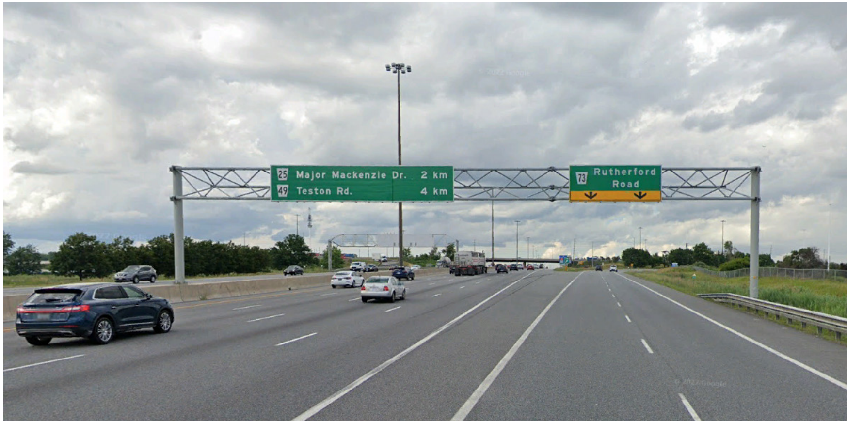
Photograph 12: Looking northbound at existing sign structure OHS-12 Existing tri-chord sign, left (median-mounted) and right (ground-mounted) footings Station 15+719
