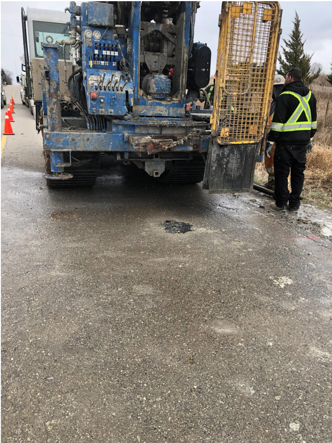
Photograph 3: Borehole 9CULV-03 upon completion, Looking North
