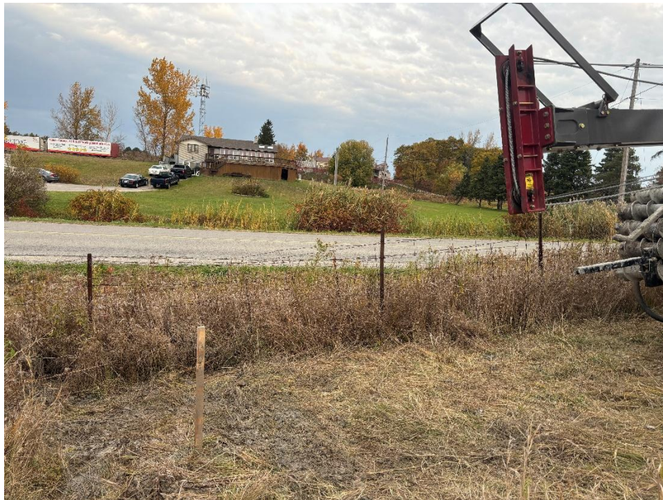
Photograph 2: Borehole 9CULV-03 upon completion, Looking North
