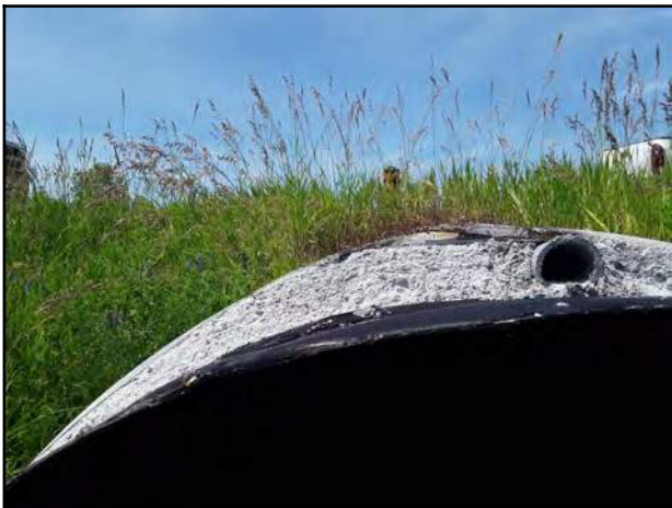
Photo 35 - Annular space of 80 mm between existing pipe and sliplined culvert at inlet.
