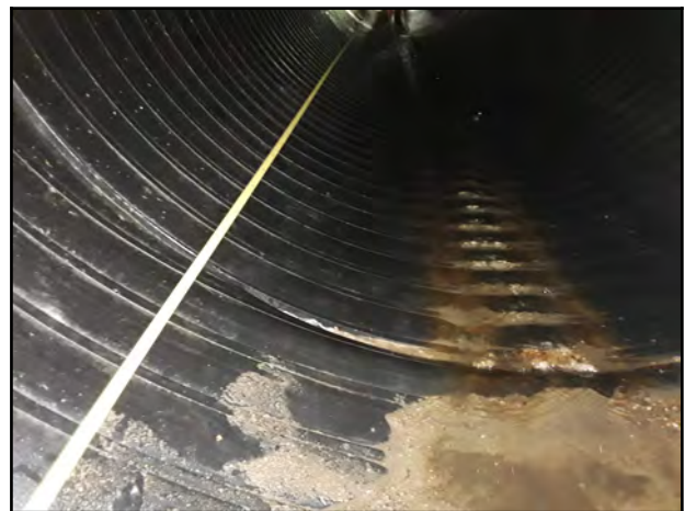
Photo 18 - V-2: Pipe sections overlapping at joint.
