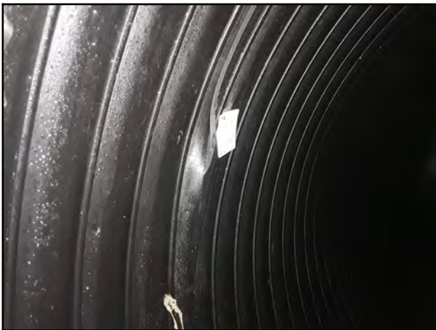
Photo 21 - V-5: Localized damage at joint.
