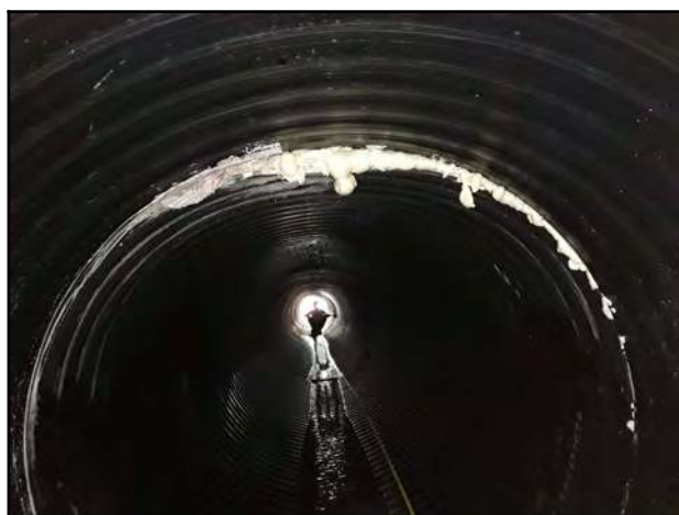
Photo 23 - V-5: Offset joint by approximately 40 mm with visible grouting and foam.
