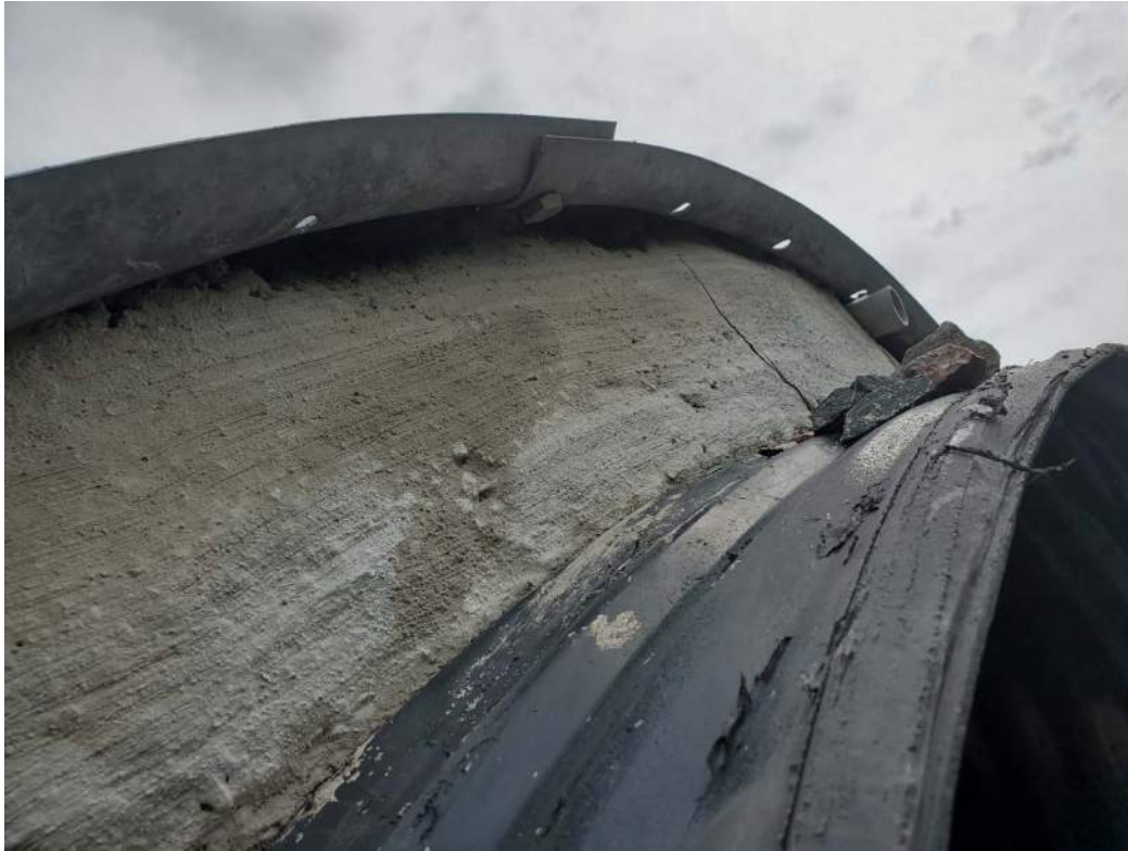
Photo 3: Minimal hairline fractures observed in grout at inlet and outlet in both culverts
