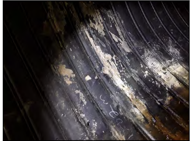
Photo 14 - V-2: Joint with visible expansion foam.
