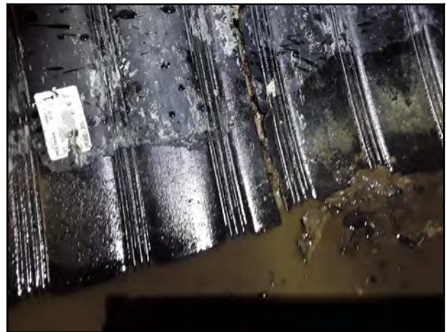
Photo 16 - V-2: Joint with visible expansion foam and visible supporting material.
