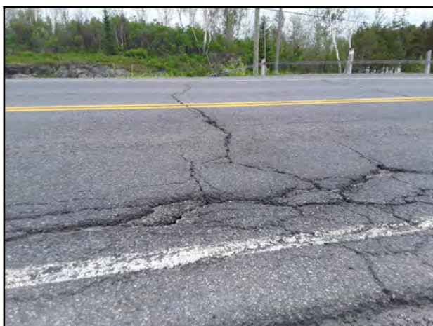
Photo 3 - Pothole measuring approximately 100 mm in-depth not directly over pipe.
