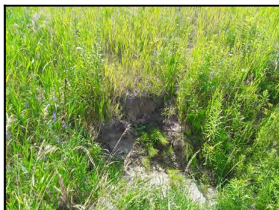
Photo 4 - Minor soil movement at the outlet embankment.
