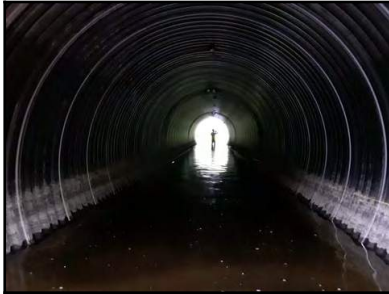
Photo 12 - Upstream pipe alignment and shape.
