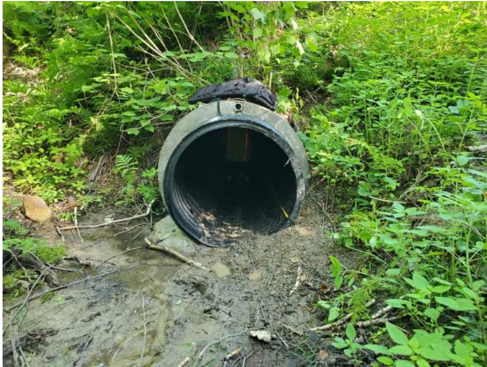
Photo 1: South end of culvert (inlet) exhibiting good grout condition and cut off grout pipe – looking north
