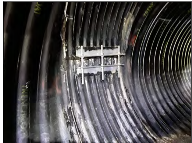
Photo 16 - V-2: Joint with visible expansion foam and grout buildup on the invert.
