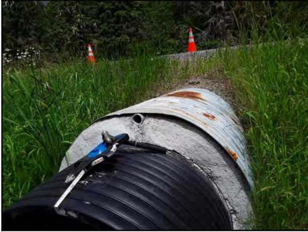
Photo 25 - Annular space of 170 mm between the existing CMP and the sliplined HDPE at outlet.
