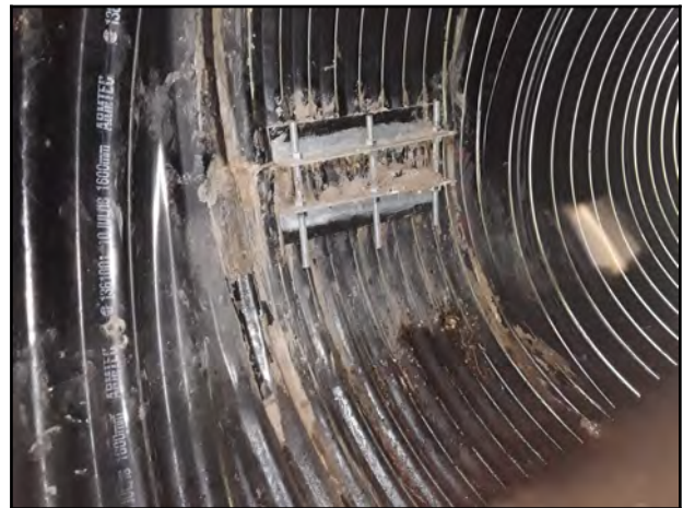
Photo 28 - V-6: Joint with visible expansion foam.
