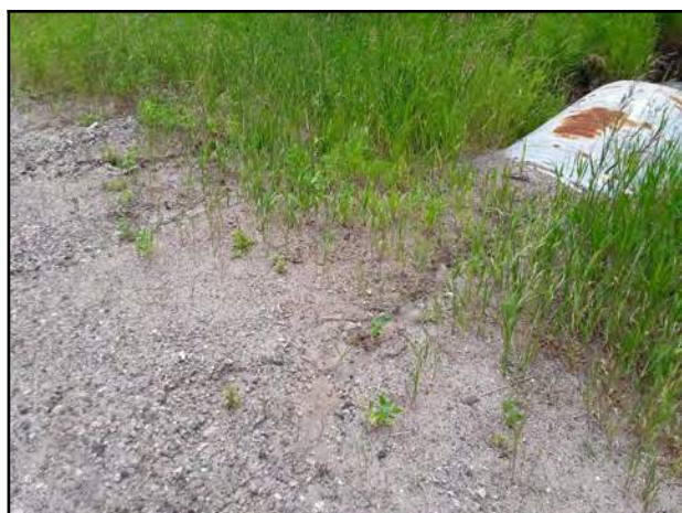
Photo 3 - Minor erosion channels on the outlet embankment with the most severe measuring approximately 190 mm in width.
