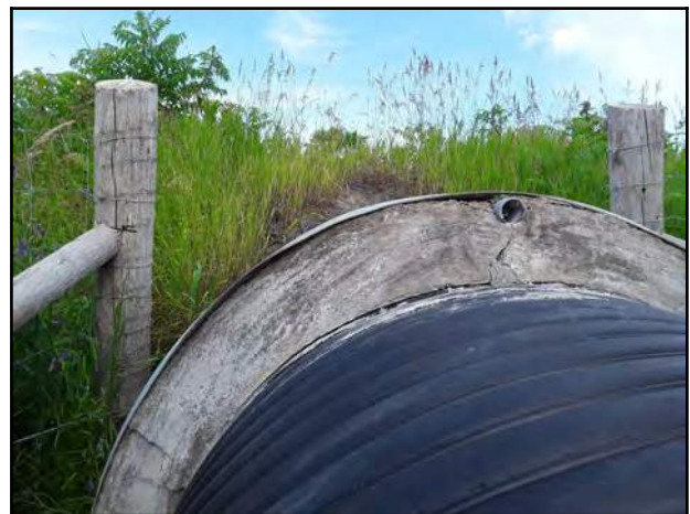
Photo 30 - Annular space of 230 mm between the existing CMP and the sliplined HDPE at outlet.
