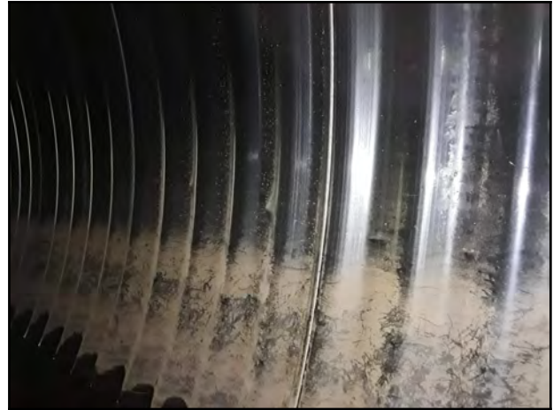
Photo 20 - V-3: Minor dents protruding approximately 15 mm.
