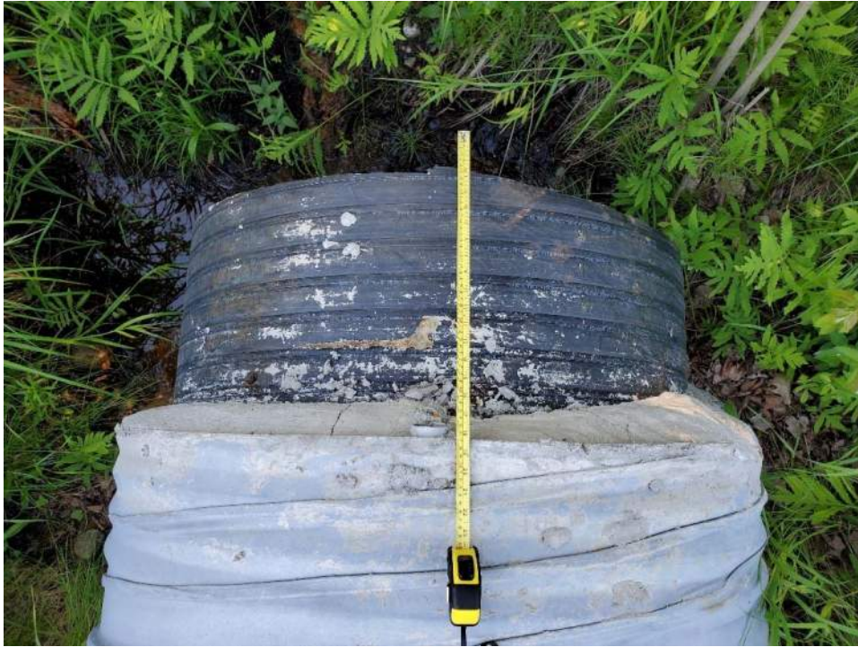
Photo 3 – Inlet looking down at grout protruding ~30 to 70mm
