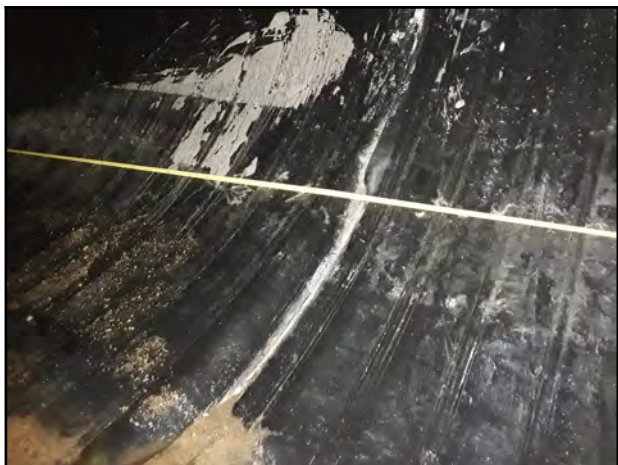
Photo 25 - V-6: Pipe sections overlapping at joint with foam evident.
