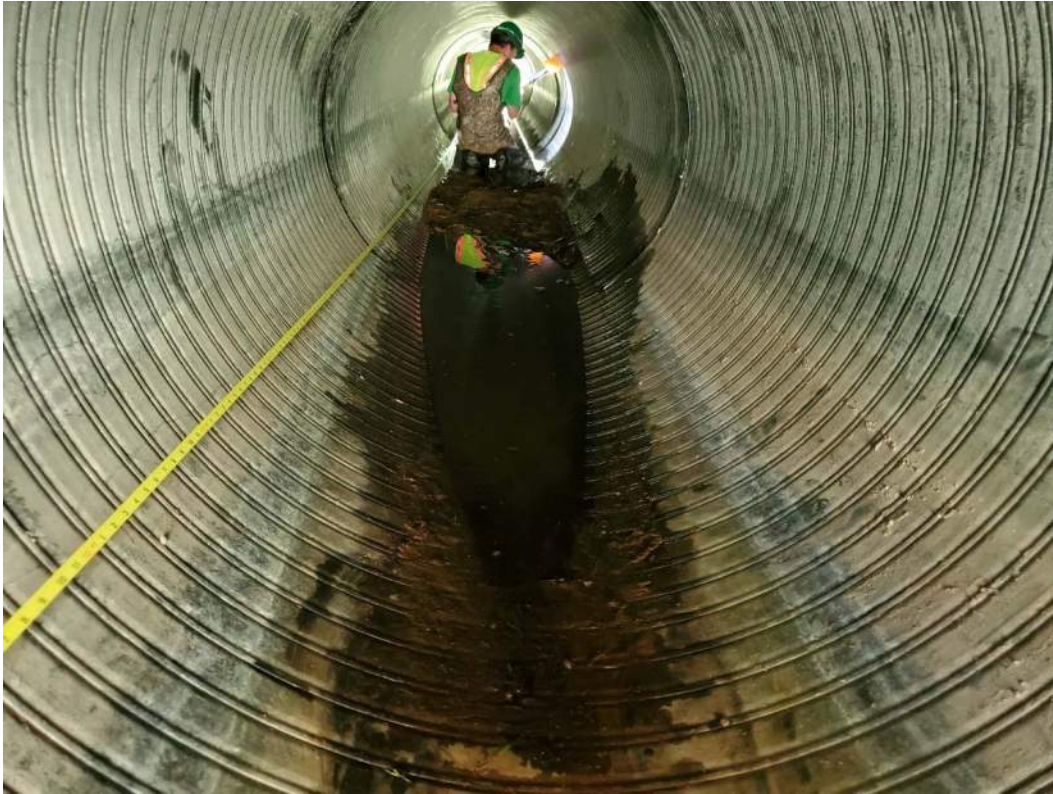
Photo 3: Basal sediment/muck observed from approx. 3.4m from inlet to outlet – looking south towards outlet
