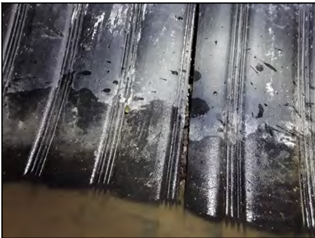
Photo 15 - V-2: Joint with visible expansion foam and visible supporting material.
