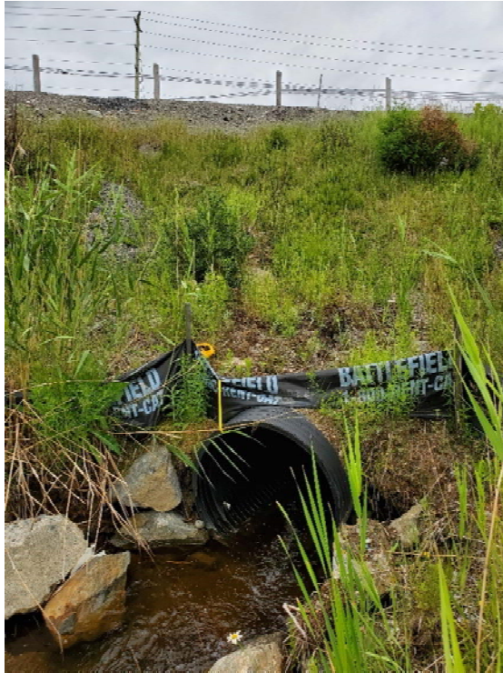
Photo 1: Grout and host pipe not visible at north end of culvert (outlet) – looking south
