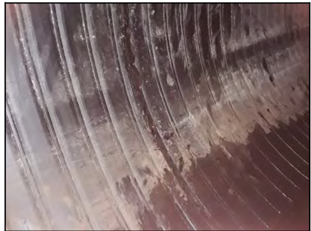
Photo 16 - V-2: Joint with evident black caulking.
