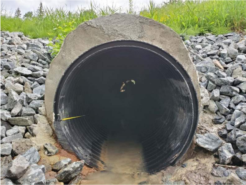
Photo 1: East end of culvert (outlet) surrounded by rip rap embankment exhibiting low flow and no visual grout pipes. – looking west
