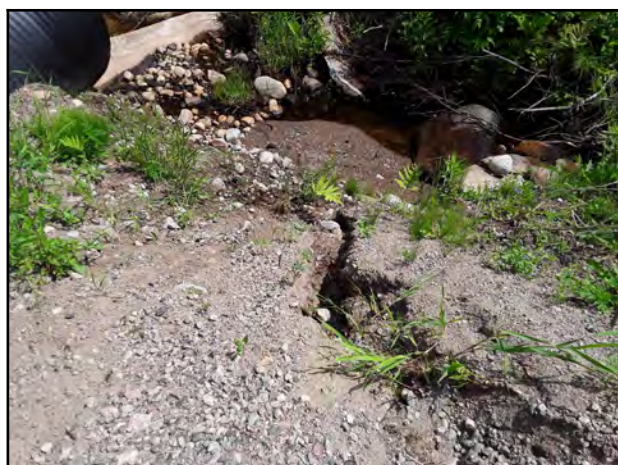
Photo 3 - Erosion channel on the outlet embankment measuring approximately 300 mm in width.
