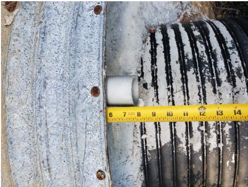
Photo 4: Approximately 150mm host pipe left unfilled with grout at south end of culvert.
