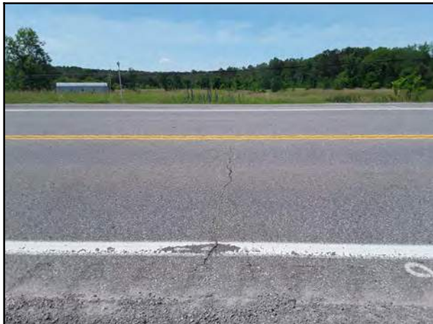
Photo 1 - Transverse crack present above the asset.
