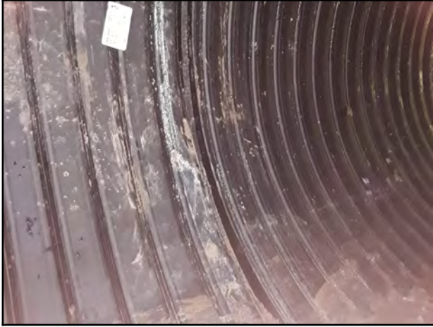
Photo 25 - V-6: Separated joint by approximately 40 mm with minor localized damage evident.
