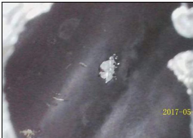
Photo 25 - V-3: Endoscope camera placed in the probe hole showing void.
