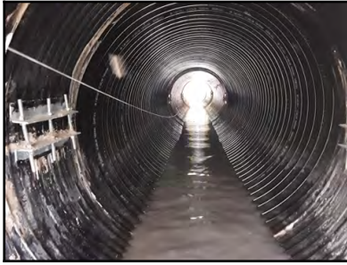
Photo 11 - Upstream pipe alignment and shape.
