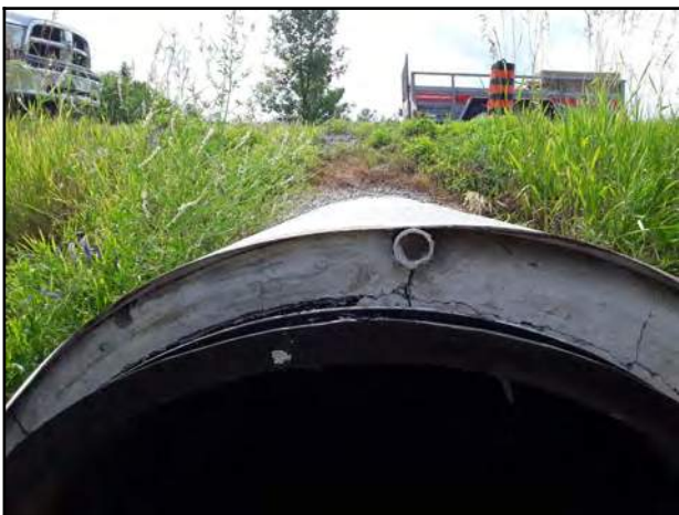
Photo 29 - Annular space of 240 mm between the existing CMP and the sliplined HDPE at inlet.
