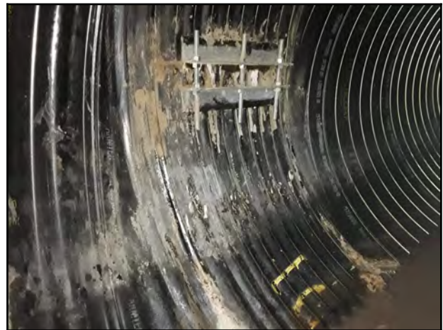
Photo 22 - V-4: Joint with visible expansion foam.
