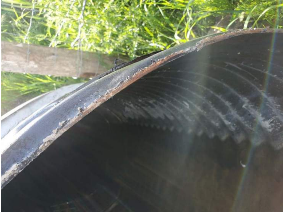
Photo 3 – Rust on steel/metal liner pipe at outlet
