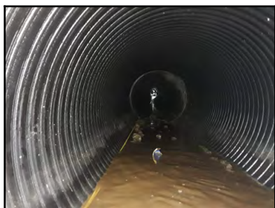
Photo 10 - Upstream pipe alignment and shape.
