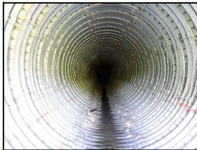
Photo 7 - Downstream pipe alignment and shape.
