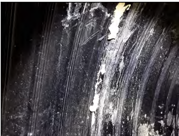
Photo 17 - V-2: Joint with visible expansion foam and visible supporting material.
