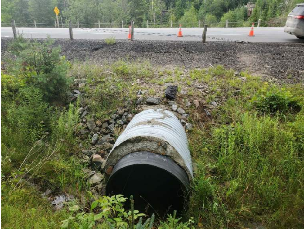
Photo 1: Inlet liner with irregular grouting between host pipe – looking east
