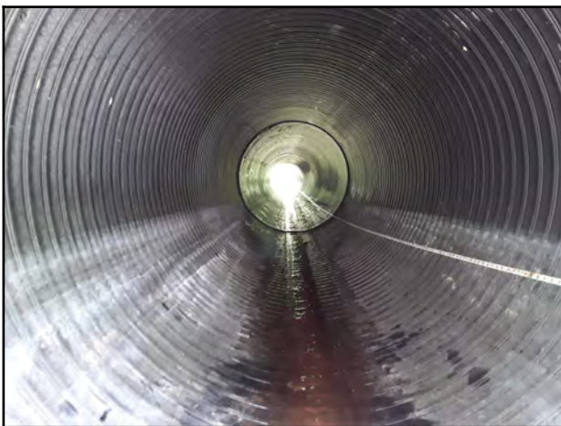
Photo 11 - Upstream pipe alignment and shape.
