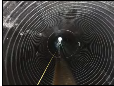
Photo 12 - Downstream pipe alignment and shape.
