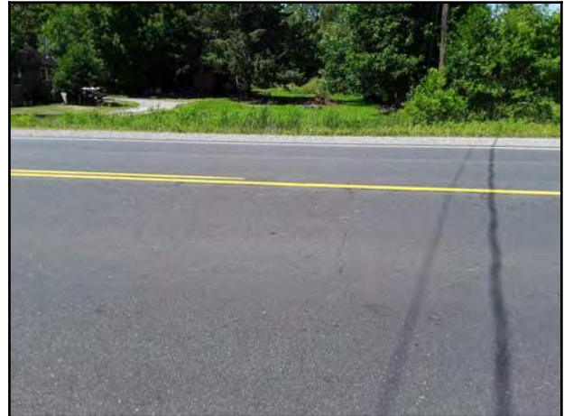
Photo 2 - Light transverse cracks.
