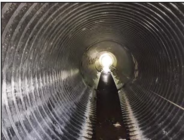
Photo 11 - Downstream pipe alignment and shape.
