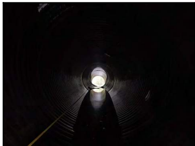
Photo 13 - Pooling of approximately 100 mm evident within pipe due to the vertical misalignment at the outlet end.
