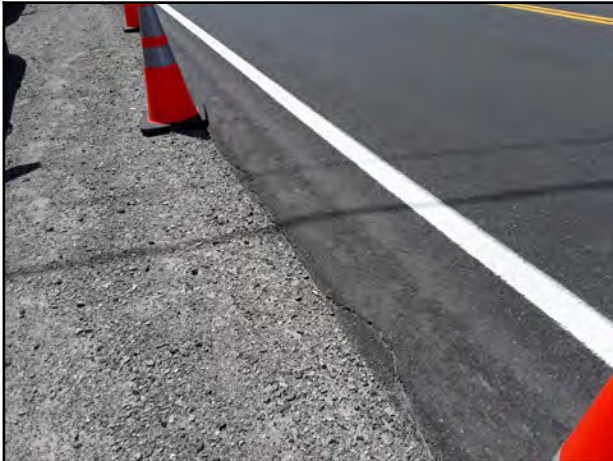
Photo 1 - Light progressive edge cracking on outlet side.
