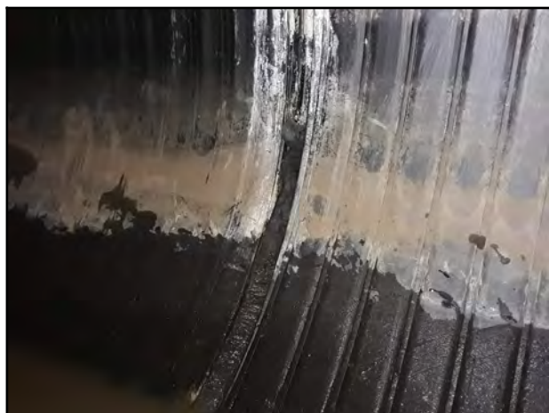
Photo 21 - V-4: Separated joint by approximately 40 mm with black caulking evident.
