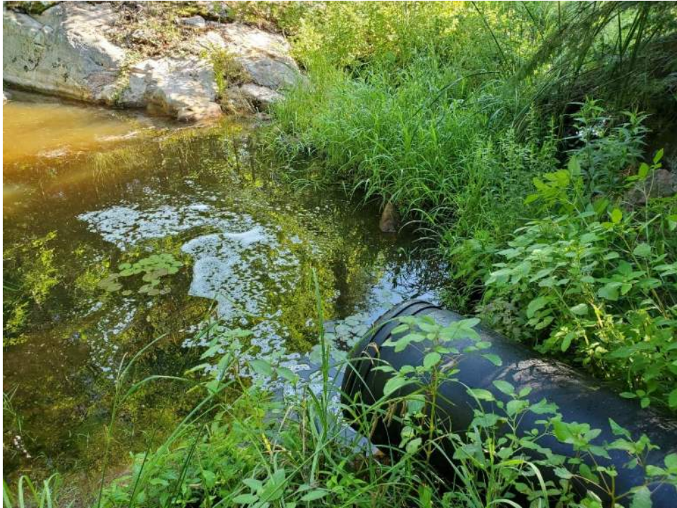
Photo 1: Outlet liner (Host pipe buried in embankment)– looking northeast
