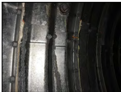
Photo 5 - Level 1 water infiltration evident at seam bolt hole locations throughout the entire culvert.
