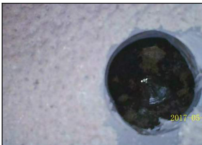
Photo 29 - V-7: Endoscope camera placed in the probe hole showing some void since host pipe is resting on Sliplined HDPE.
