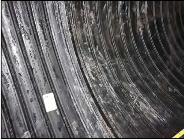
Photo 19 - V-4: Separated joint by approximately 40 mm.
