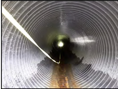
Photo 16 - Upstream pipe alignment and shape.
