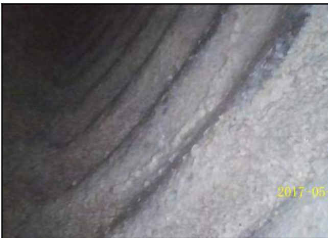
Photo 17 - V-2: Endoscope camera placed in the probe hole showing void.
