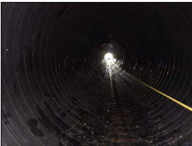
Photo 11 - Downstream pipe alignment and shape.
