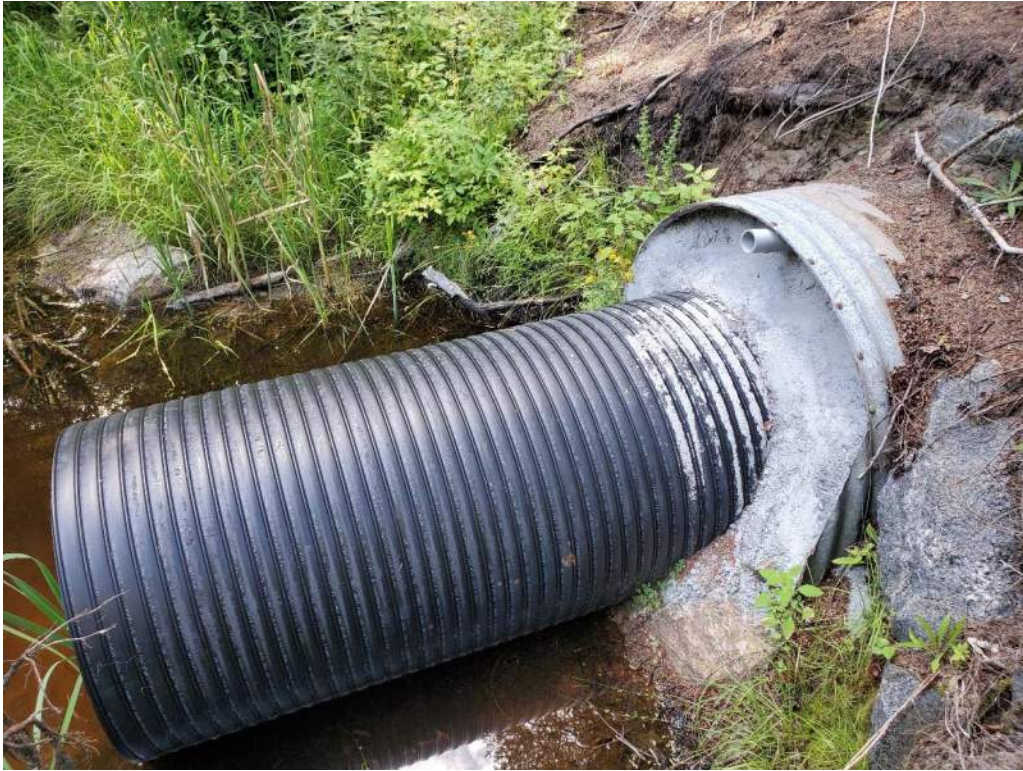
Photo 3: South end of culvert with one cut off grout pipe exposed– looking west
