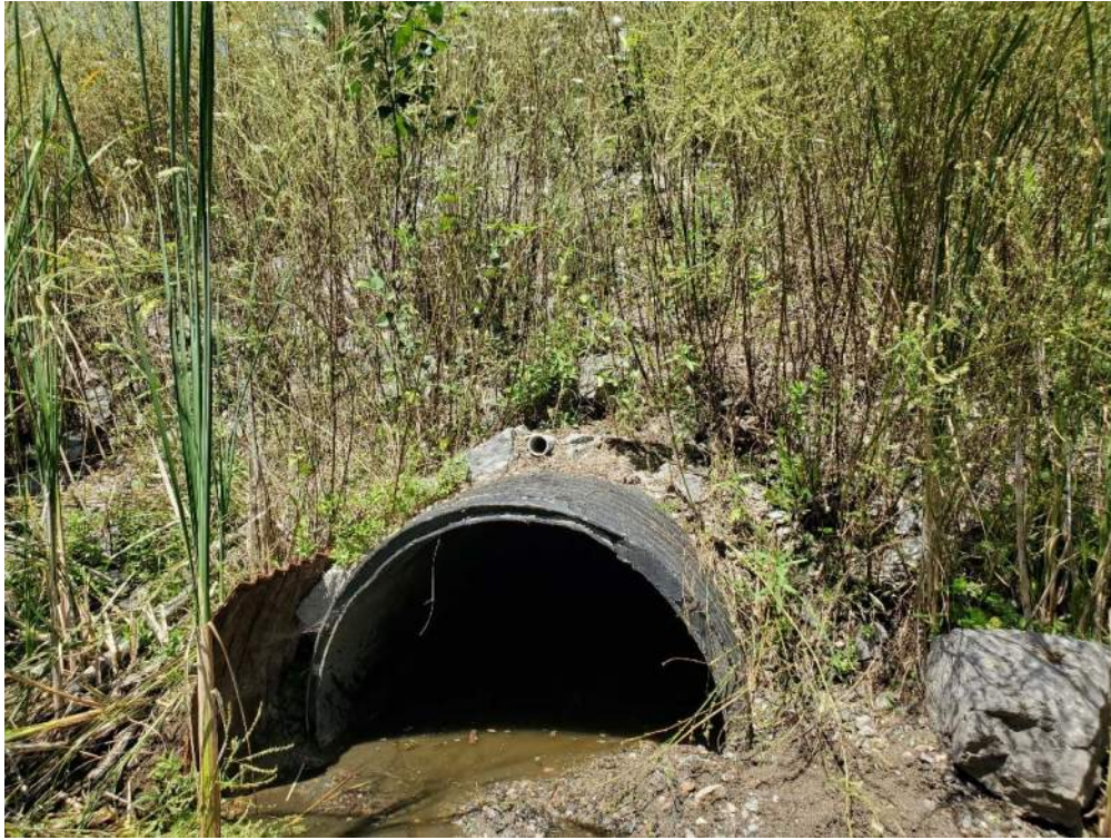
Photo 3: Excessive sediment at south end of culvert – looking north
