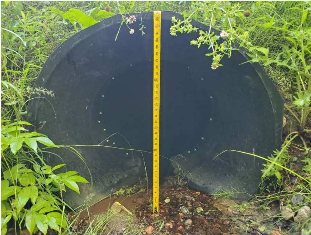
Photo 3: West end of culvert (inlet) trumpet entrance telescoping to smaller diameter liner. Host pipe not visible - looking south
