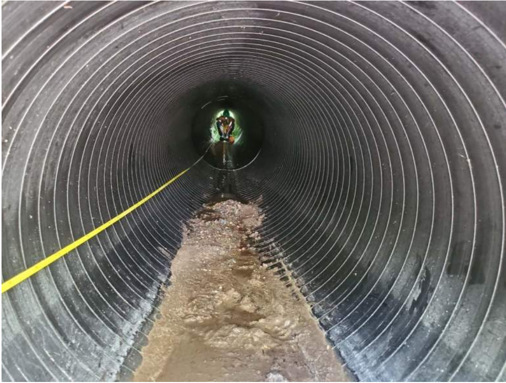
Photo 3: Minimal basal sediments observed near culvert outlet– looking south
