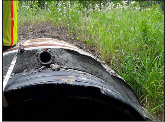
Photo 26 - Annular space of 120 mm between the existing CMP and the sliplined HDPE at inlet.
