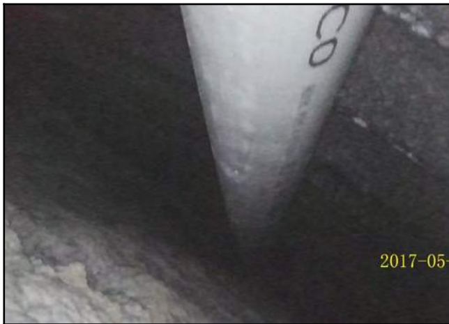
Photo 15 - V-1: Endoscope camera placed in the probe hole showing void.
