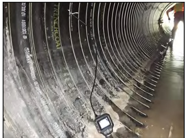
Photo 24 - V-5: Endoscope camera showing visible void.
