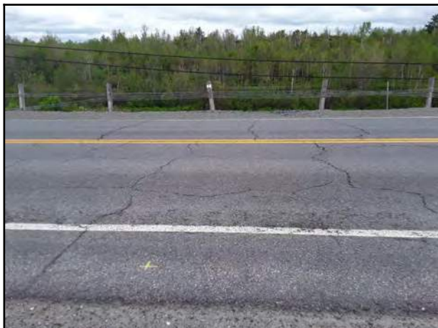
Photo 1 - Multiple severe transverse and longitudinal cracks directly above the pipe.
