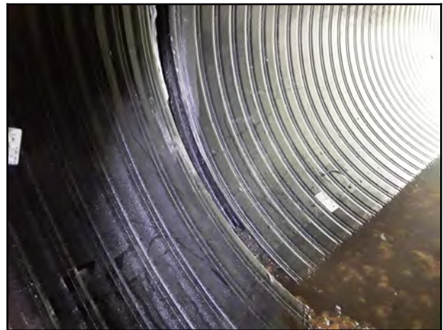
Photo 16 - V-2: Separated joint of approximately 70 mm with visible supporting grout material.
