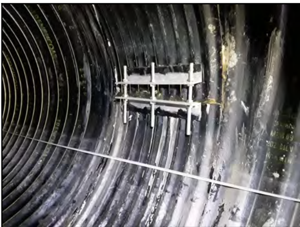
Photo 17 - V-2: Joint with visible expansion foam and grout buildup on the invert.
