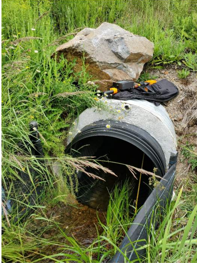
Photo 3: South end of culvert (inlet) exhibits good grout condition. Cut off grout pipe observed in grout fill. - looking north
