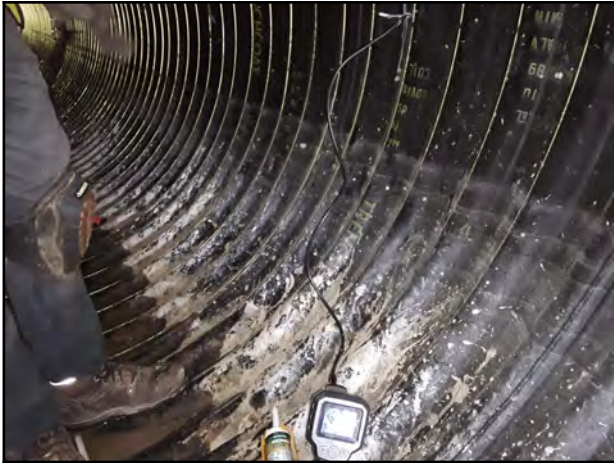
Photo 19 - V-3: Endoscope camera showing visible void.
