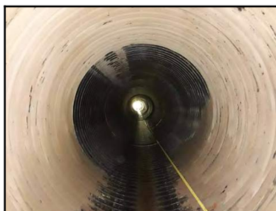
Photo 11 - Downstream pipe alignment and shape.
