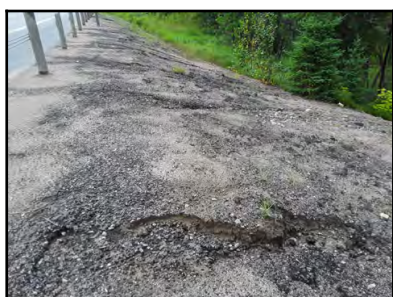
Photo 7 - Multiple erosion channels on the outlet embankment with the most severe measuring approximately 400 mm in width.
