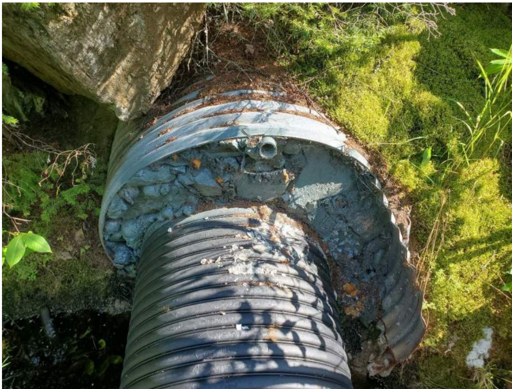
Photo 2: Voids at north end of culvert filled with cobbles and spray foam insulation – looking south
