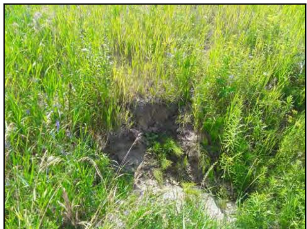
Photo 4 - Minor soil movement at the outlet embankment.
