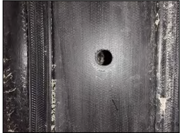
Photo 14 - V-1: Endoscope camera showing visible void.
