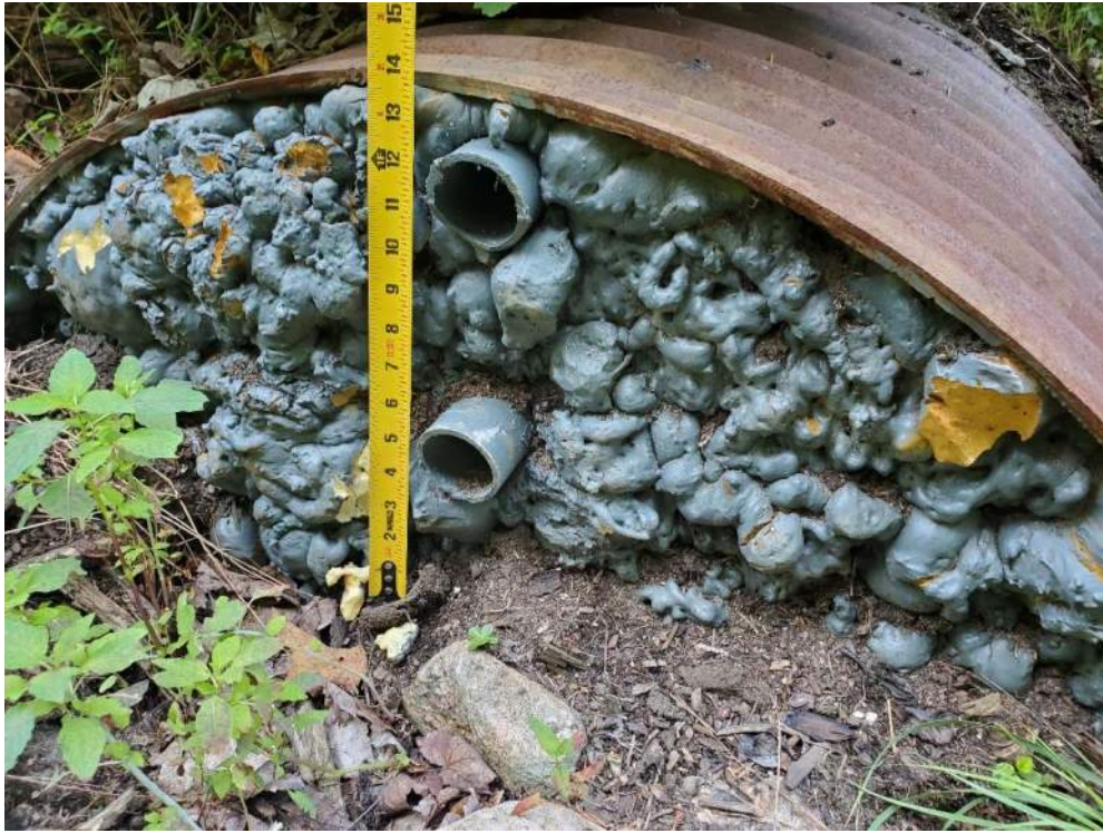
Photo 3: Damaged host pipe filled with spray foam insulation at inlet
