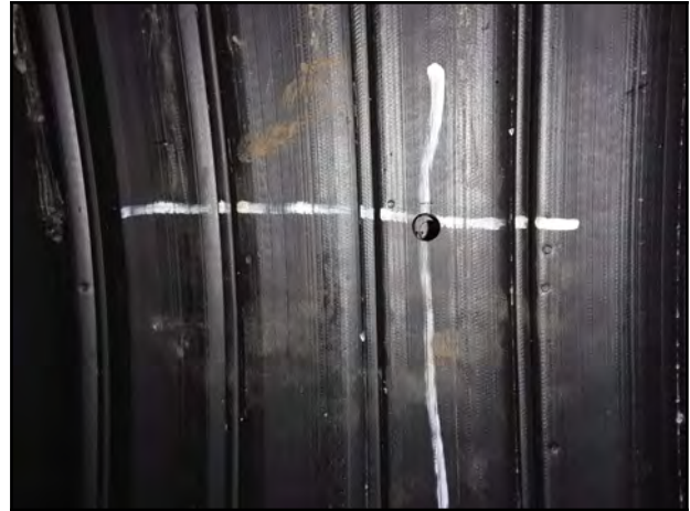
Photo 26 - V-6: Endoscope camera showing visible void.
