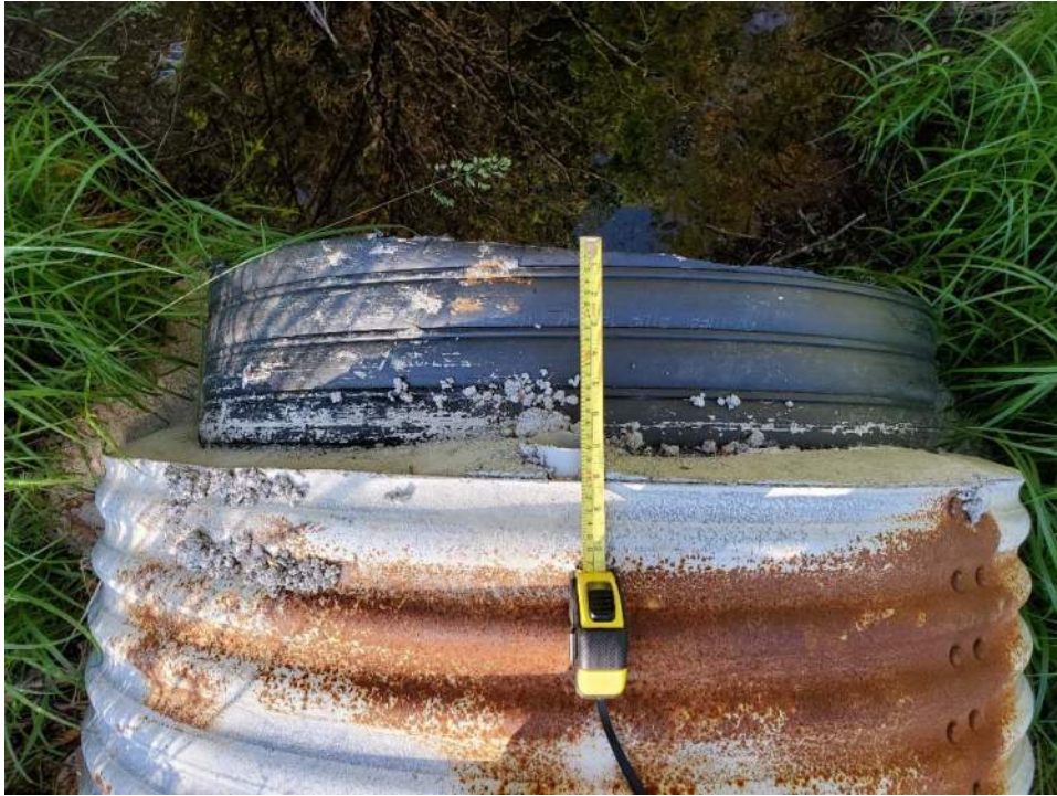
Photo 3 – Inlet looking down at grout protruding ~30 mm
