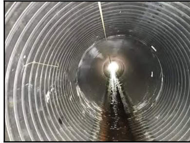
Photo 11 - Downstream pipe alignment and shape.
