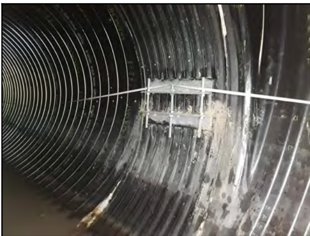
Photo 23 - V-4: Joint with visible expansion foam.
