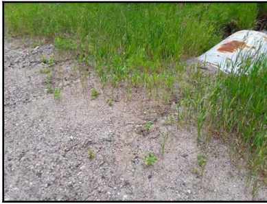
Photo 3 - Minor erosion channels on the outlet embankment with the most severe measuring approximately 190 mm in width.
