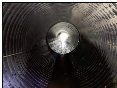
Photo 12 - Downstream pipe alignment and shape.
