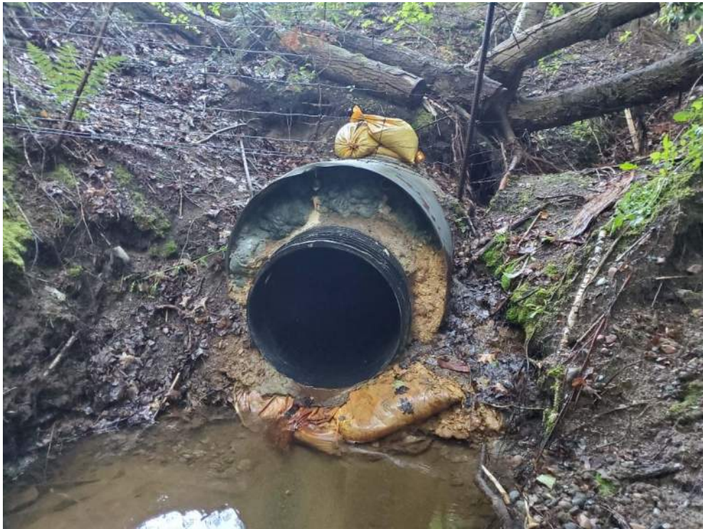
Photo 1: East end of culvert (outlet) in poor condition. Spray foam and sandy material utilized to fill voids – looking west
