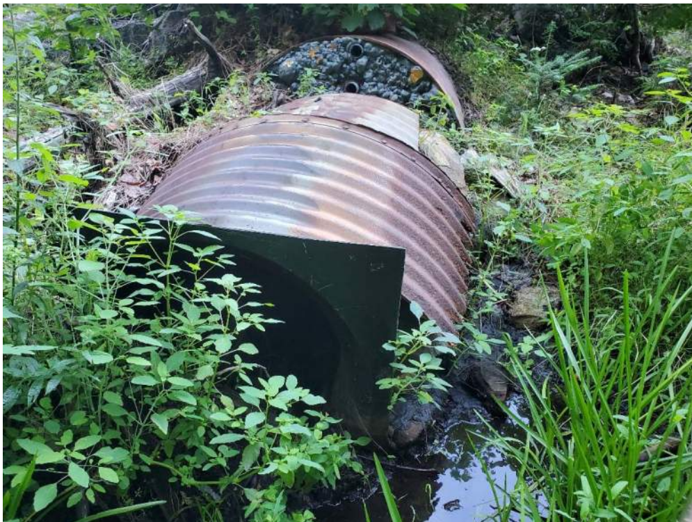
Photo 2: Liner observed in severely damaged inlet (no flow)– looking northwest
