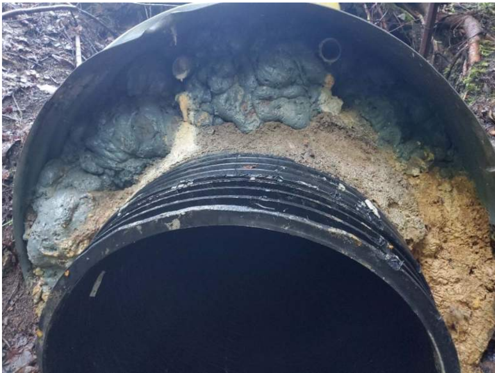
Photo 2: Cut off grout pipes noted, but no grout is visible at culvert outlet. Bulkhead appears to consist solely of spray foam and sandy material – looking west
