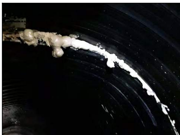
Photo 21 - V-5: Offset joint by approximately 40 mm with visible grouting and foam.
