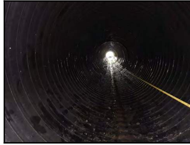
Photo 11 - Downstream pipe alignment and shape.
