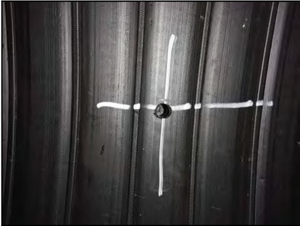
Photo 13 - V-1: Endoscope camera showing visible void.
