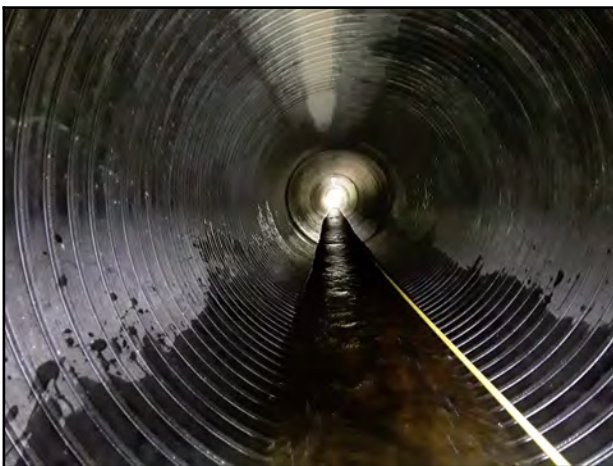
Photo 17 - Downstream pipe alignment and shape.
