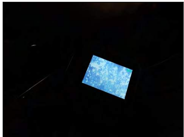
Photo 18 - V-3: Endoscope camera showing visible void.
