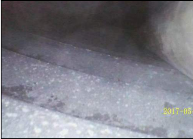
Photo 19 - V-1: Endoscope camera placed in the probe hole showing void.
