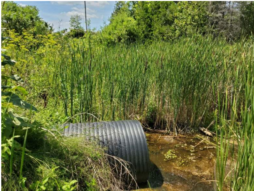
Photo 4: Marshy area with bulrushes and significant basal sediment at south end of culvert. – looking east
