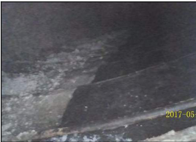
Photo 21 - V-2: Endoscope camera placed in the probe hole showing void.
