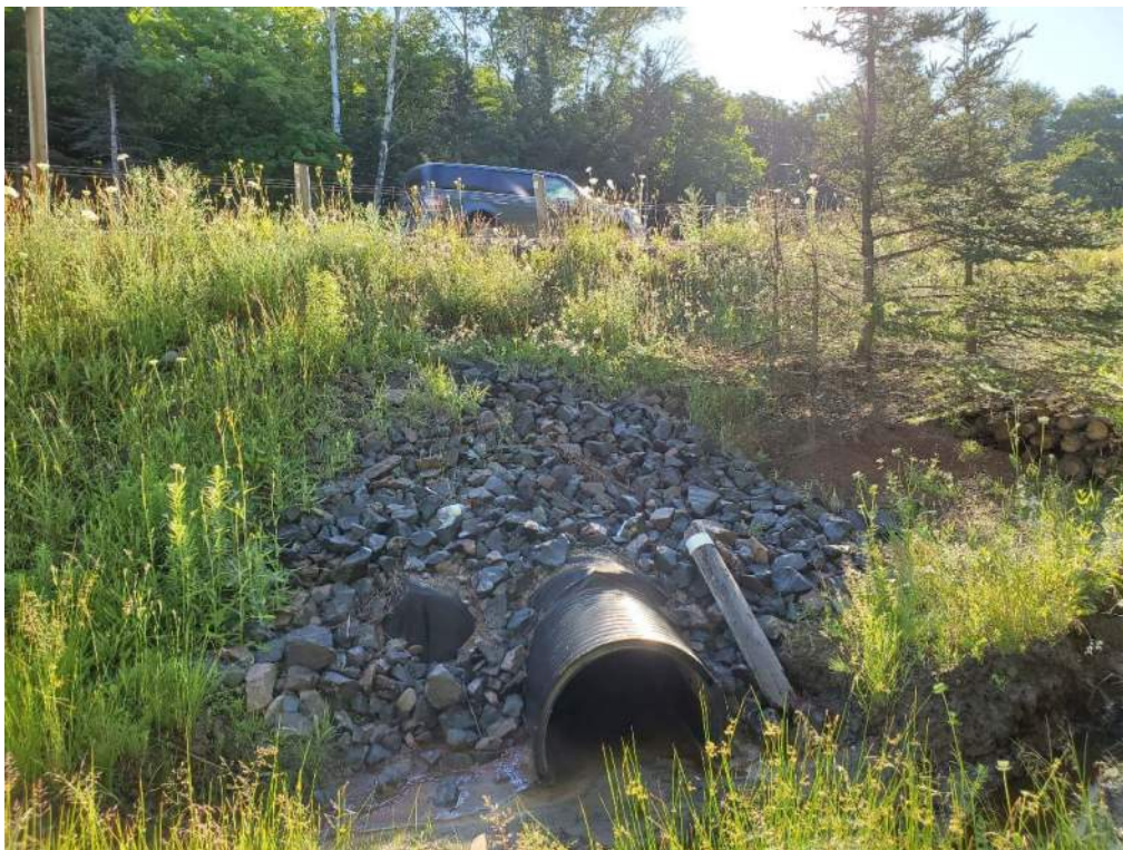
Photo 2: West end of culvert (outlet) liner, surrounded by rip rap embankment. Host pipe is not visible – looking east
