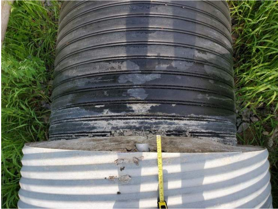
Photo 3 – Outlet looking down at grout protruding ~70mm
