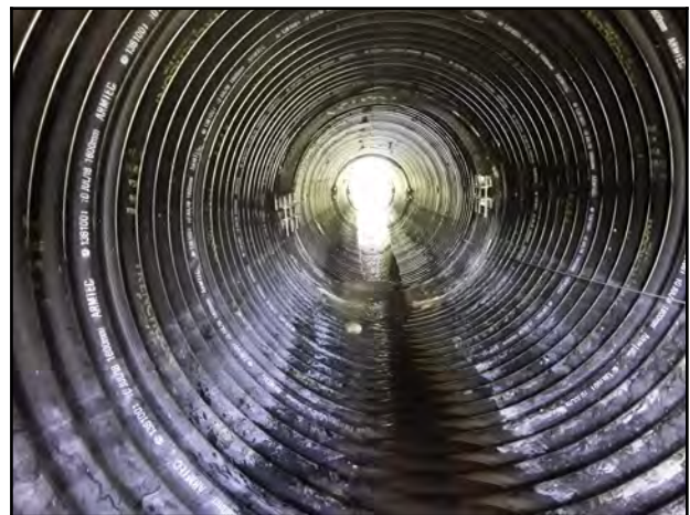
Photo 12 - Downstream pipe alignment and shape.
