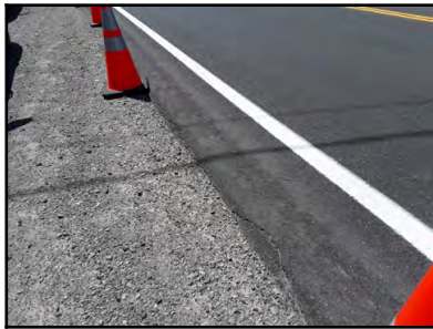
Photo 1 - Light progressive edge cracking on outlet side.
