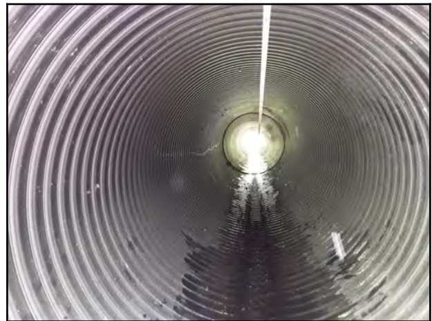
Photo 10 - Upstream pipe alignment and shape.
