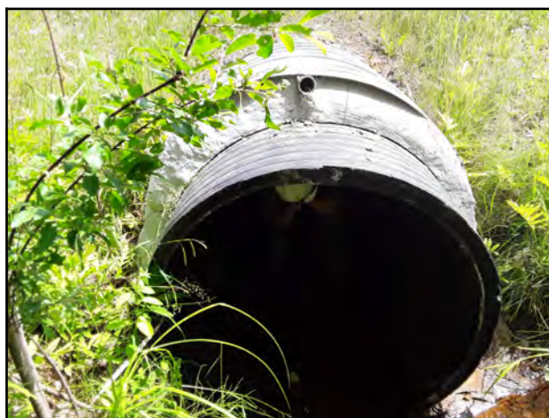
Photo 6 - Inlet overview.: Annular space of 80 mm between the existing CMP and the sliplined HDPE.
