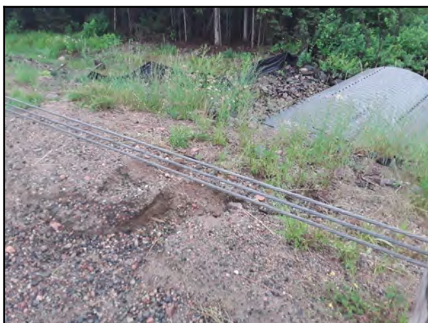
Photo 5 - Erosion channel on the outlet embankment measuring approximately 430 mm in width.
