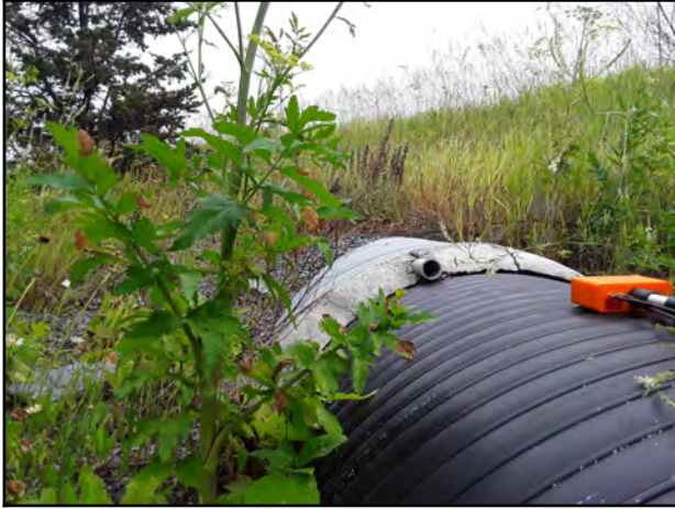
Photo 25 - Annular space of 120 mm between the existing CMP and the sliplined HDPE at inlet.
