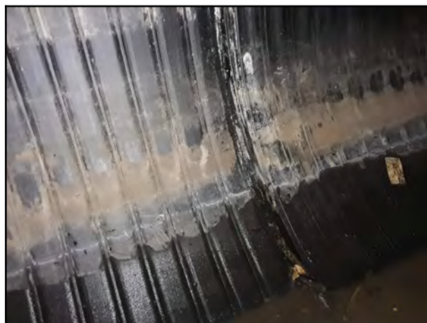
Photo 22 - V-4: Separated joint by approximately 40 mm with black caulking evident.
