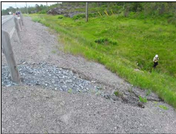
Photo 9 - Poorly repaired erosion channel on the inlet embankment.
