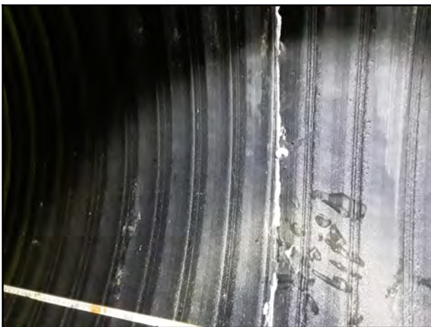
Photo 17 - V-3: Joint with visible silicone sealant.
