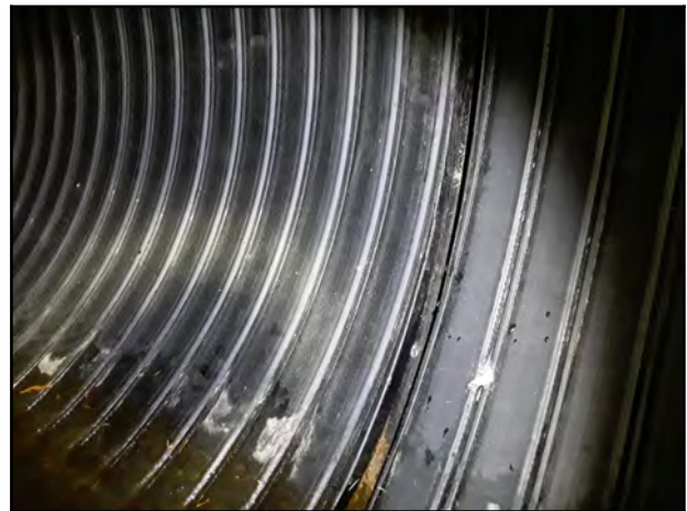
Photo 16 - V-3: Separated joint of approximately 30 mm with a visible coupler.
