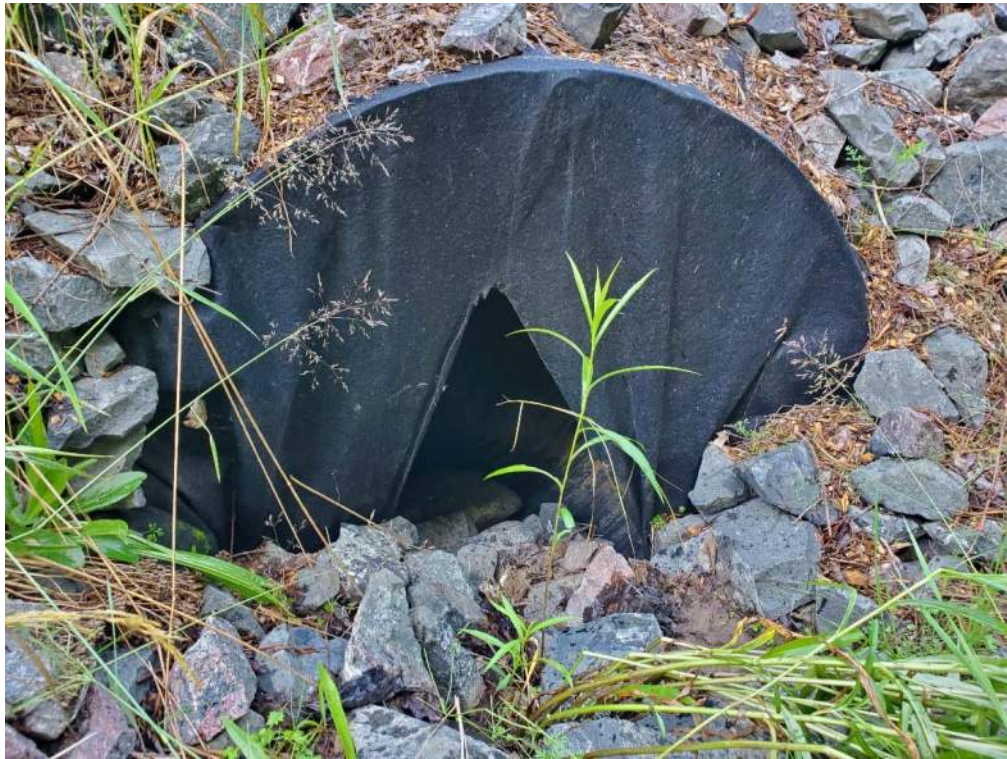
Photo 1: East end of culvert (inlet) covered with silt fence and surrounded by rip rap embankment. Grout is not visible. – looking west
