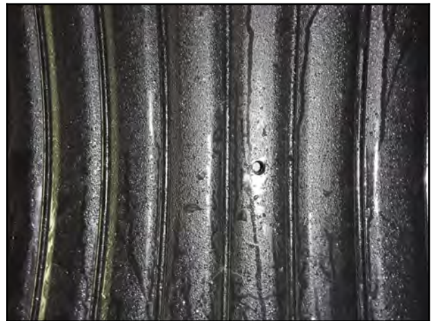
Photo 22 - 3.4 m at 8:30 with visible void.
