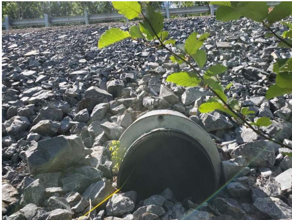
Photo 2: North end of culvert (outlet) surrounded by rock fill embankment. Cut off grout pipe noted– looking south
