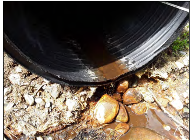
Photo 10 - Outlet is perched by approximately 260 mm in height.
