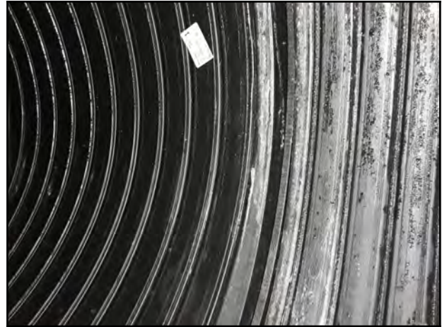
Photo 20 - V-4: Separated joint by approximately 40 mm.
