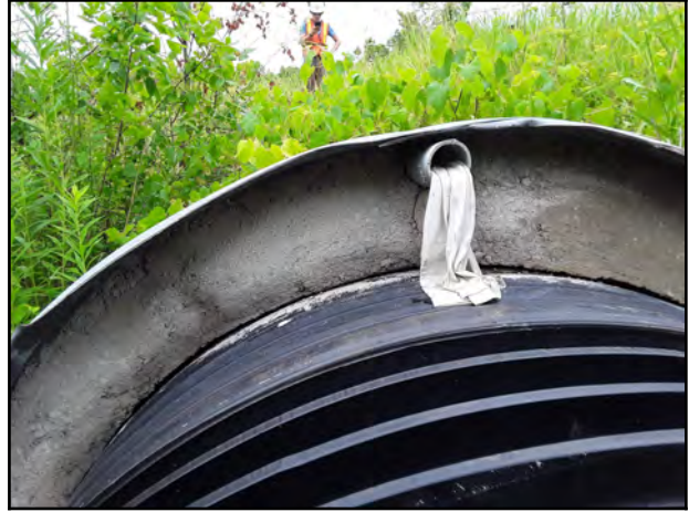
Photo 26 - Annular space of 200 mm between the existing CMP and the sliplined HDPE at outlet.
