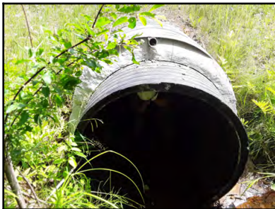
Photo 6 - Inlet overview.: Annular space of 80 mm between the existing CMP and the sliplined HDPE.
