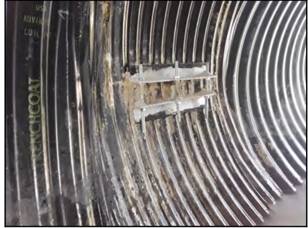
Photo 32 - V-8: Joint with visible expansion foam.
