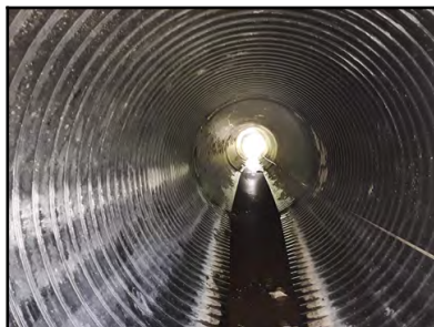
Photo 11 - Downstream pipe alignment and shape.
