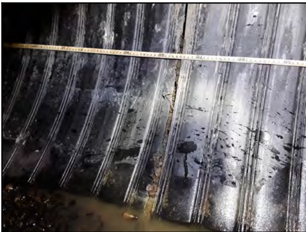
Photo 21 - V-4: Joint with visible expansion foam and visible supporting material.
