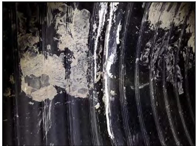
Photo 22 - V-4: Joint with visible expansion foam and visible supporting material.
