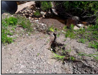
Photo 3 - Erosion channel on the outlet embankment measuring approximately 300 mm in width.
