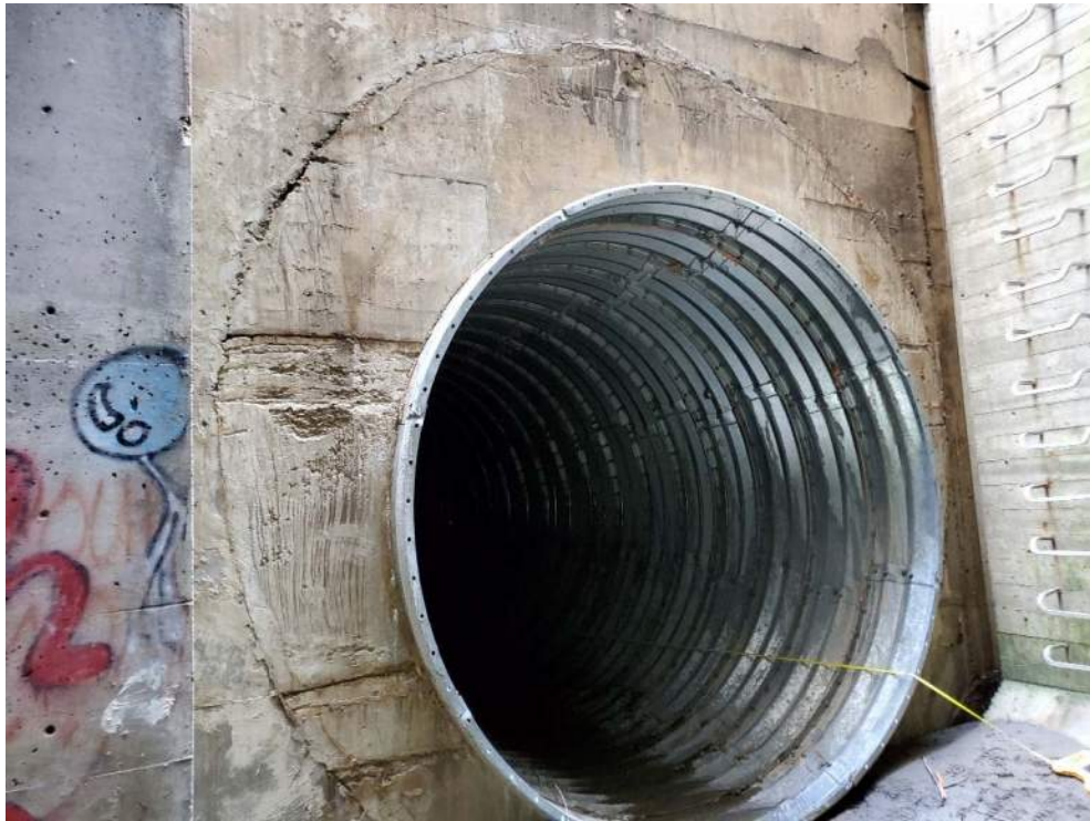
Photo 2: South end of culvert (outlet) beneath Highway 401 grouted in original concrete host pipe – looking north
