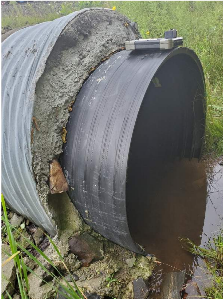
Photo 3: Cobbles paired with spray foam insulation utilized to fill voids at inlet in irregular grout finish
