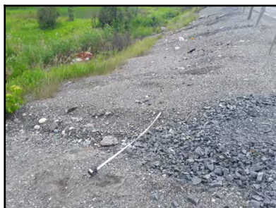
Photo 8 - Multiple erosion channels on the outlet, most severe measuring approximately 1500 mm in width.
