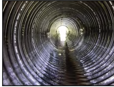
Photo 12 - Downstream pipe alignment and shape.
