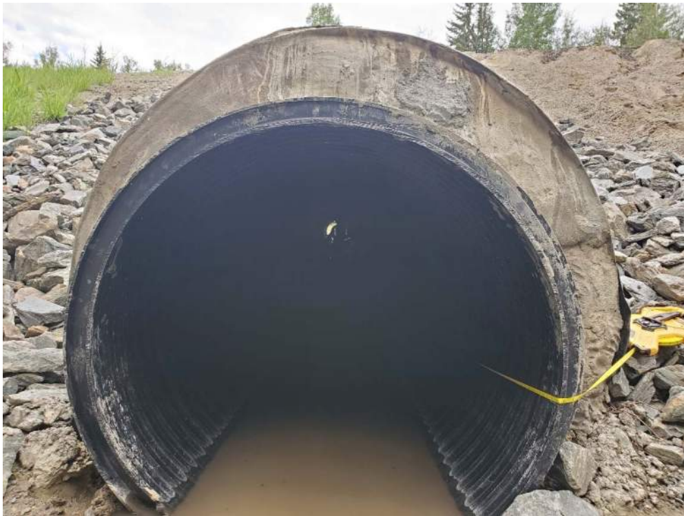
Photo 2: West end of culvert (inlet) not well centred in host pipe, surrounded by rip rap embankment – looking east
