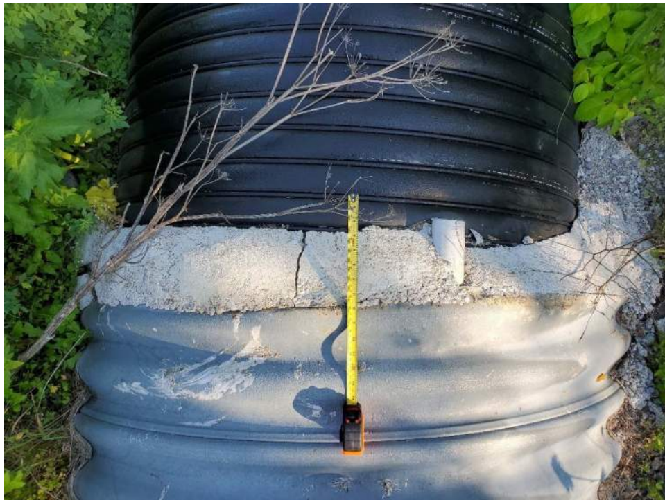
Photo 3 – Inlet looking down at grout protruding ~120mm
