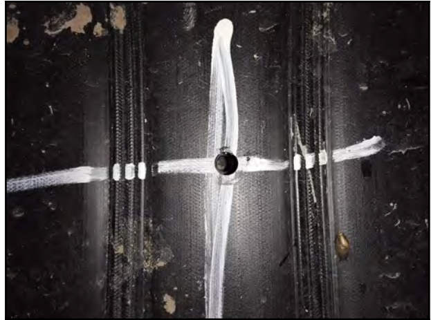
Photo 20 - V-3: Endoscope camera showing visible void.
