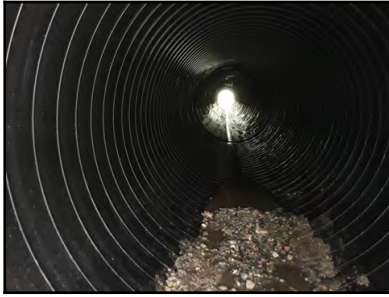
Photo 10 - Upstream pipe alignment and shape.
