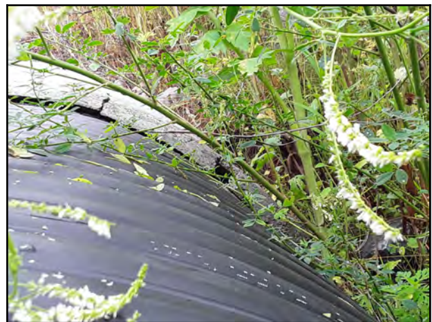
Photo 24 - Broken piece of grout at the inlet.
