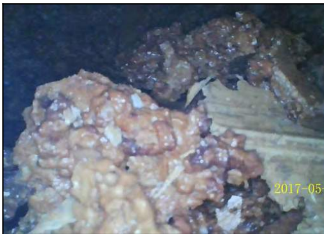
Photo 23 - V-5: Endoscope camera placed in the probe hole showing void.
