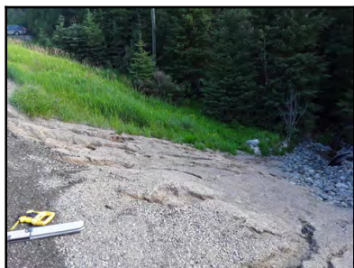
Photo 4 - Multiple erosion channels on the outlet embankment, most severe measuring approximately 800 mm in width.
