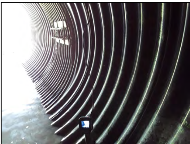
Photo 29 - V-7: Endoscope camera showing visible void.
