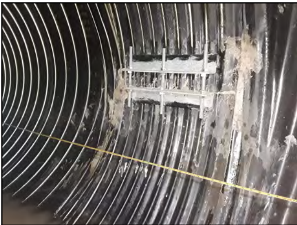
Photo 27 - V-6: Joint with visible expansion foam.
