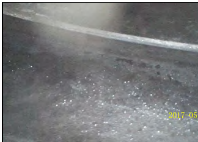
Photo 20 - V-3: Endoscope camera placed in the probe hole showing void.
