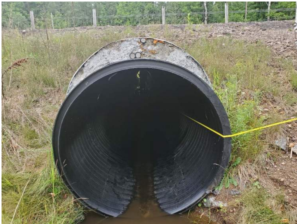
Photo 2: Outlet with minimal flow showing three (3) cut off grout pipes– looking west
