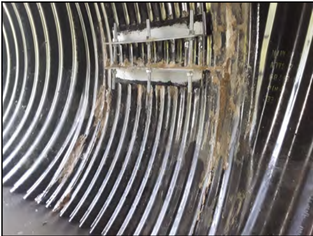
Photo 33 - V-8: Joint with visible expansion foam.
