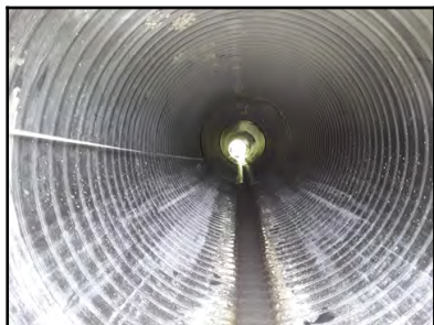
Photo 10 - Upstream pipe alignment and shape.
