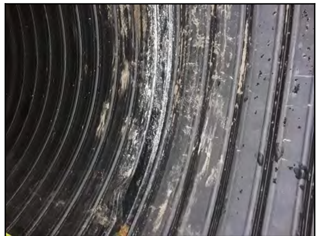
Photo 24 - V-6: Separated joint by approximately 40 mm with minor localized damage evident.
