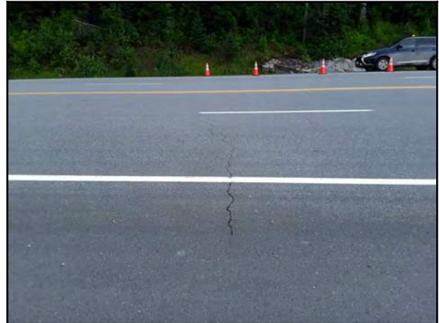
Photo 2 - Transverse crack.
