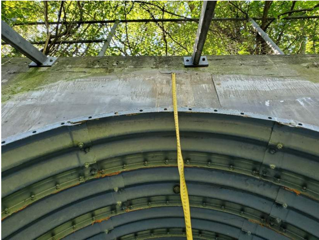
Photo 3: Crown grout infill approx. 0.53m at inlet– looking south
