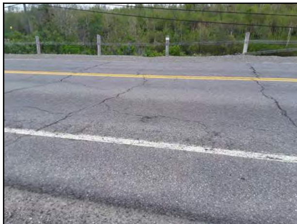
Photo 2 - Minor pothole measuring approximately 20 mm in-depth.
