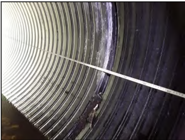
Photo 15 - V-2: Separated joint of approximately 70 mm with visible supporting grout material.
