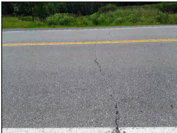
Photo 1 - Minor transverse crack present above the asset.
