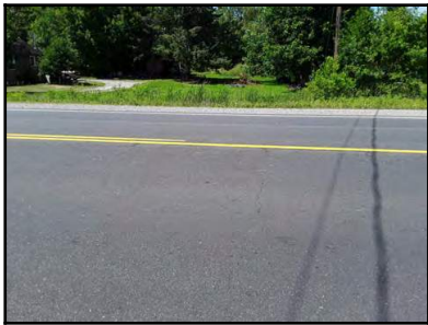
Photo 2 - Light transverse cracks.
