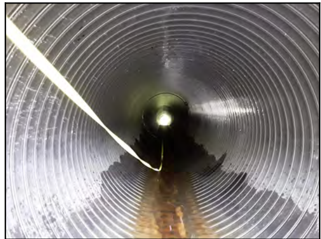
Photo 16 - Upstream pipe alignment and shape.
