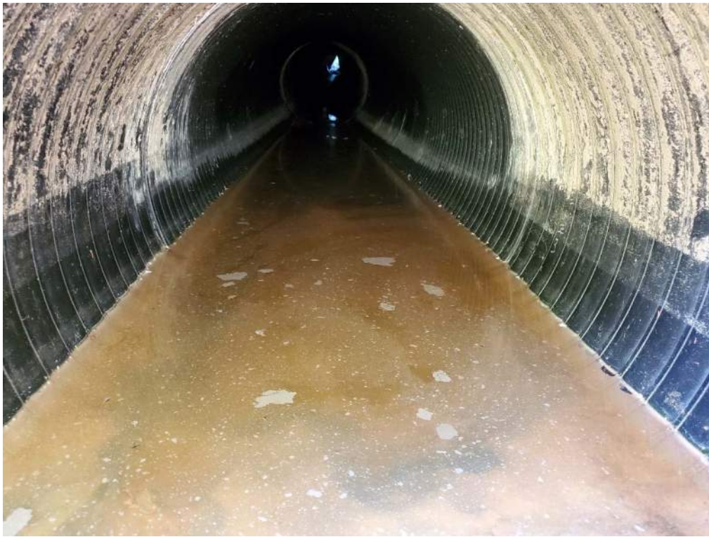
Photo 3: Standing water and basal sediments observed at outlet - looking east
