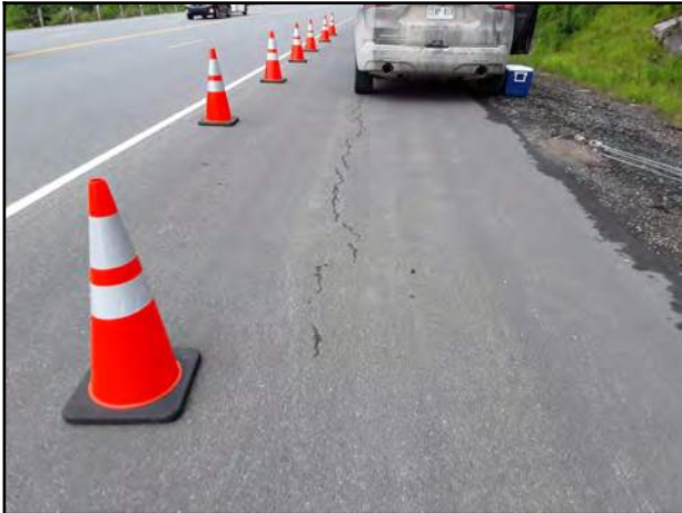
Photo 1 - Longitudinal crack.
