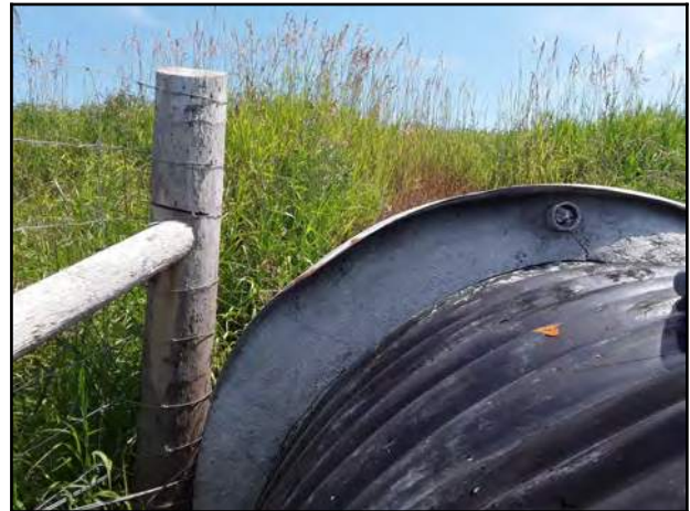
Photo 34 - Annular space of 240 mm between existing pipe and sliplined culvert at outlet.
