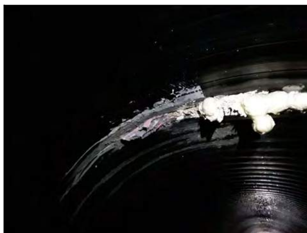
Photo 22 - V-5: Offset joint by approximately 40 mm with visible grouting and foam.
