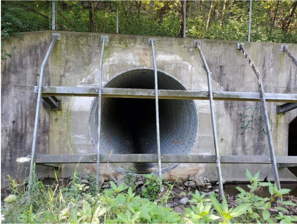
Photo 1: North end of culvert (inlet) grouted in original concrete host pipe – looking south
