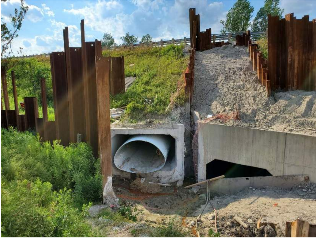
Photo 1: Liner installed but not yet grouted - active construction site – looking northwest at southern embankment
