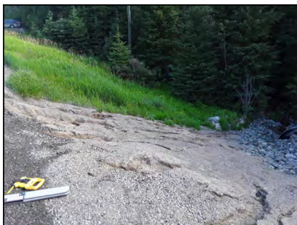
Photo 4 - Multiple erosion channels on the outlet embankment, most severe measuring approximately 800 mm in width.
