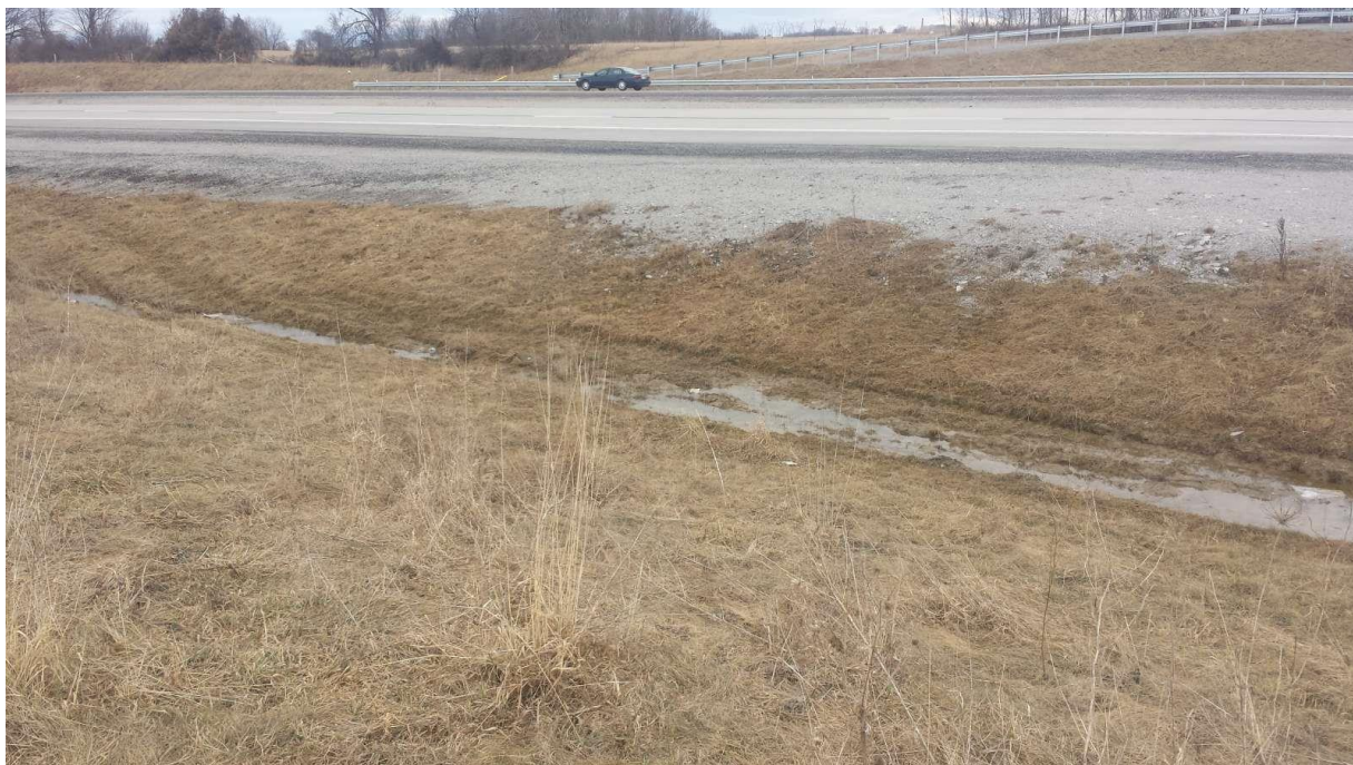
Plate 6: A view of the berm slope (bottom), stormwater drainage swale (centre) and Highway 404 (top), looking northeasterly. A small amount of water can be seen in the ditch on this day (April 10, 2015).
