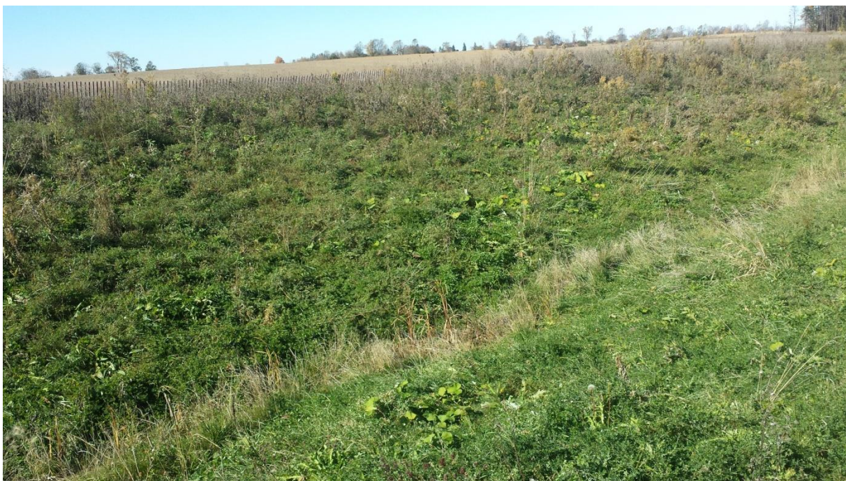
Plate 18: A view of the highway berm slope, looking northwest. No signs of seeps or erosion were evident on the berm (October 23, 2015).
