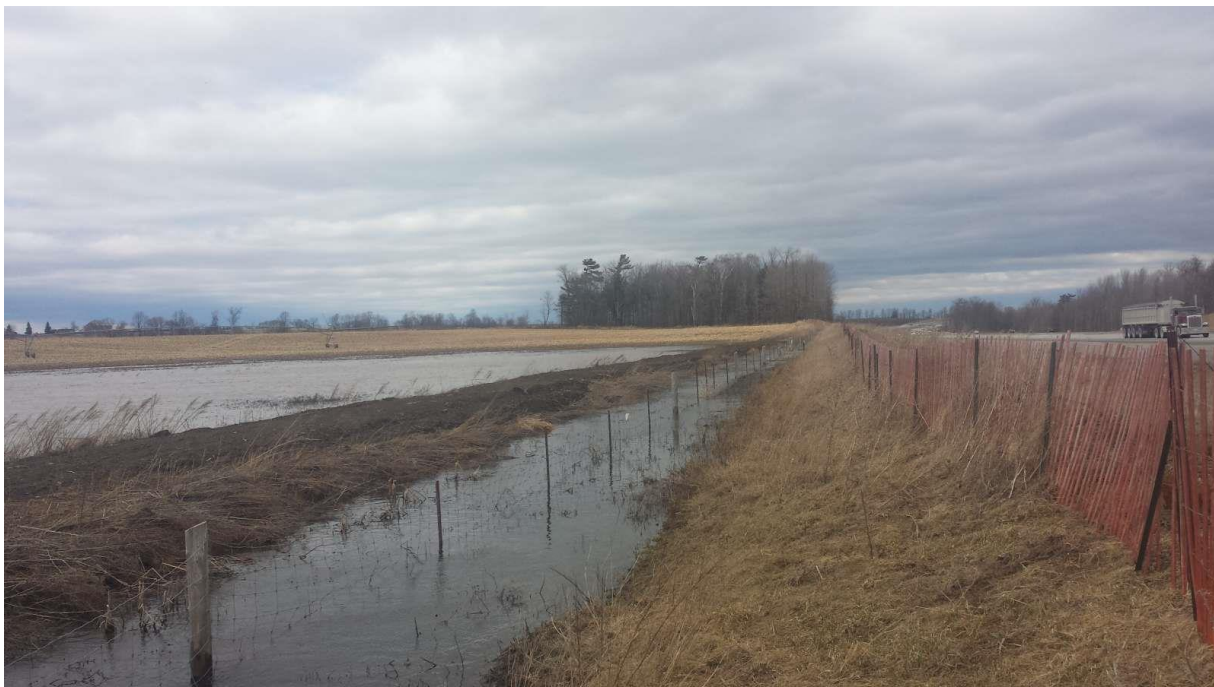
Plate 3: A view of the Site looking north from the berm. From left to right are the water ponded field, the berm on the Farm, the fenceline, and the berm in the highway Right-Of-Way (April 10, 2015).
