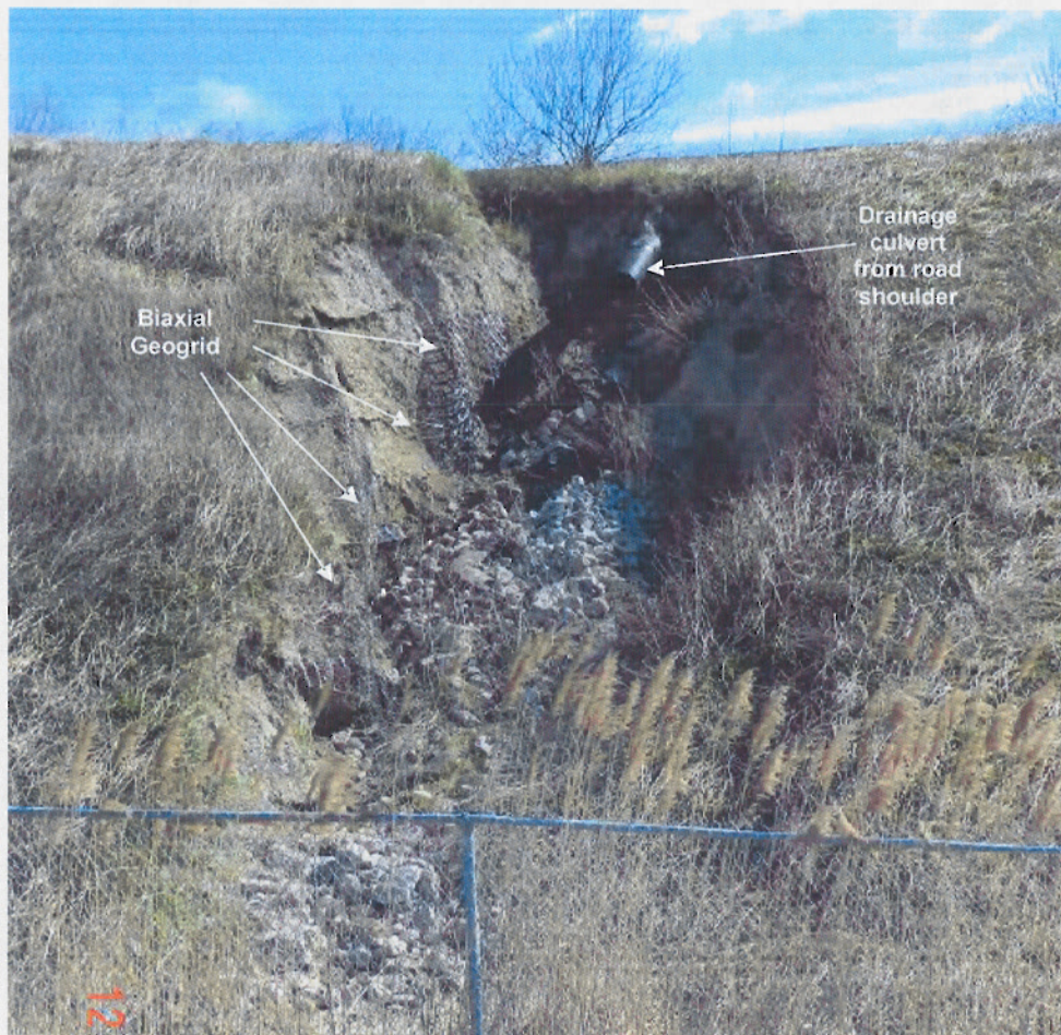
Figure 8: Photo of Slope Erosion Problem Area Number 3
