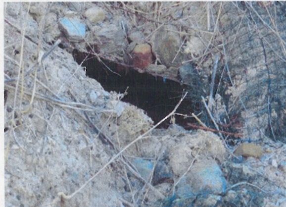
Figure 3: Close up of Slope Erosion Problem Area Number 1. Left, surface erosion; top, undermining and biaxial geogrid
