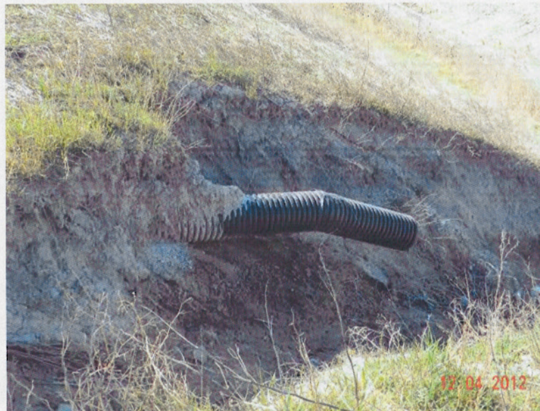
Figure 7: Material washed away around PVC pipe at the Problem Area Number 3
