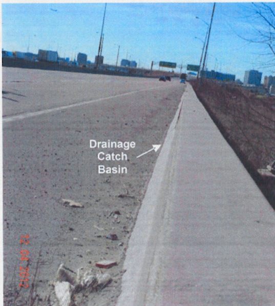
Figure 2: Drainage of HWY 427 Southbound. Left, road shoulder with watertight barrier, top, drainage catch basin
