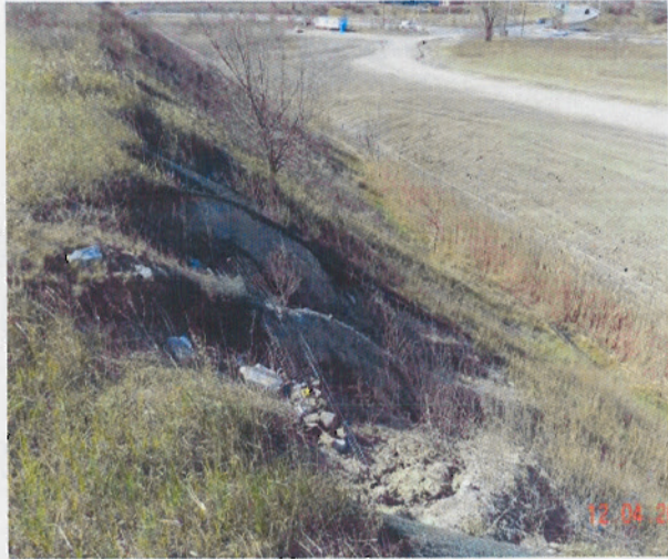
Figure 6: Close up of Slope Erosion Problem Area Number 2. Left, northern portion, 77m-86m south of the bridge; right, southern portion, 86m-110m south of bridge.
