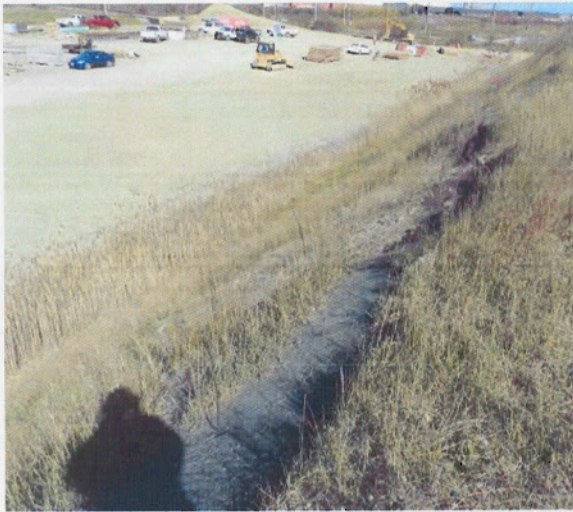
Figure 6: Close up of Slope Erosion Problem Area Number 2. Left, northern portion, 77m-86m south of the bridge; right, southern portion, 86m-110m south of bridge.
