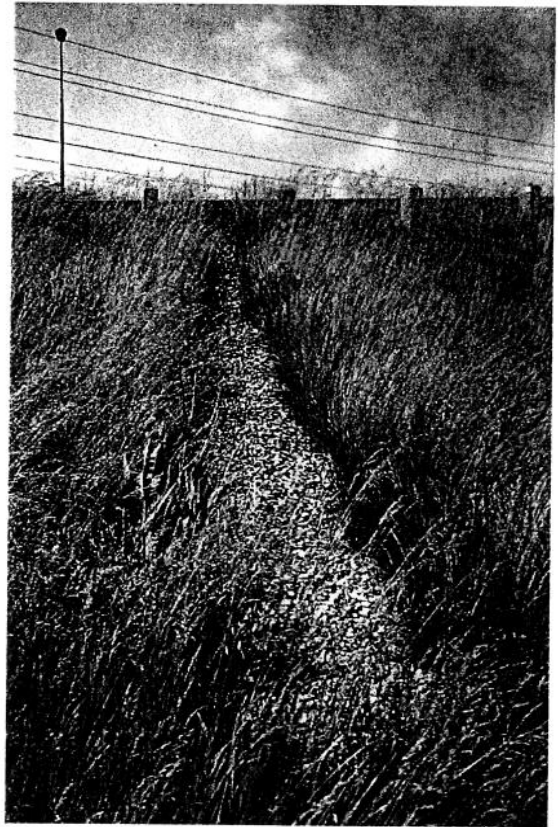
Slope Treatment consisting of crushed stone surrounding PVC drainage pipe.
