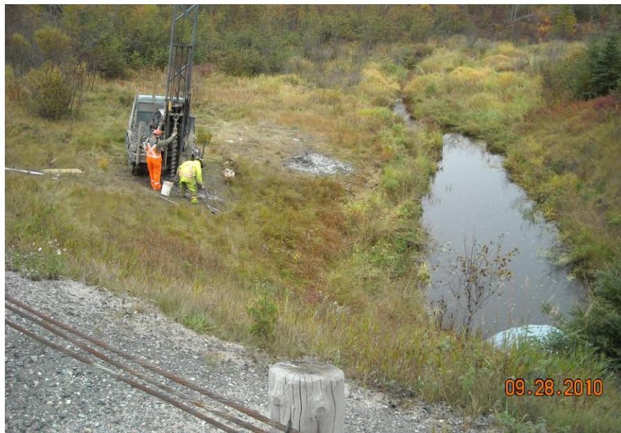
Drilling Boreholes for Culvert Extension – Looking East
