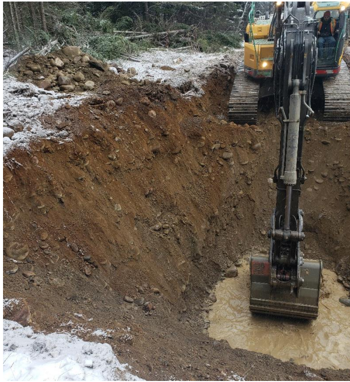
Photo 5. Excavating below water level, looking at west side wall (2018/11/29)
