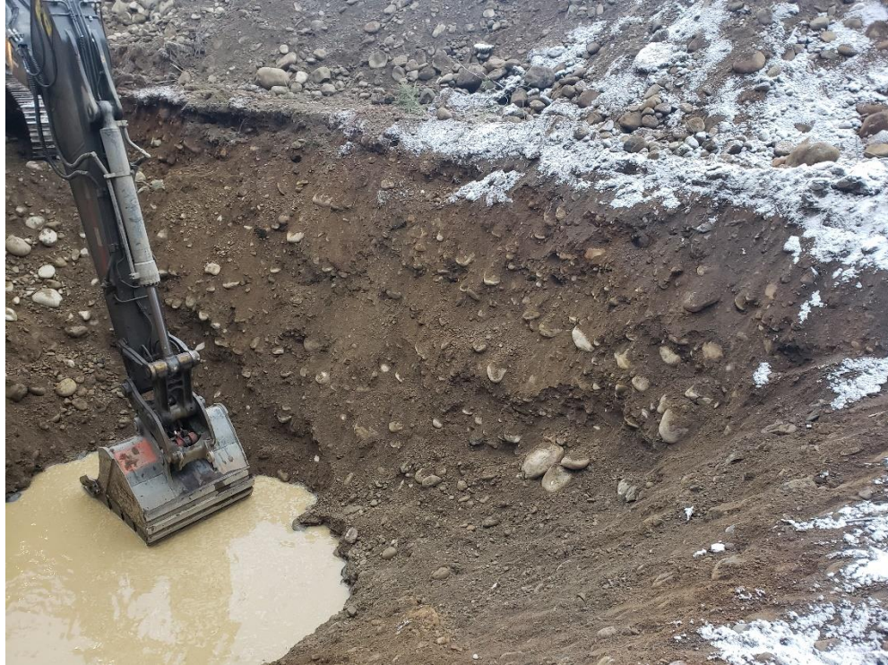
Photo 6. Excavating below water level, looking at east side wall (2018/11/29)
