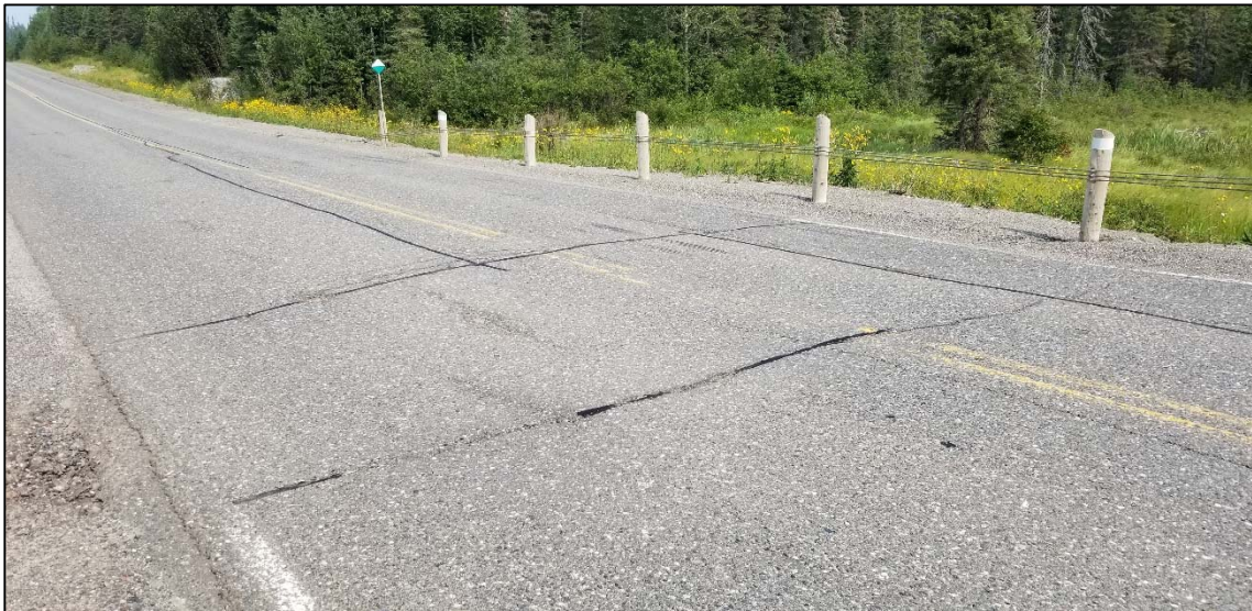
Photo 7. Transverse cracking near north culvert (2018/08/12)
