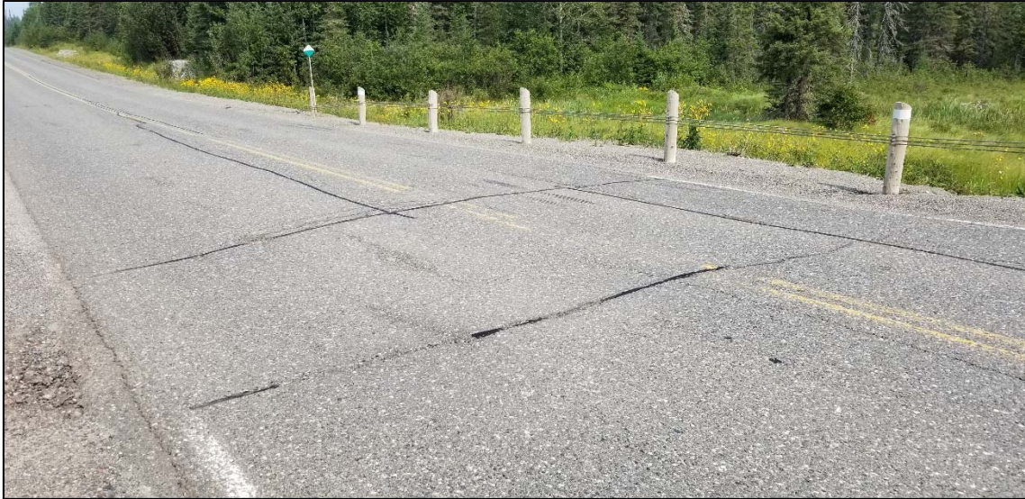
Photo 7. Transverse cracking near north culvert (2018/08/12)
