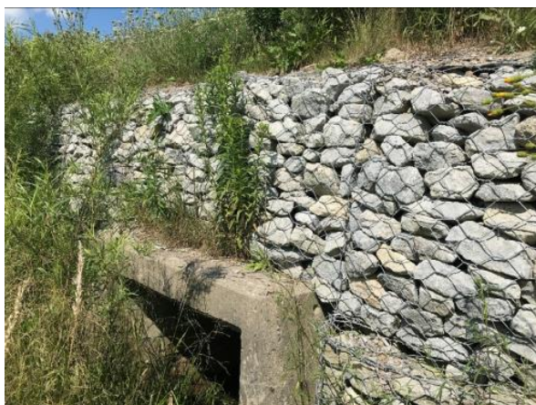
Photograph 1: Culvert inlet on west side of County Road 4 (August 2021, photograph courtesy of AECOM)
