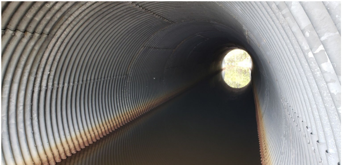
Photograph 2: Existing SPCSP Culvert (June 2020).
