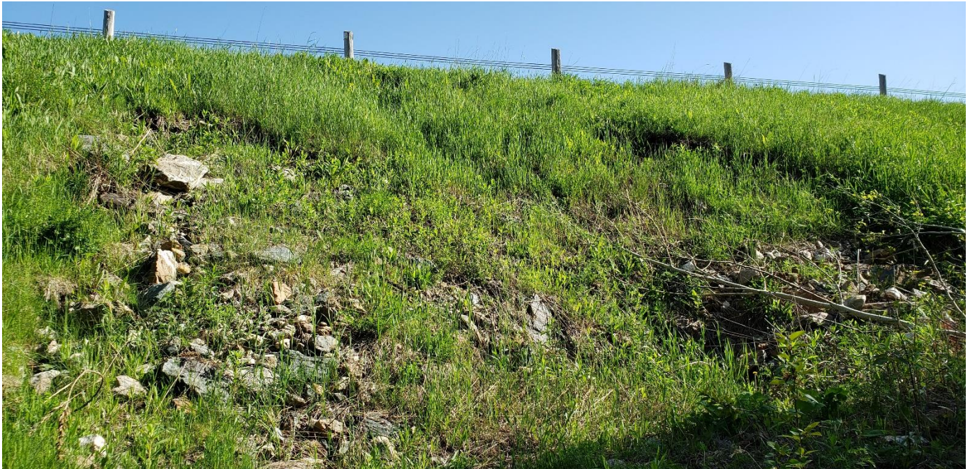
Photograph 3: South embankment, looking up the slope at previous slope failure and rehabilitated area (June 2020)
