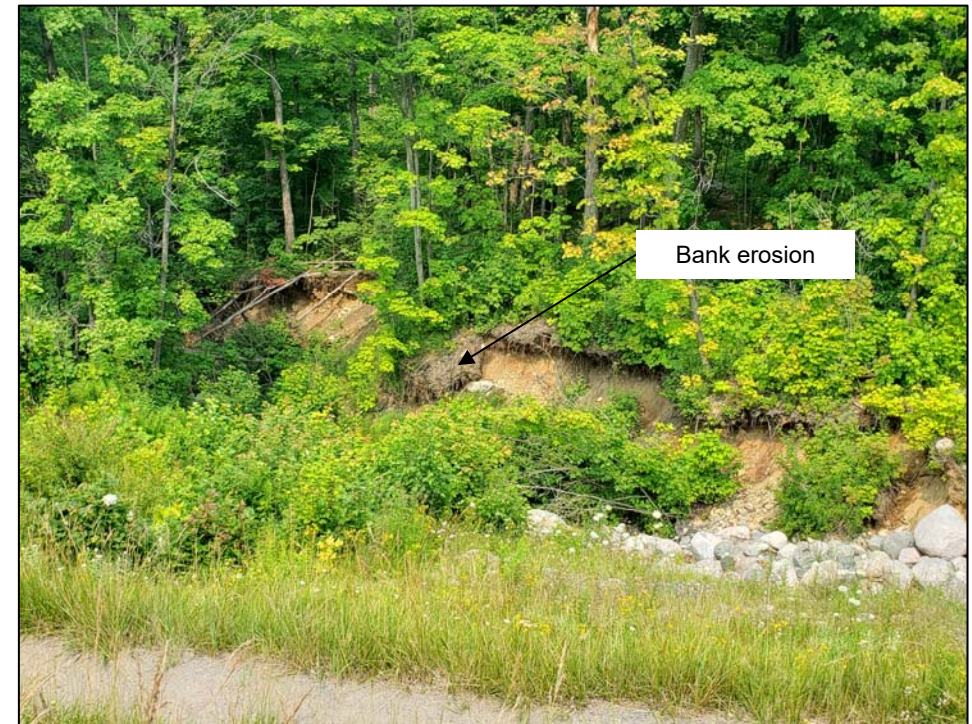
Photograph 2 (Watercourse channel at the toe of high fill area): Watercourse banks appear over steepened and eroding (looking east from Highway 17)
