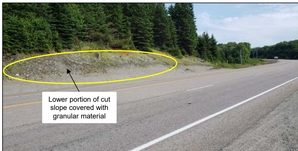
Photograph 2 (Southern segment of deep cut area): The lower portion of the cut slope is covered with granular material and the upper portion of the cut slope is heavily vegetated with coniferous trees (looking southeast from Highway 17)
