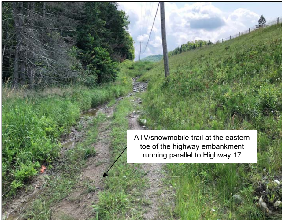
Photograph 3 (Borehole HF1-02 as-drilled location): The eastern slope of the highway embankment is vegetated with grasses and weeds; standing water and a marsh are visible near the toe of the slope (looking south, parallel to Highway 17)
