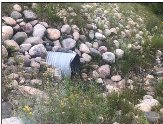
Photograph 3 (Outlet of CSP Culvert at STA 13+410 ): The slope of the highway embankment near the culvert outlet is covered with rip-rap (looking north and parallel to Highway 17)
