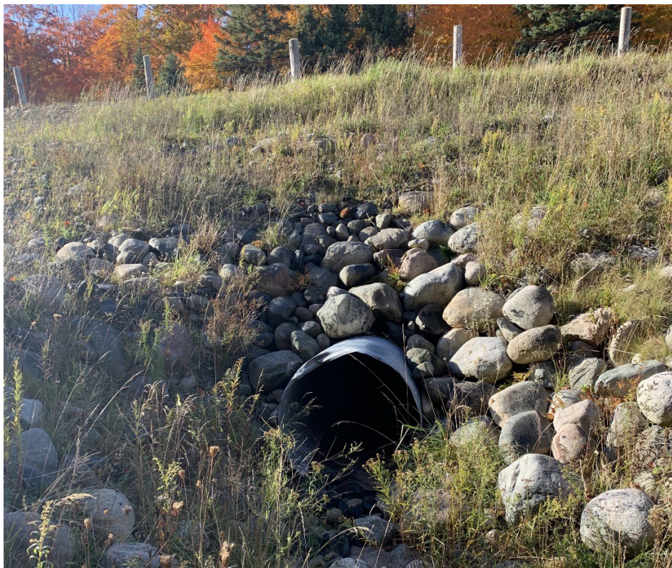
Photograph 1: Existing CSP culvert outlet (October 2022)
