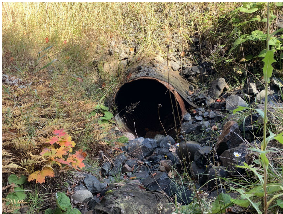
Photograph 2: Existing CSP culvert inlet (October 2022)
