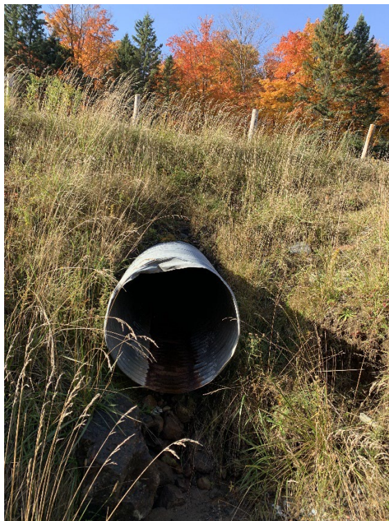
Photograph 1: Existing CSP culvert outlet (October 2022)
