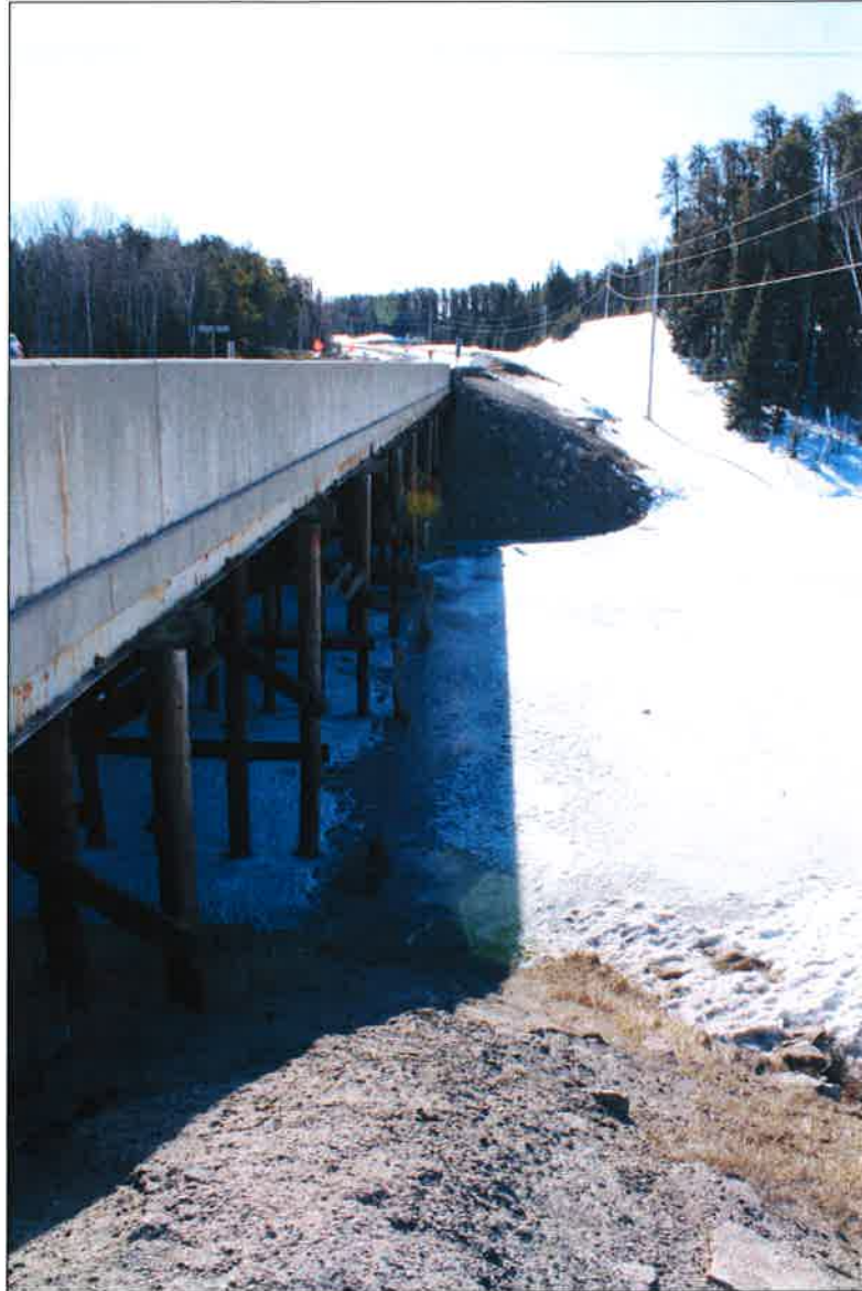
Photograph 3 – Gulliver River Bridge, existing foundation elements
