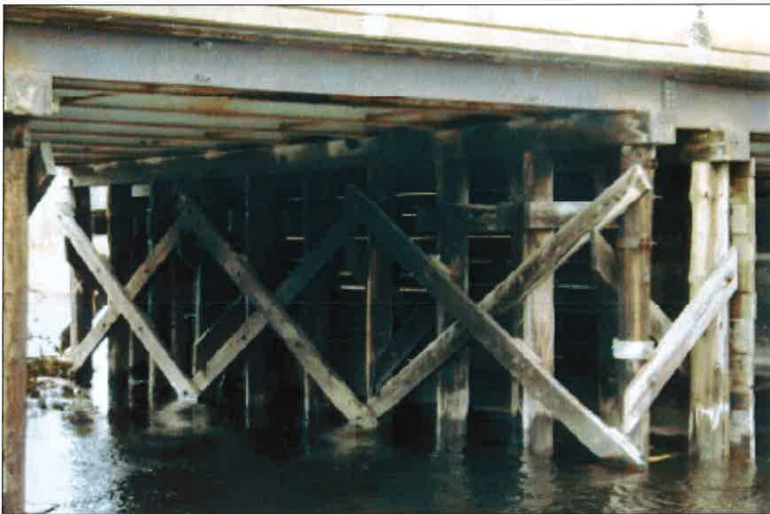
Photographs 5 and 6– Blackwater River bridge, existing piers
