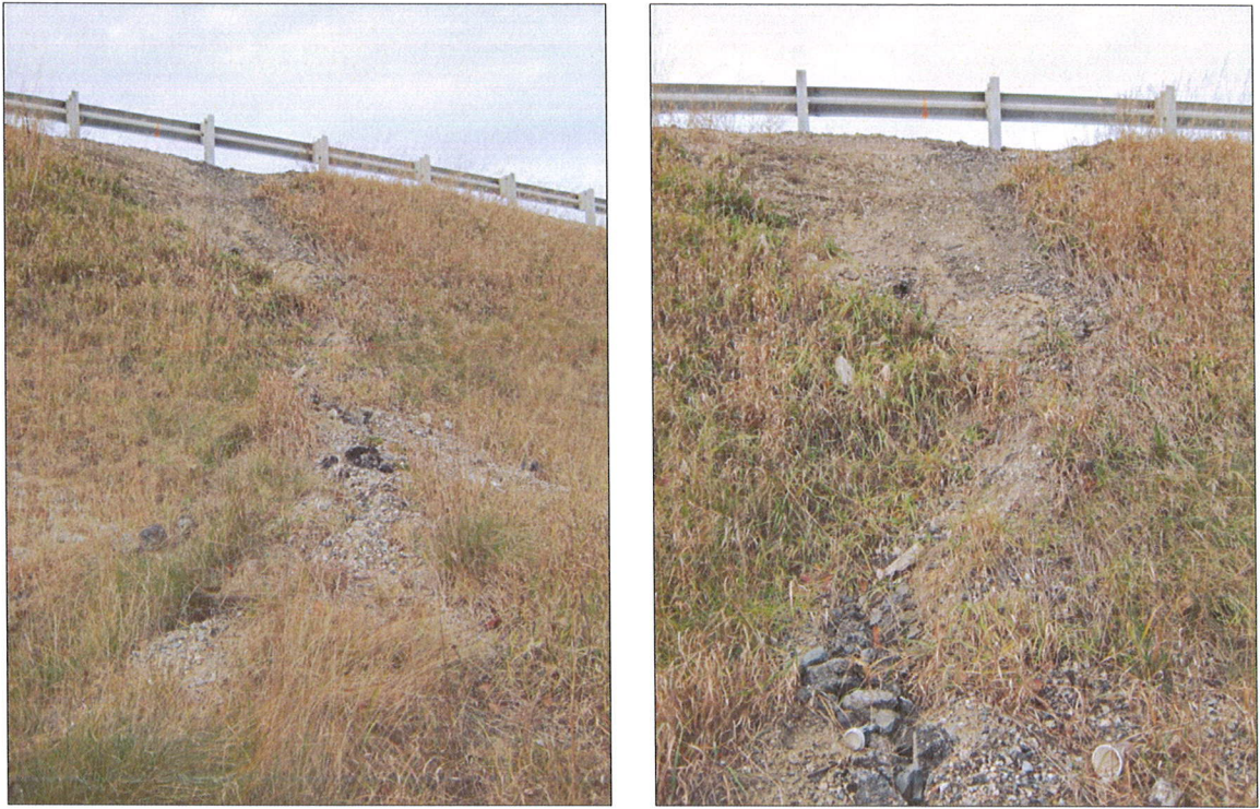
Photograph 3 – Surficial erosion on the southeast embankment
