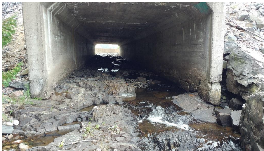
Photograph 4: West End (Outlet) and Exposed Bedrock at Invert (August 2018)
