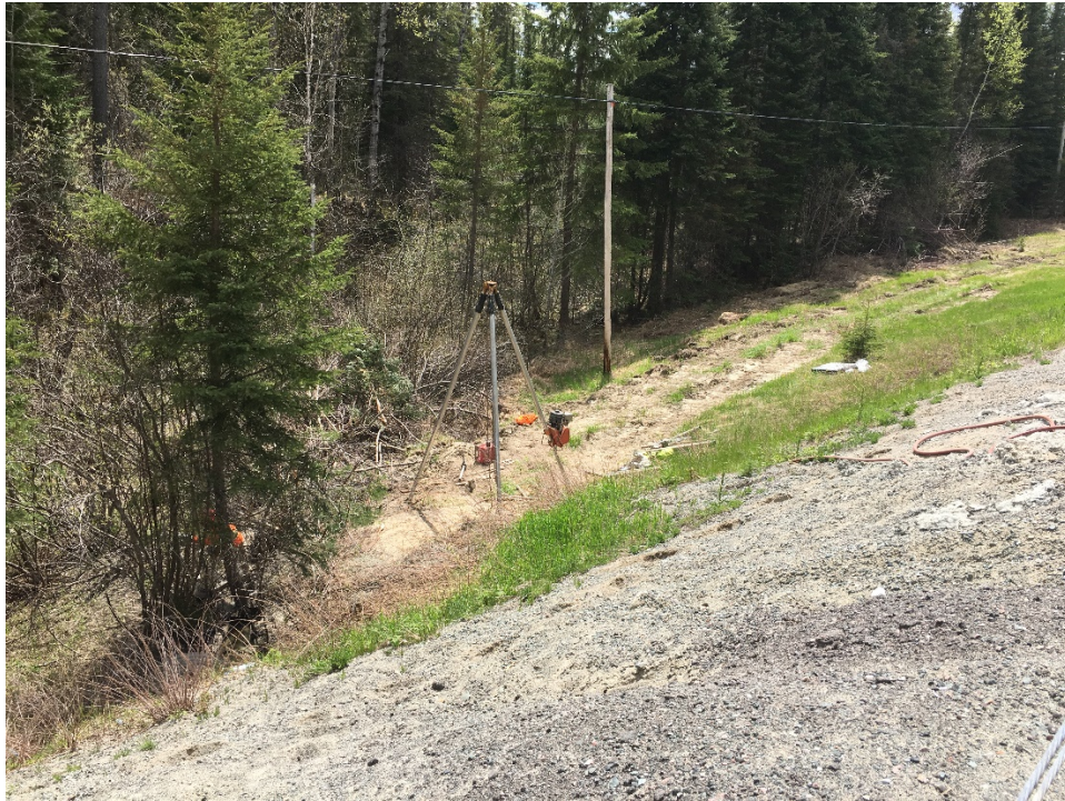
Photograph 3: Portable Drilling Rig Positioned at Borehole C263-5 near Culvert Outlet (June 2019)
