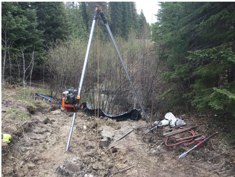
Photograph 4: Portable Drilling Rig Positioned at Borehole C263-4 near Culvert Inlet (June 2019)
