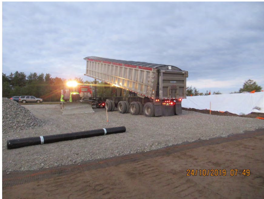
Photograph 1: Unloading of 50 mm CRL for Granular Pad
