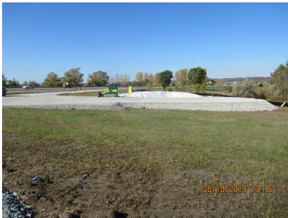
Photograph 6: Completed Granular Pad.
