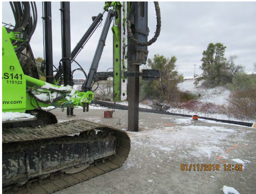
Photograph 5: Pile Driving of First Pile Segment (18 m length)
