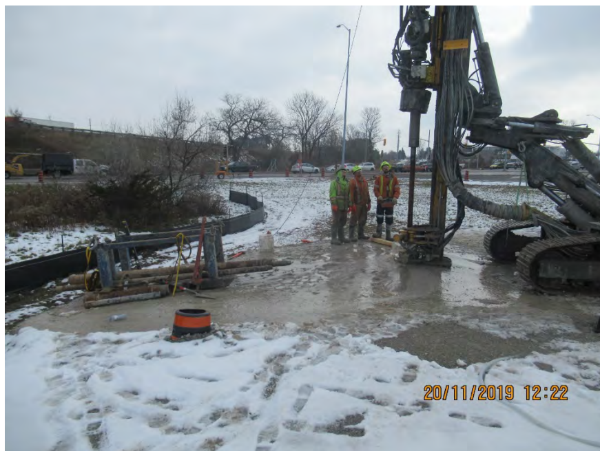
Photograph 2: Casing Installation for Micropiles
