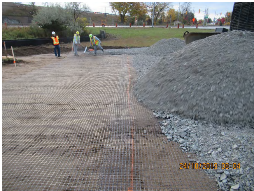
Photograph 2: Installing Geo-Grid with 30 cm Overlap
