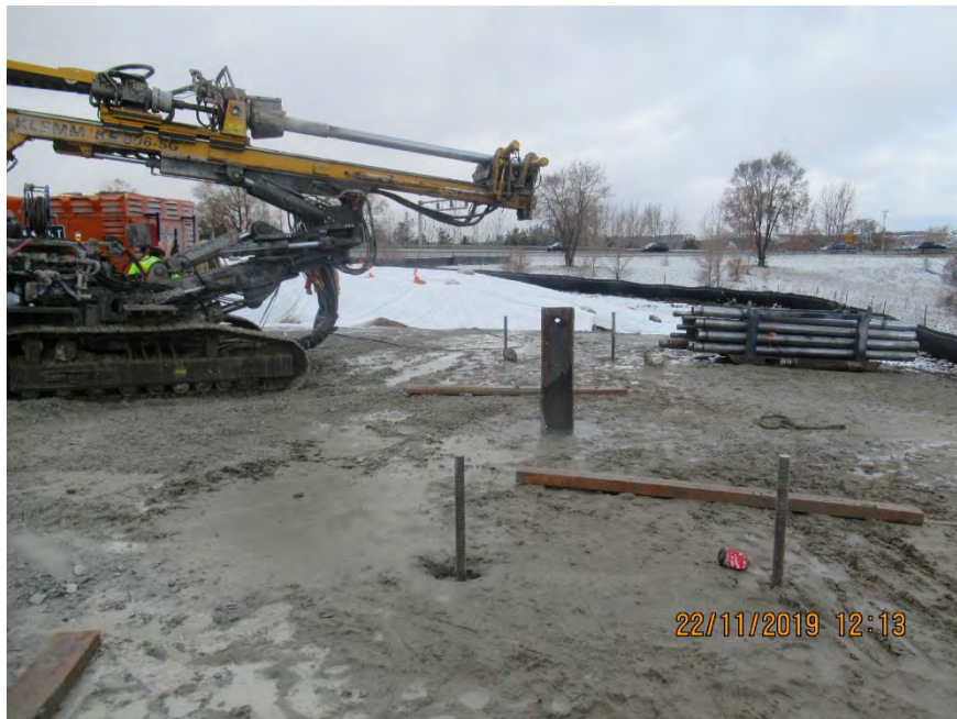
Photograph 8: Test Pile TP-1 and Micropiles MP-1A, MP-1B at bottom left to right and Micropiles MP-2A and MP-2B at top left to right
