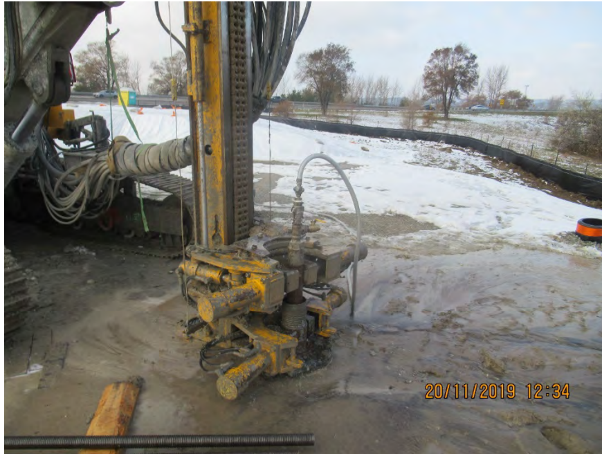
Photograph 3: Grout Injection at Micropile MP-1A
