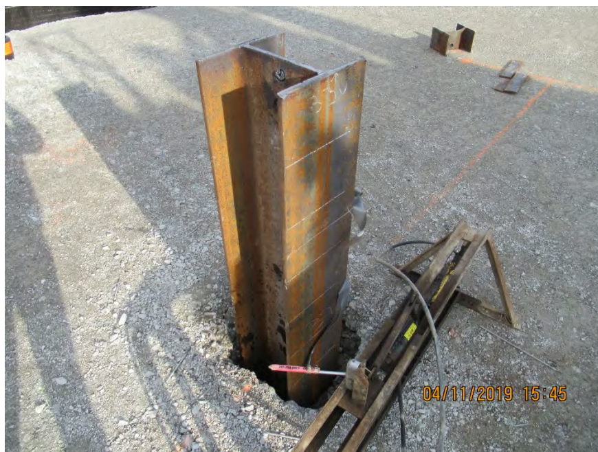
Photograph 9: Final driven Elevation of Pile to 31.8 m
