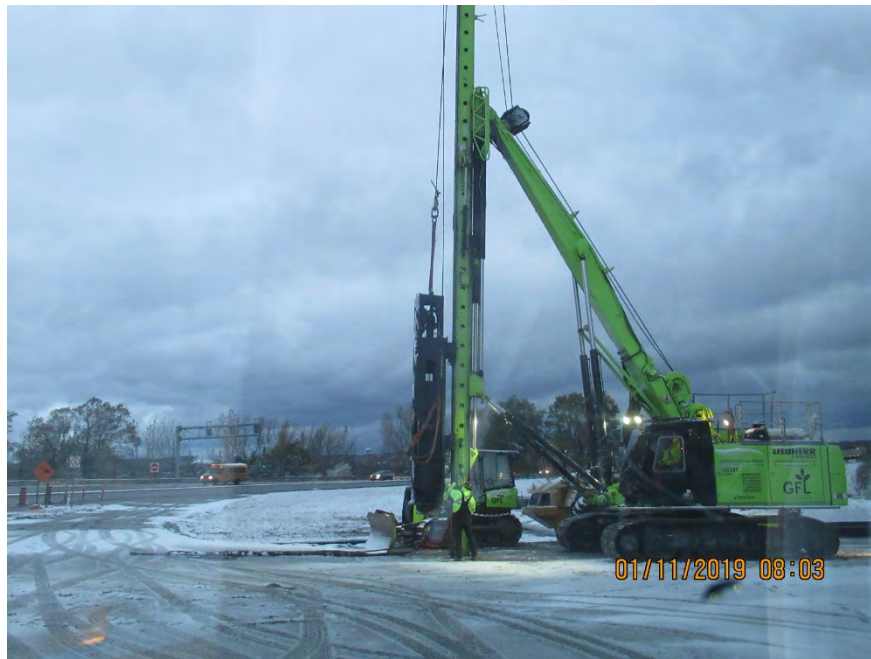
Photograph 1: Installing H-40/7 Hydraulic Hammer
