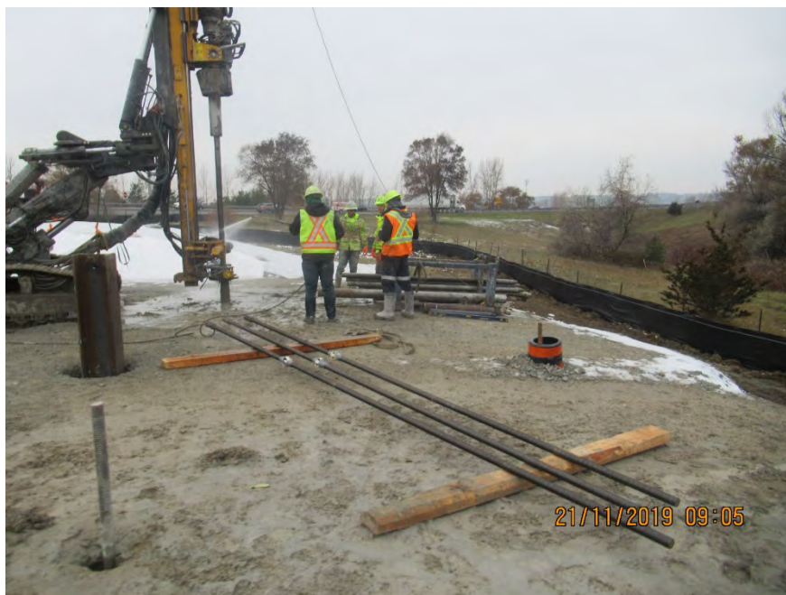
Photograph 4: Anchor rods prepared for installation of Micropile MP-2A
