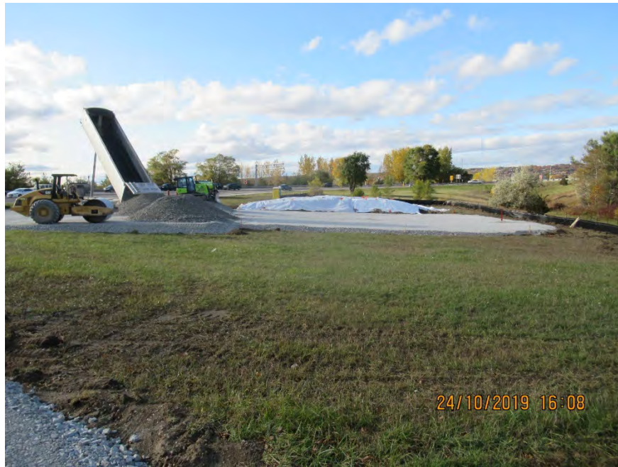
Photograph 5: Granular Pad under construction.
