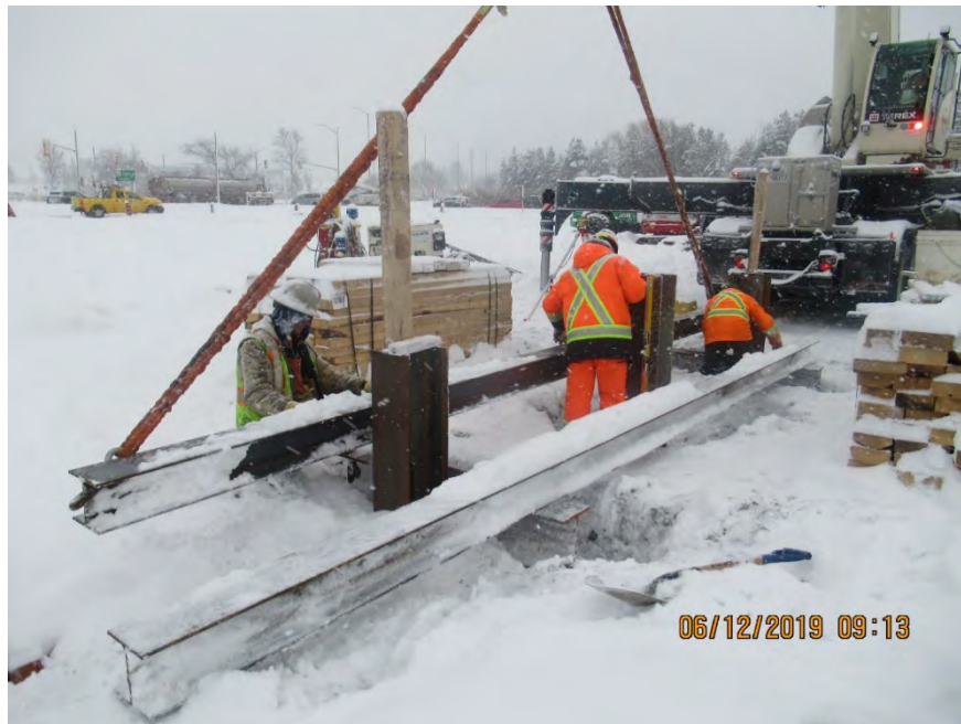
Photograph 11: Reaction Frame Assembled
