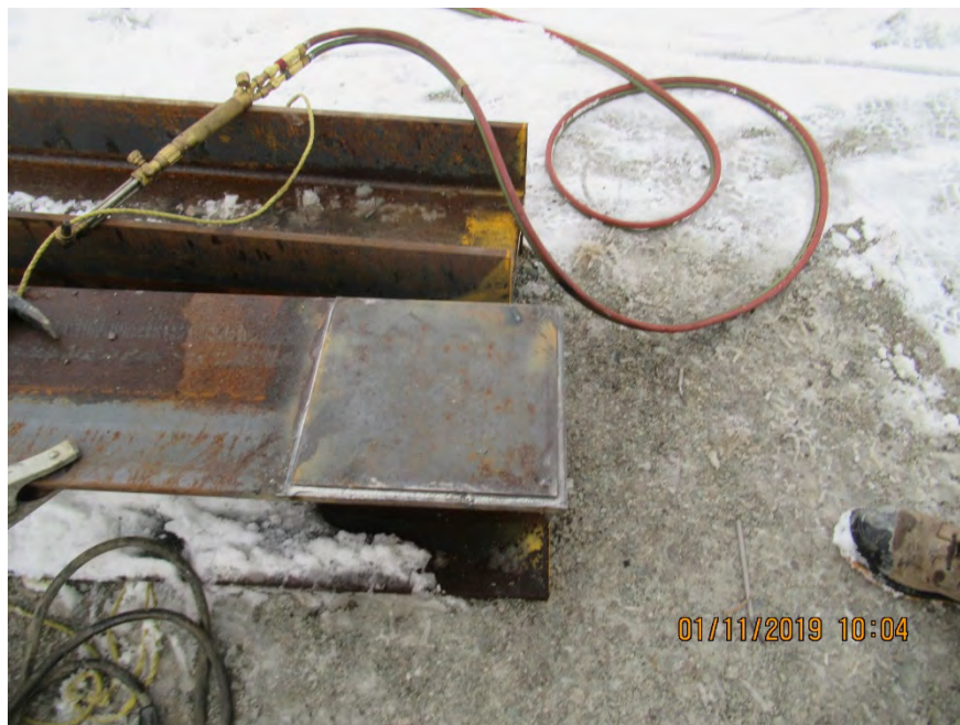
Photograph 2: One of the Two Pile Driving “Shoes”
