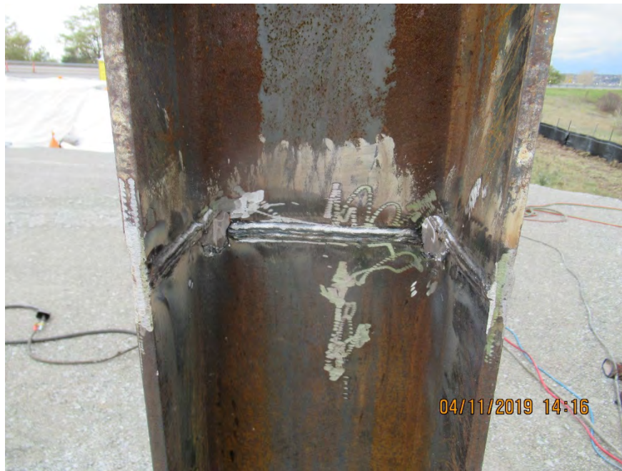
Photograph 7: Welding of Pile Segment 1 and Pile Segment 2
