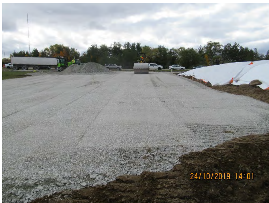
Photograph 4: Compaction of first lift of 50 mm CRL (30 cm lift)
