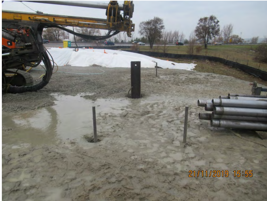
Photograph 7: Test pile TP-1 and Micropiles MP-1A, MP-1B and MP-2A
