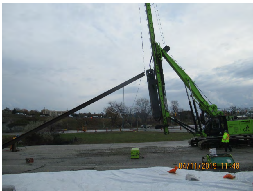
Photograph 6: Lifting of Second Pile Segment (18 m length)
