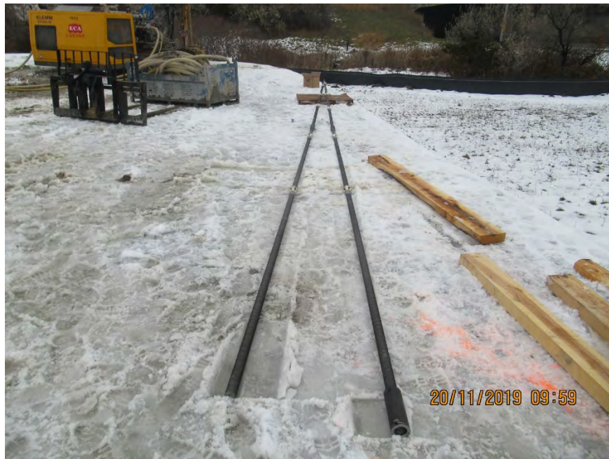
Photograph 1: Micropile Rods Prepared for Installation
