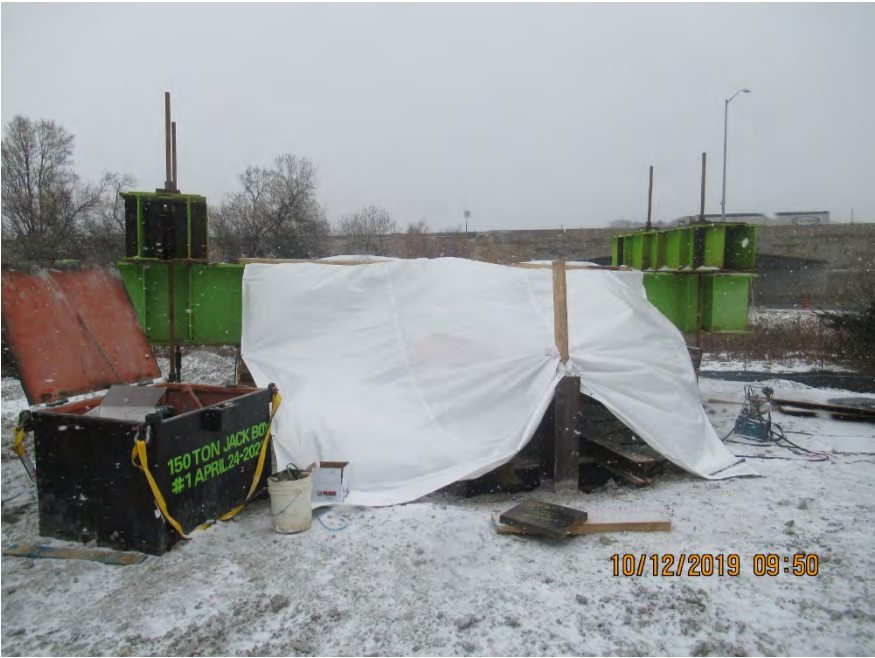
Photograph 13: Reaction Frame Setup with Tent
