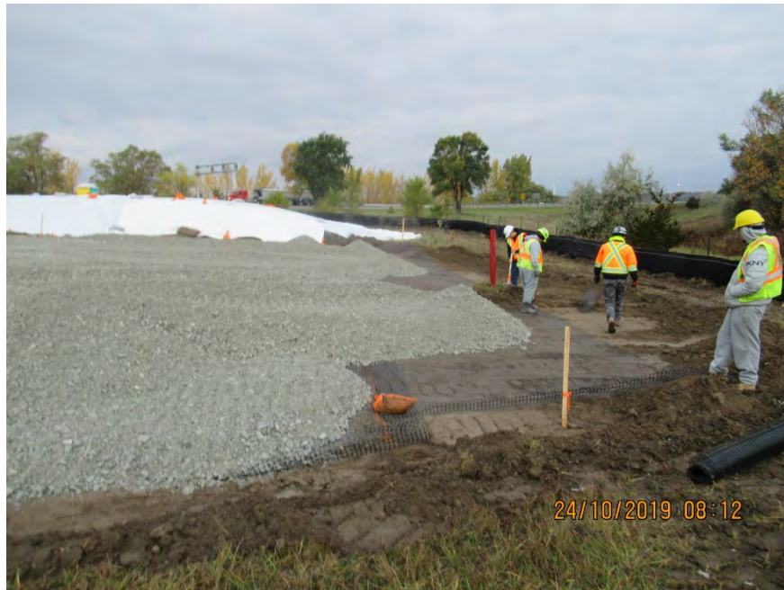
Photograph 3: Installing Geo-Grid and Placing 50 mm CRL
