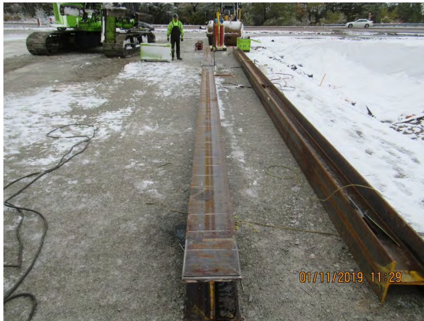
Photograph 3: Interval Markings (20 cm) on H-Pile Lengths
