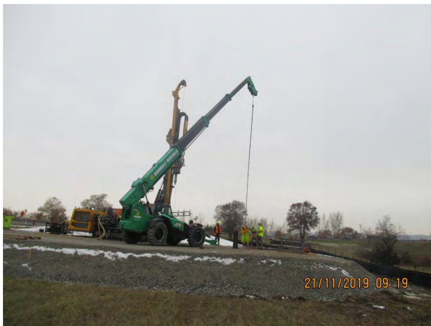
Photograph 6: Installation of Anchor Rod for Micropile MP-2A
