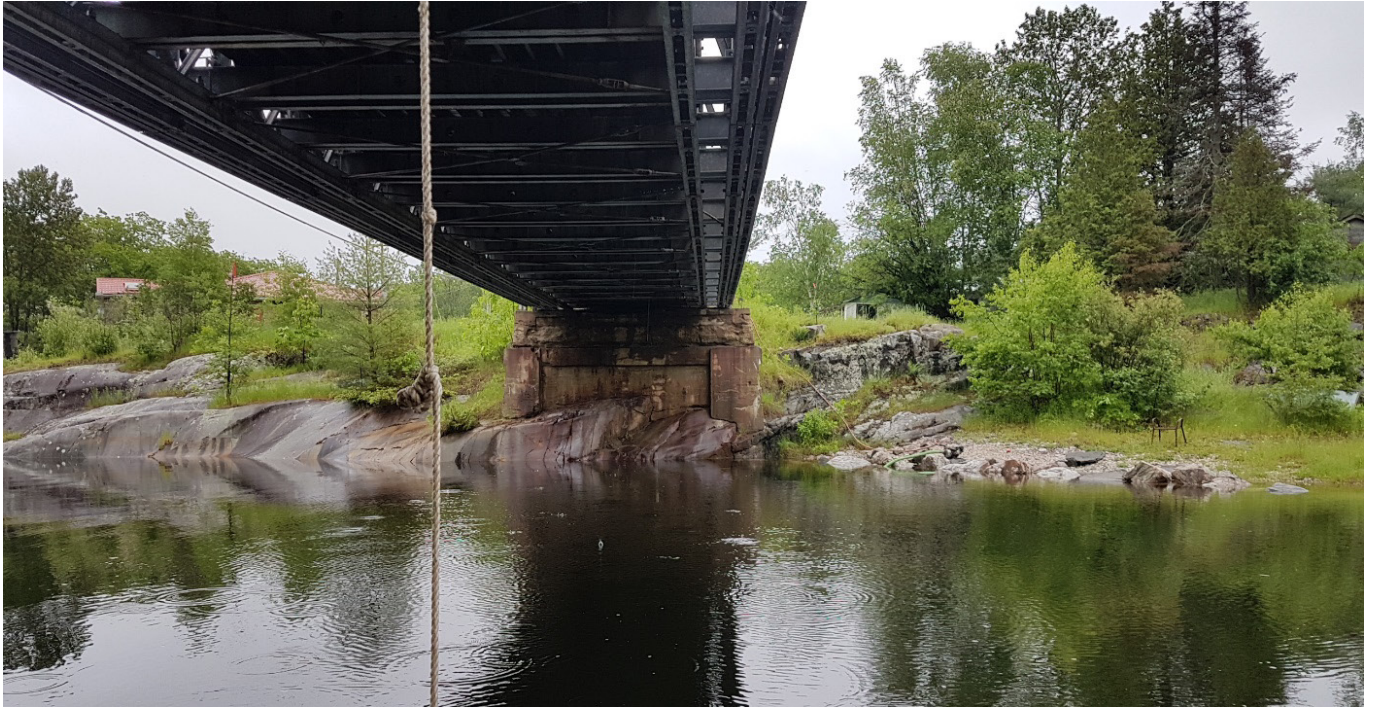
Photograph 5: South Abutment on Exposed Bedrock –North Side of Bridge Facing South (June 2019)
