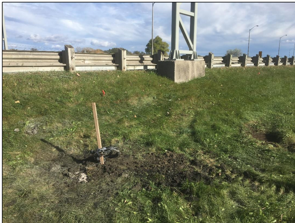
Photo 2. Borehole 17-01 upon completion of vibrating wire installation (2017-10-26).
