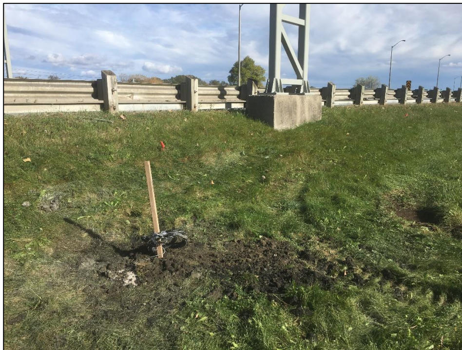
Photo 2. Borehole 17-01 upon completion of vibrating wire installation (2017-10-26).
